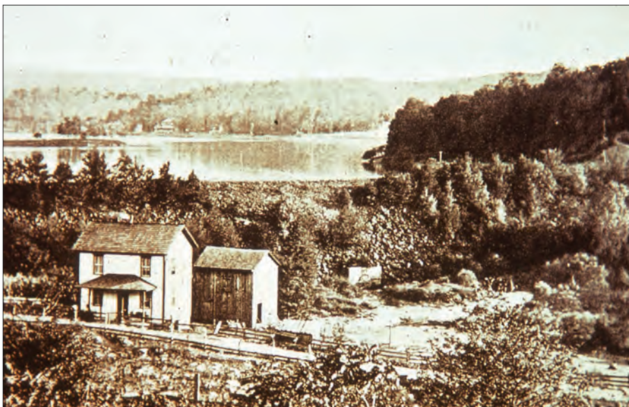
Figure 1.51. This farmhouse, which was likely owned by Joseph Lecky (Leahey), was located on the downstream side of side on the northeast corner of the dam, down the hill from Lake View Farm. The area of the dam repaired by the South Fork Fishing and Hunting Club is characterized by rip wrapped stones. (Johnstown Flood National Memorial Archives)
