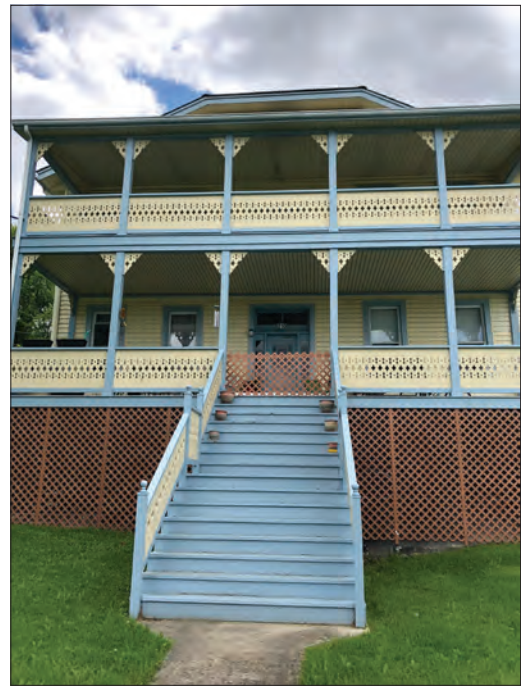
Figure 2.13. A view of northeast facade of the Double Cottage, 2018. (Olmsted Center for Landscape Preservation).
