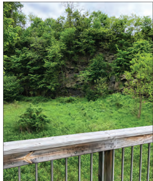
Figure 3.15. Woody vegetation grows from the embankments surrounding the former spillway, 2018, (Olmsted Center for Landscape Preservation).
