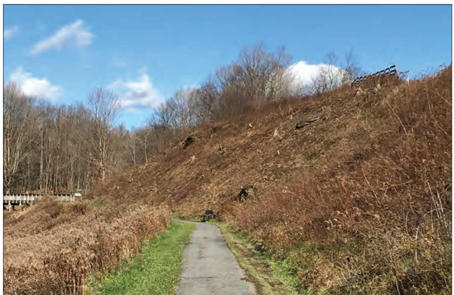
Figure 5.9. The slope east of the north abutment, selective clearing, post mastication, 2020. (Johnstown Flood National Memorial)
