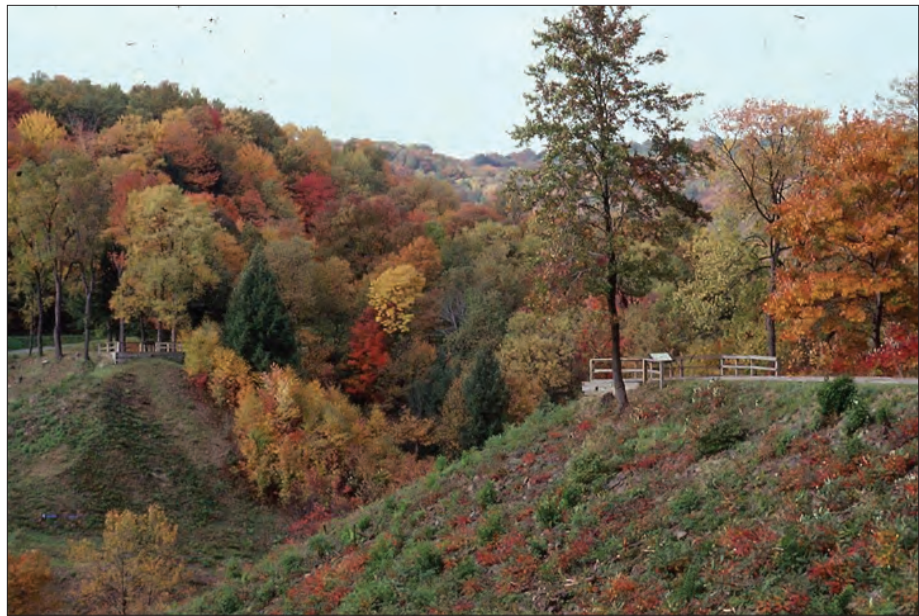
Figure 3.14. The dam abutments are visible here, circa 2000, when vegetation on the abutments was managed to control woody growth, circa 2000. (Johnstown Flood National Memorial)
