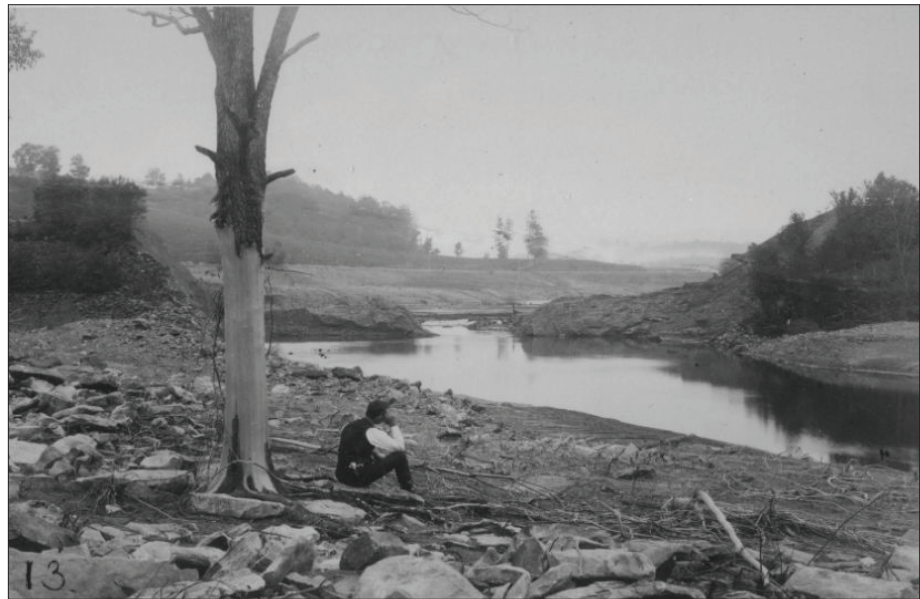
Figure 1.54. The view looking south towards the breach in the dam and the empty lakebed of Lake Conemaugh, circa 1889. (Johnstown Area Heritage Association)
