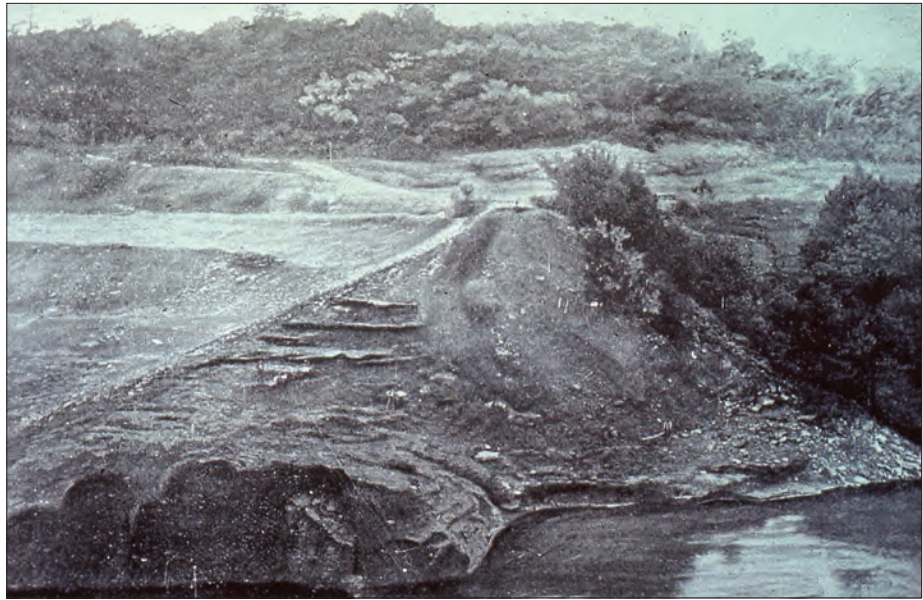
Figure 1.65. The South Fork Dam, edge of the South Abutment, looking southwest toward carriage drive, No Date. (Johnstown Flood National Memorial)
