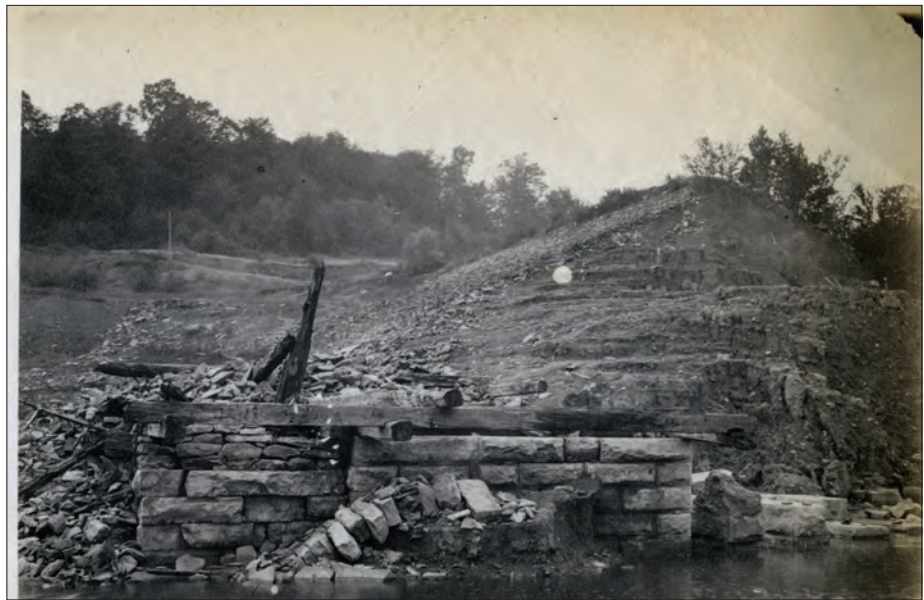
Figure 1.68. The South Fork Dam Sluice, circa July 1889. (Johnstown Flood National Memorial)
