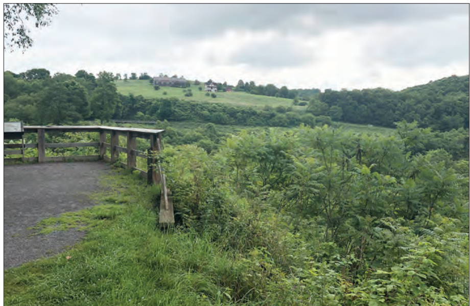
Figure 2.16. View from the south abutment, across the lakebed toward Lake View Farm and the Visitor Center, 2018. (Olmsted Center for Landscape Preservation)
