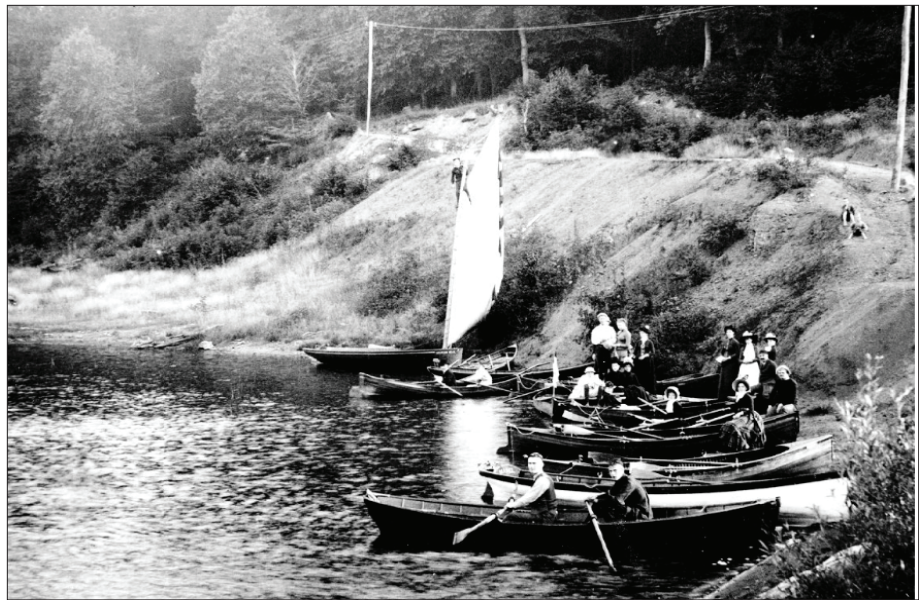
Figure 1.31. A group of members of the South Fork Fishing and Hunting Club sit at the edge of Lake Conemaugh at the base of the South Fork Dam, near a boat put in where the carriage road met the base of the south abutment. The carriage road is visible in the background of the photograph. Also note the grassy banks at the lake edge. (Louis Semple Clarke Collection, Johnstown Area Heritage Association).
