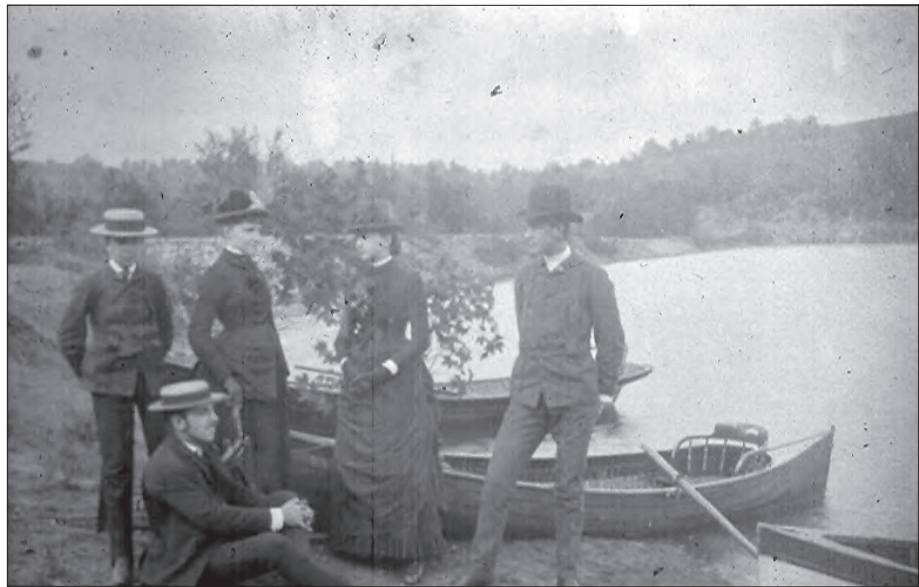
Figure 1.49. In this photograph, looking northeast from the far northwest corner of the lake near the dam, the breast of the dam is visible. The proposed sewerline would extended from the cottages, along the southwestern shore of the lake to this location, and then over the breast of the dam. As a number of photographs show boats docked in this location, this was likely the location of a boat launch. (Louis Semple Clarke Collection, Johnstown Area Heritage Association)
