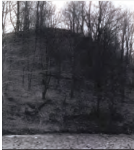
Figure 1.89. These photographs from "Reconnaissance Report" detailing feasibility of a future Johnstown Flood National Memorial, show the "left" or south abutment on left and "right" or north abutment on right, bottom photograph taken from corner of entrance drive to park and south abutment. (National Park Service, ETIC files)
