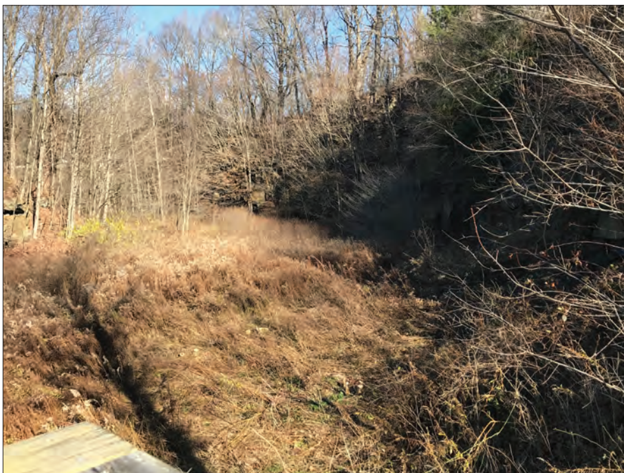
Figure 5.2. Looking north up the spillway just prior to clearing, 2020. (Johnstown Flood National Memorial)
