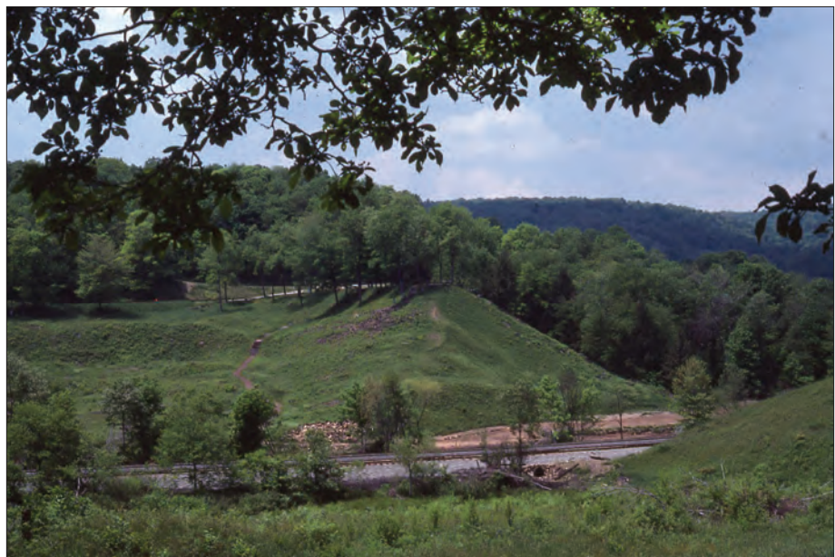
Figure 1.107. The lakebed and south abutment following clearing in 1989, evidence of scouring from flooding is visible along the river’s edge. (Johnstown Flood National Memorial).
