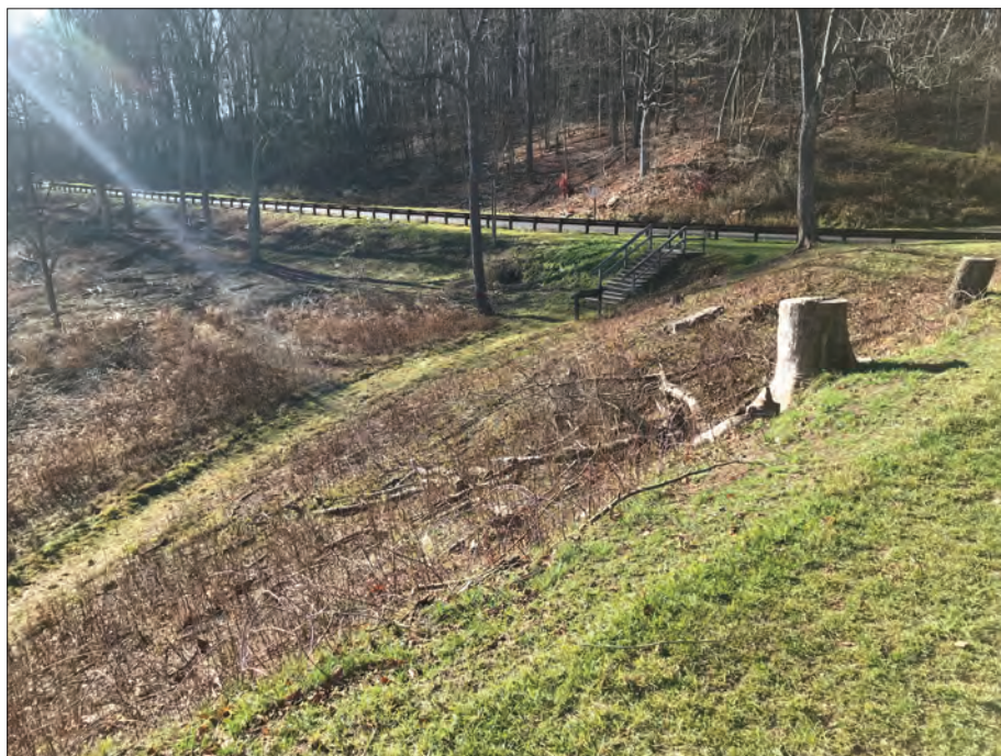
Figure 5.4. Here along the earthen embankment of the south abutment, removals included some large trees, that blocked views and also threatened to damage the historic earthworks, 2020. (Johnstown Flood National Memorial)
