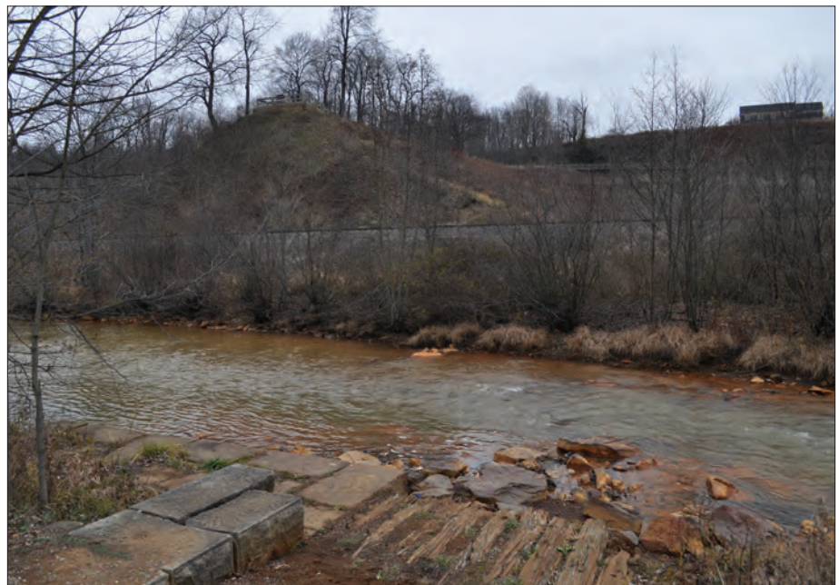
Figure 3.16. The remnants of the wood and culvert foundation stones are near the toe of the dam along the South Fork of the Little Conemaugh River, 2014. (Olmsted Center for Landscape Preservation)
