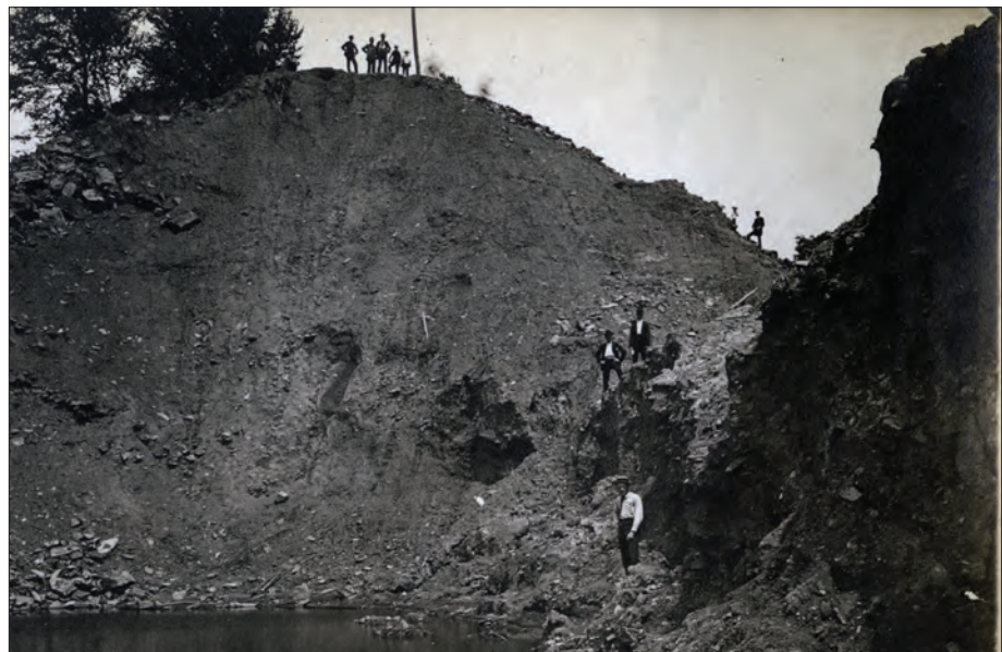
Figure 1.69. The South Fork Dam, edge of the North Abutment, (East edge of the dam break) July 28, 1889. (Johnstown Flood National Memorial)
