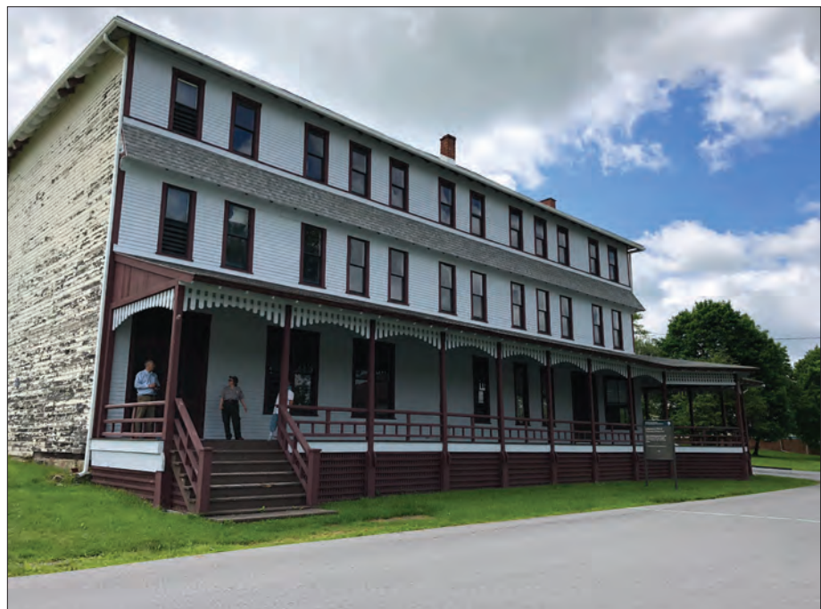
Figure 2.14. In this view of the clubhouse, the gravel parking area is visible in the lower right hand corner of the photograph, 2018. (Olmsted Center for Landscape Preservation).
