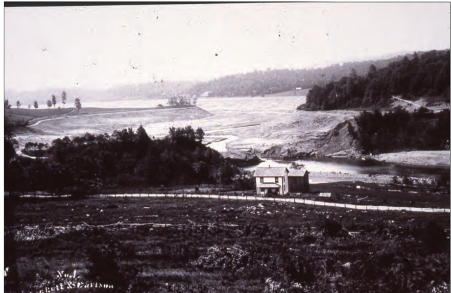
Figure 1.66. The view looking south towards the breach in the dam and the empty lakebed of Lake Conemaugh, from the hillside north of the dam. The carriage road climbing the hill side is clearly visible in the upper right hand corner. (Johnstown Flood National Memorial)
