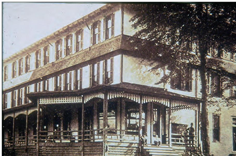
Figure 1.36. This photograph shows the 1887 addition of the club house. The photo, circa 1907–1920, was taken when the clubhouse functioned as the Sechler Hotel. (Photograph from the Costlow Collection, Johnstown Area Heritage Association)
