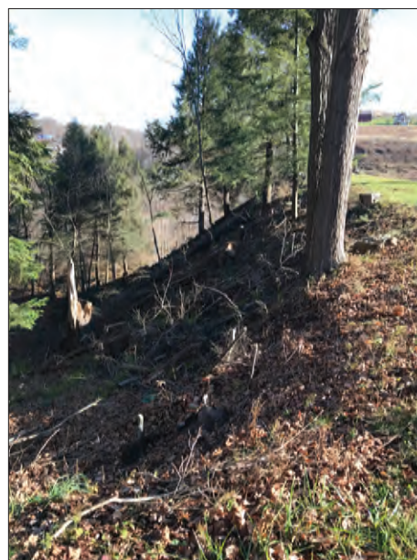
Figure 5.13. In the selective removals process on the downstream side of the south abutment, some trees were retained to screen noise and visual pollution from the adjacent highway, 2020. (Johnstown Flood National Memorial)
