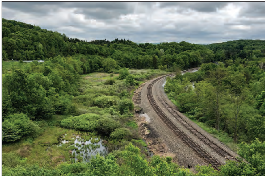
Figure 2.3. The culverts and berm from the late nineteenth century rail line concentrate water runoff in discrete areas of the lakebed supporting the growth of wetlands, 2019. (Olmsted Center for Landscape Preservation)
