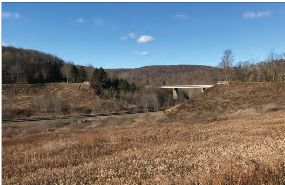
Figure 5.11. The north and south dam abutments are visible again, with tree clearing still in process, 2020. (Johnstown Flood National Memorial)
