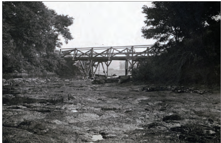
Figure 1.25. A detail from a photograph of the trestle bridge over the spillway looking southeast immediately after the flood, 1889. (Johnstown Flood National Memorial Archives)
