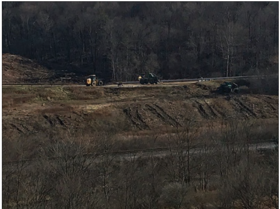
Figure 5.5. The Masticator at work near the rail line in the Lakebed, 2020. (Johnstown Flood National Memorial)
