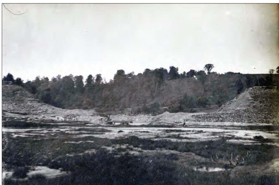
Figure 1.64. The South Fork Dam, edge of the South Abutment (West edge of the dam break), July 28, 1889. (Johnstown Flood National Memorial)
