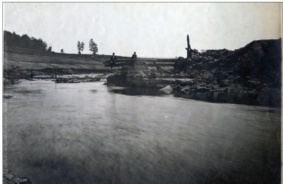
Figure 1.55. The South Fork Dam Sluice Gate, following the flood, looking south through the breach in the dam, circa July 1889. ((Johnstown Flood National Memorial).
