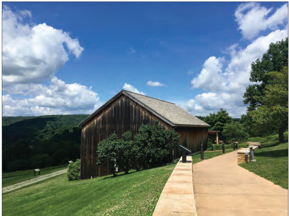
Figure 2.7. The entrance to the barn-like Visitor Center includes stone retaining walls, concrete sidewalks and plantings of herbaceous perennials and shrubs, 2018. (Olmsted Center for Landscape Preservation)
