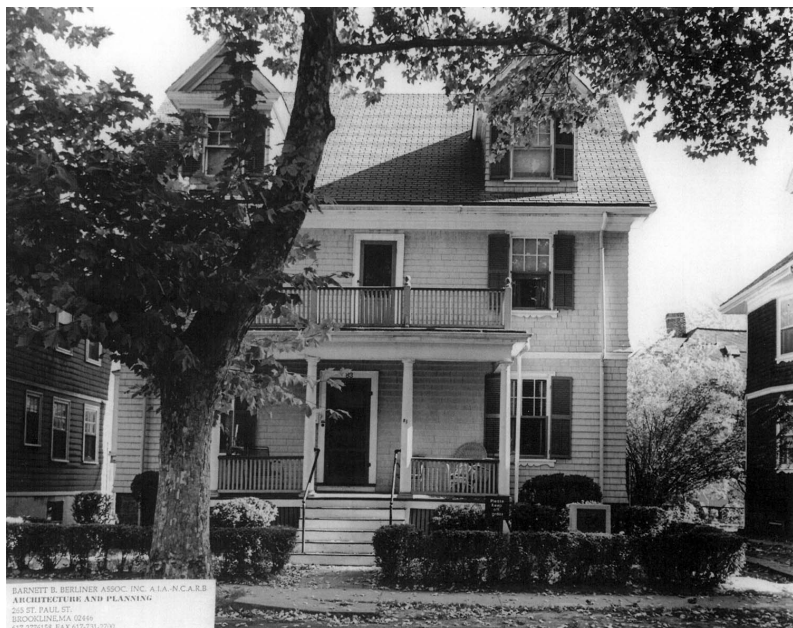
Figure 8. View of northwest elevation, October 1964, shows the privet hedge, commemorative marker, yew planting, and sod installation (Irene Shwachman, 1964, Private collection of Mr. Robert Berliner, copies reside in the JOFI Management Records).
