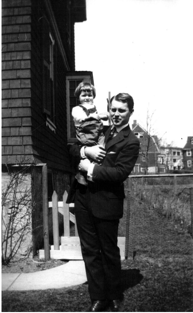
Figure 5. Joseph P. Kennedy Sr. and Joseph P. Kennedy Jr., undated, likely 1917. By the east corner of the house at 83 Beals, a concrete walk provided access to the rear yard (Kennedy Family Collection, copyright John F. Kennedy Library Foundation).
