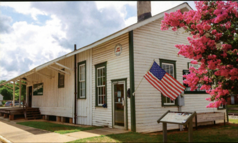
PLAINS DEPOT 100 West Main Street. The depot was completed in 1888. The town, then named Plains of Dura, moved a short distance south to take advantage of the new railroad and shortened its name to Plains. In 1919, 66 carloads of hogs and cows were shipped from the depot. In the 1920s, 6,000 to 10,000 bales of cotton were shipped annually from Plains. The building has been restored to its 1976 appearance as Carter's campaign headquarters.
