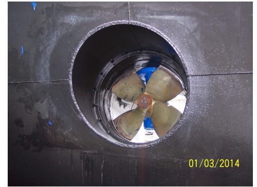
Bow thruster after cast iron housing was blasted clean, primed and coated with the latest protective "goop" to combat cavitation pitting that has required repair three times since 1998.
