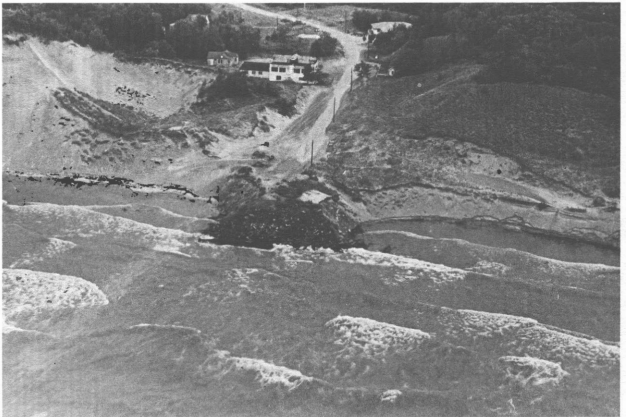
Figure 5. Lake currents undercutting old Lakeshore Drive at Central Avenue near Beverly Shores.
