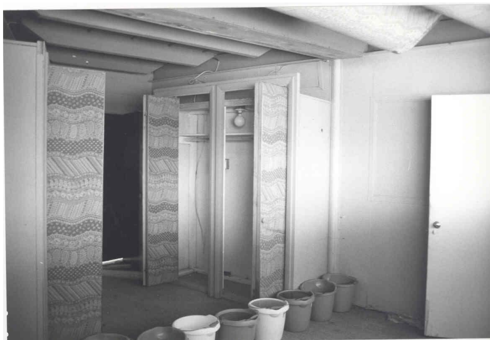
View 32 – Bedroom/Workshop – South Wall and Closets
