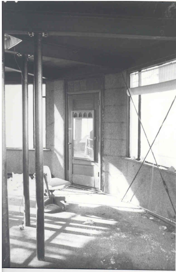
View 1 - Door to Roof Deck
