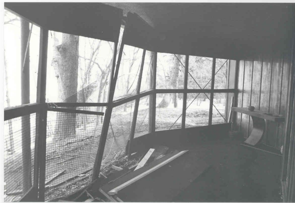
View 58 – Front Porch – Looking East
