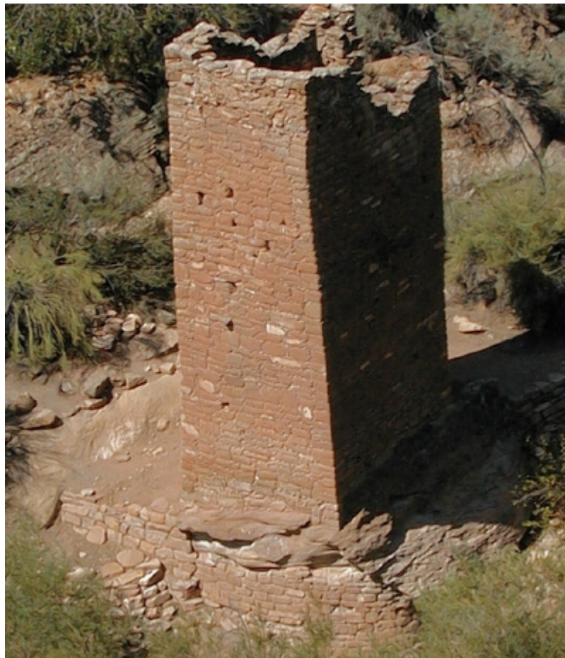
Figure 3: Square Tower at Hovenweep National Monument built on a slump block of Dakota Sandstone. The sandstone is being eroded due to the presence of a nearby stream. The National Park Service built the stabilizing wall below the boulder in 1960. Photograph by Anne Poole, NPS.
