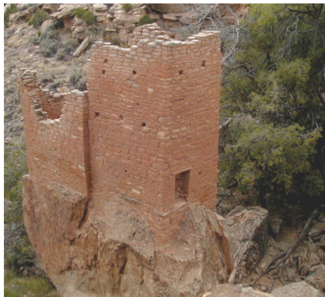
Figure 10: Holly Unit, Hovenweep National Monument. Dwelling is constructed on Dakota Sandstone that has subsequently been subjected to erosion, leaving the ruin in a precarious position. This is probably the ruin called "Holly Tower" in Fewkes, 1919, (figure 9, C). Photograph by Anne Poole, NPS.
