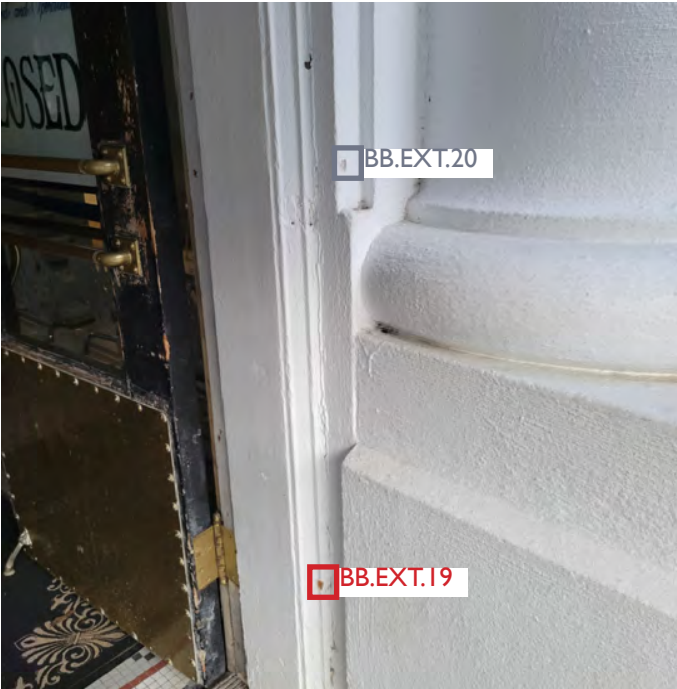
West elevation 1F, front door
