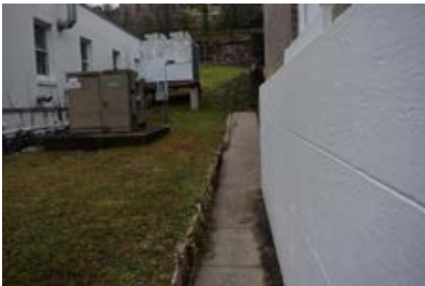
Figure 1.D.83. Concrete walk north of the bathhouse, which includes a stone curb to retain the turfgrass area between Buckstaff and Ozark. The walk provides access to the north stair. View to east (WLA Studio, 2025).
