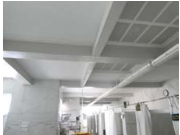
Figure 1.D.27. Beams, girders and slabs in finished spaces are completely covered in plaster and painted.
