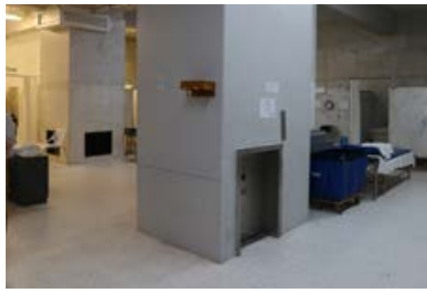
Figure 1.D.76. The company added the dumbwaiter through the bath halls in 1967.
