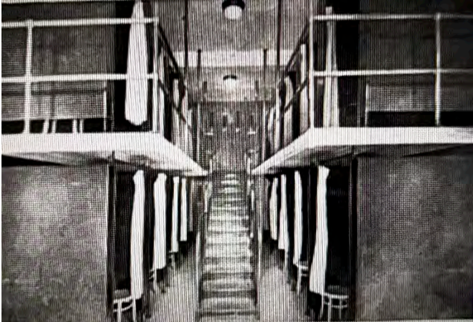
Figure 21. Image of north Men's Dressing Room (Room 110) c. 1916, view looking east. (Image extracted from current HSR, Figure 1B.12)
