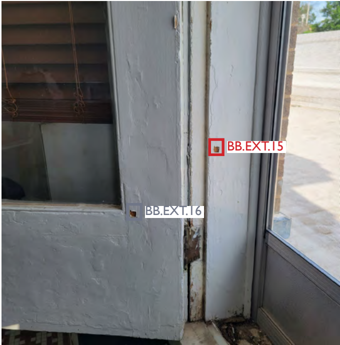
North elevation roof, door
