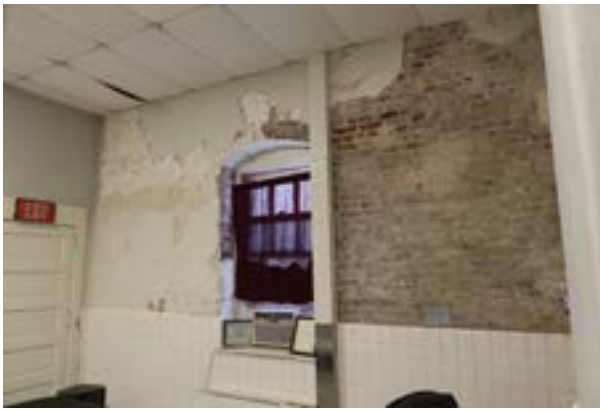
Figure 1.D.66. Interior plaster wall surfaces are in good condition overall except at areas where water infiltration has caused damage. The east wall of room 107 exhibits the worst plaster damage in the building. The ceramic tile wainscoting is believed to date from the 1950s and is in good condition overall.
