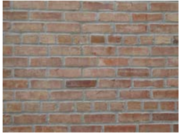
Figure 1.D.36. These walls were laid in common bond with header brick tying the various wythes together every 6 th course to form a monolithic assemblage.
