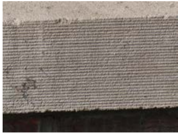
Figure 1.D.40. A few of the original limestone windowsills were left unpainted on the east elevation. The original profile is still visible which is called a "X cut" with X being the number of grooves per inch as the stone was fabricated.
