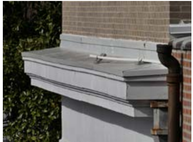
Figure 1.D.47. Sheet metal has been installed on top of the stone cornice of both the main and upper roof levels.
