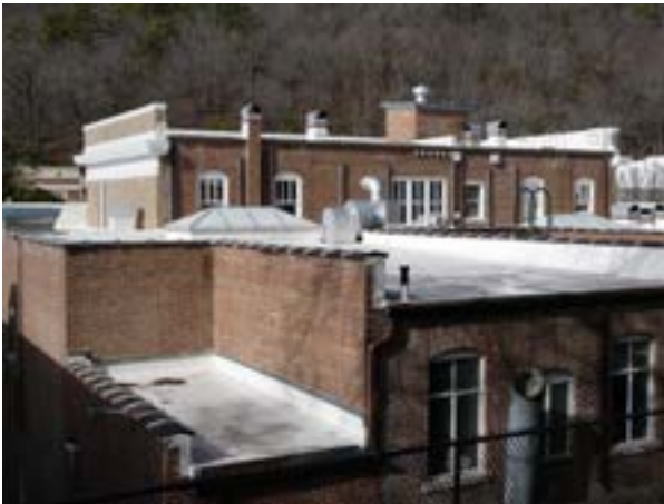
Figure 1.D.35. Light reddish buff brick were used to face walls which were not readily visible from the street.
