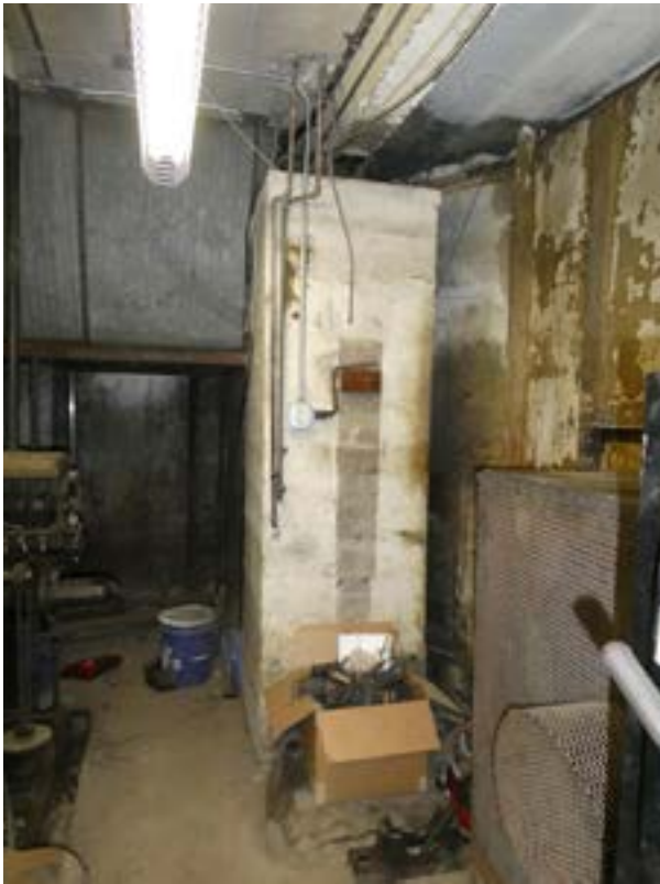
Figure 1.D.19. These became relatively tall piers in the full depth portion of the basement.
