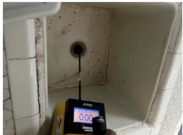
Photo 12 Screening drains near identified rooms.
