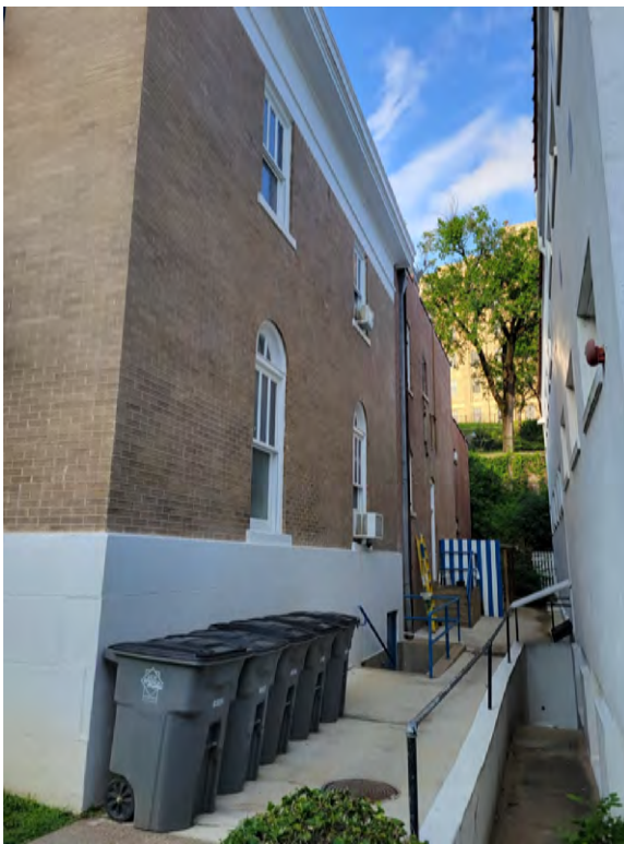
Figure 2. South elevation, view looking northeast.
