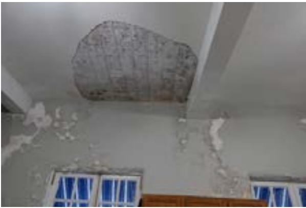
Figure 1.D.69. Plaster ceiling finishes are in good condition overall. This area below a major roof leak in room 300 exhibits some of the worst plaster damage in the building.
