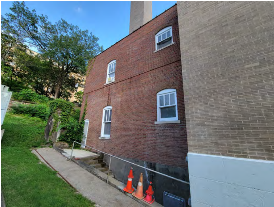
Figure 4. Rear of north elevation, view looking southeast.
