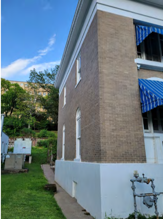
Figure 3. North elevation, view looking southeast.
