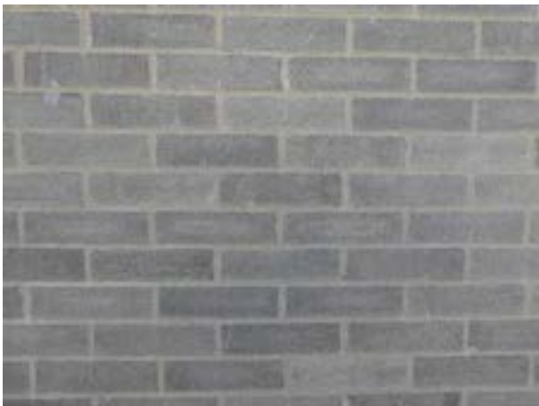
Figure 1.D.31. The blonde ironspot brick are laid in running bond.
