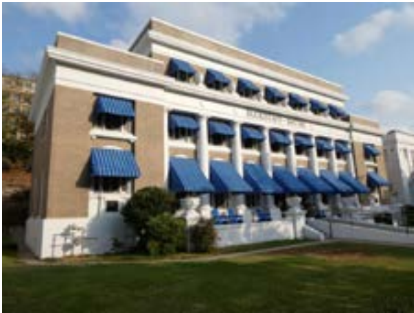
Figure 1.D.30. The west elevation façade is constructed of blonde ironspot face brick with limestone accents. All of the stone has been painted white.
