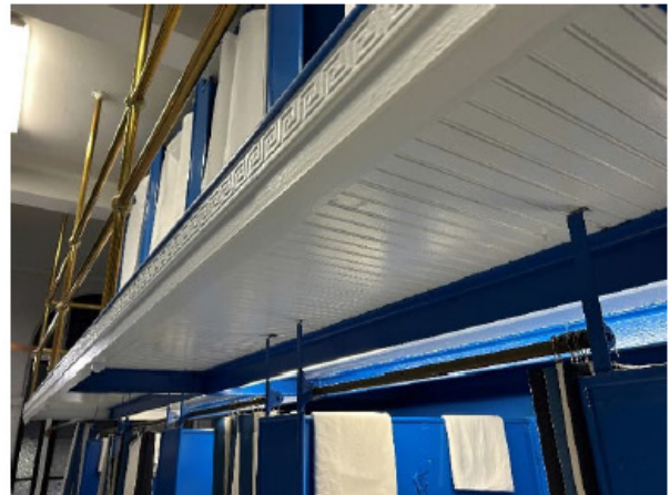
Photo 10 Overview of the interior of the bath house.
