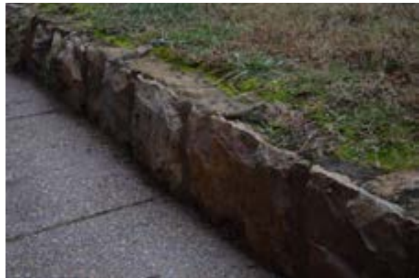
Figure 1.D.84. Detail view of the stone curb wall adjacent to the north walk. The stones and construction are similar to the North Retaining Wall east of the building. View to northwest (WLA Studio, 2025).
