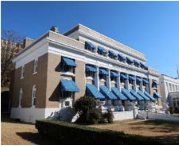
Figure 1.C.1. Figure 1. Character-defining features of the site and exterior include the Magnolia Promenade, turf grass lawn, holly hedges, exposed-aggregate concrete walkways, the overall massing and composition of the building, the terrace (with its urns, ramp, and steps), exterior materials (stone, brick), historic windows (wood, metal, and steel) and seasonal awnings, and glazed and paneled wood doors.
