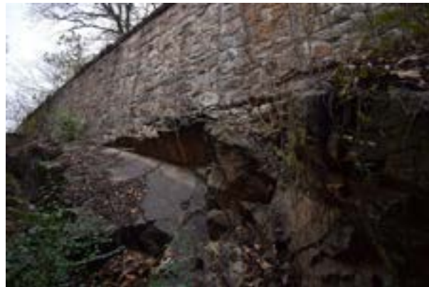
Figure 1.D.93. South retaining wall, set on exposed rock outcrop. The stones are mortared and irregular in an irregular pattern. The wall has a limestone cap. View to north (WLA Studio, 2025).
