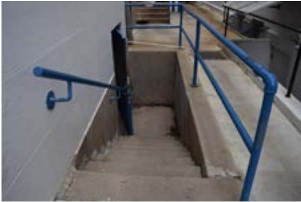
Figure 1.D.82. View of the south side of the Buckstaff Bathhouse, which includes a walk that leads to two sets of stairs and the rear of the building. The concrete area between the stair wells of the buildings (photo right) is graded to provide drainage to the inlet shown in the photo (WLA Studio, 2025).
