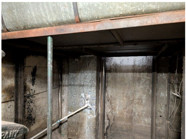
Space below Elevator Pit
