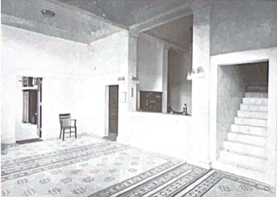
Figure 12. Image of Lobby (Room 100) in 1912, view looking northeast. (Image extracted from current HSR Figure 1B.9)
