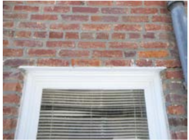
Figure 1.D.46. Loose steel lintels support the masonry above several of the windows.
