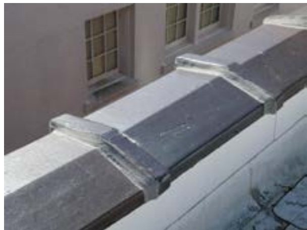
Figure 1.D.42. The Vitreous Clay Tile (VCT) cap and chinking mortar is in good condition.
