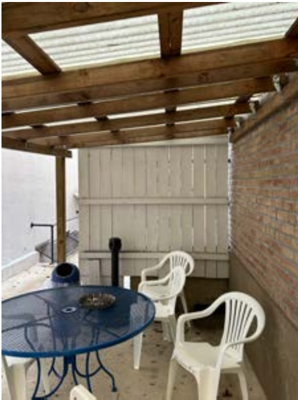
Figure 1.D.99. A wood shed structure with corrugated plastic provides cover for a staff break area on the south side of the building. There is a painted wood screen installed between the break areas and the west side of the building to screen it from the public view. View to the West. (WLA Studio, 2025)
