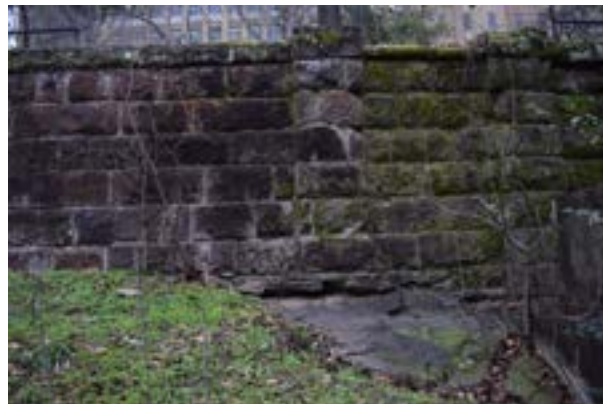
Figure 1.D.94. North retaining wall, set partially on exposed rock outcrop. The stones are rectangular-shaped and mortared in an ashlar pattern. Square stone piers are spaced throughout the wall. View to east (WLA Studio, 2025).
