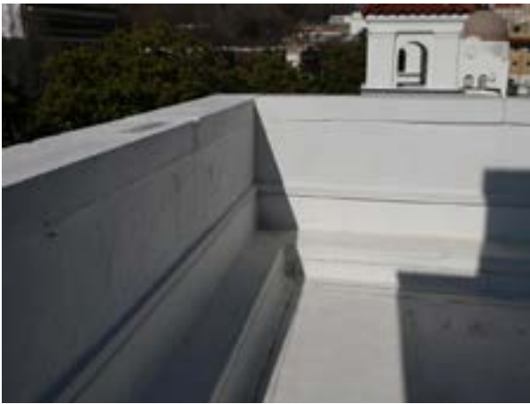
Figure 1.D.59. This membrane extends up the interior face of the parapet.
