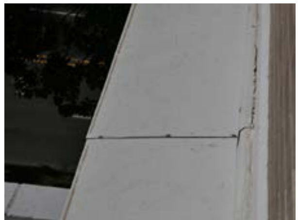
Figure 1.D.48. The laps are screwed together.
