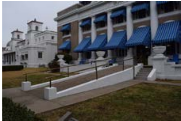
Figure 1.D.85. Front ramp entry and stairs. Stairs flank both sides of the ramp. View to northeast (WLA Studio, 2025).
