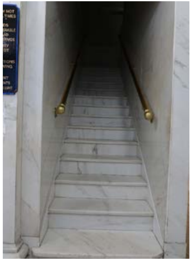
Figure 1.D.65. Marble and brass components at front stair (S1).
