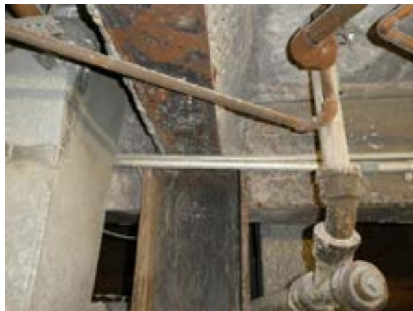
Figure 1.D.22. Location where a steel beam and girder connect into a steel column. The sides of the beams and girders are encased in concrete.
