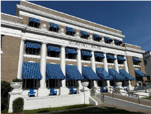
Photo 1 Exterior of the Buckstaff Bath House
