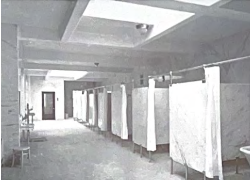
Figure 45. Image of Women's Bath Hall, 1912. (Image extracted from current HSR Figure 1B.16).
