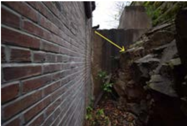
Figure 1.D.90. Exposed rock outcrop (indicated) on the east side of the Buckstaff Bathhouse. The outcrop serves as a foundation for the mortared retaining wall above. View to north (WLA Studio, 2025).
