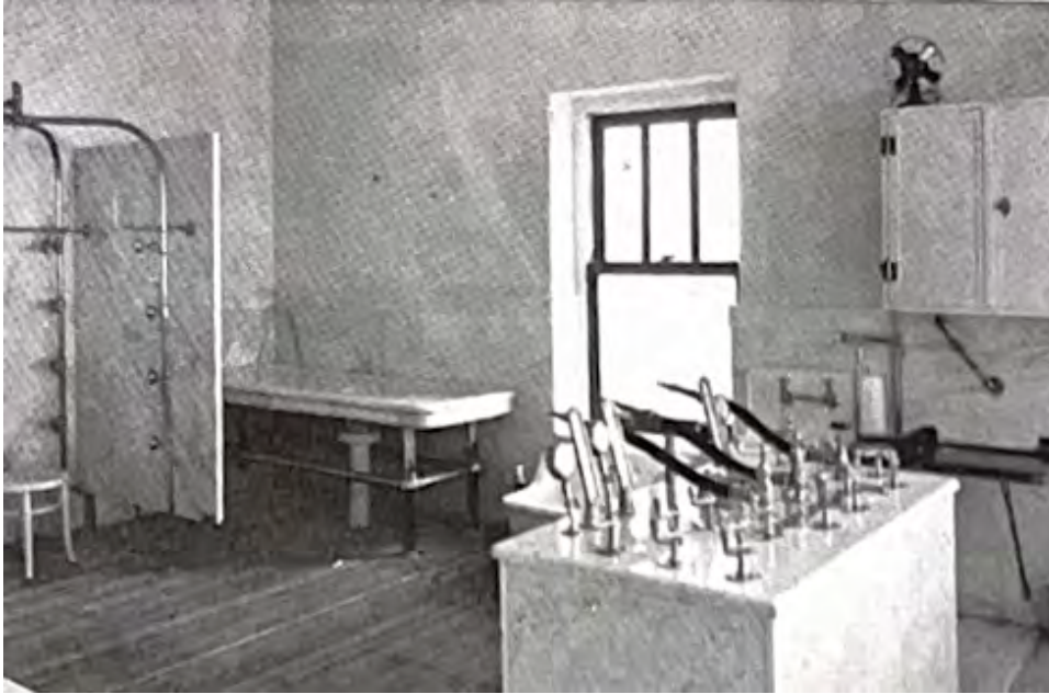
Figure 36. The Hydrotherapeutic Department in 1912, currently Room 205. Note the dual-color scheme on the window with dark sash and light frame, which may also have been applied to the Men's Cooling Room. (Image extracted from current HSR, Figure 1B.14).
