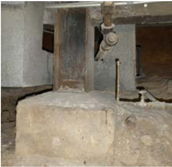
Figure 1.D.18. Concrete foundations in the crawlspace.
