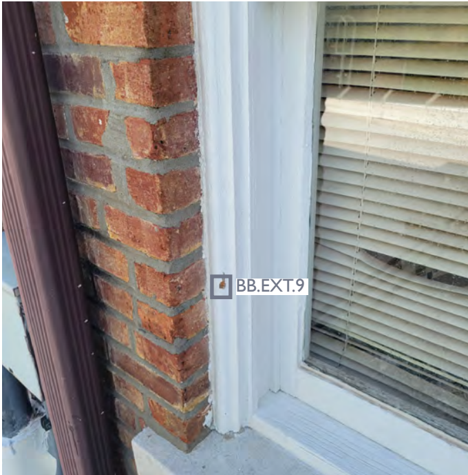
East elevation roof, window
