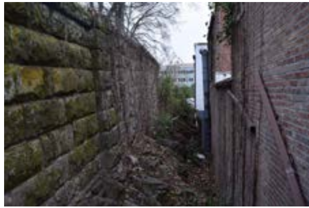
Figure 1.D.92. Narrow area between the east side of the building and the stone retaining wall. The north and south retaining walls are visible in this photograph. View to south (WLA Studio, 2025).
