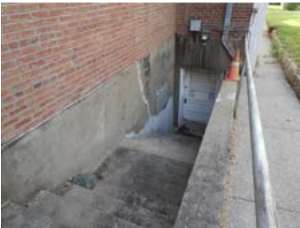
Figure 1.D.14. Concrete wall and stairs leading down to the basement level.
