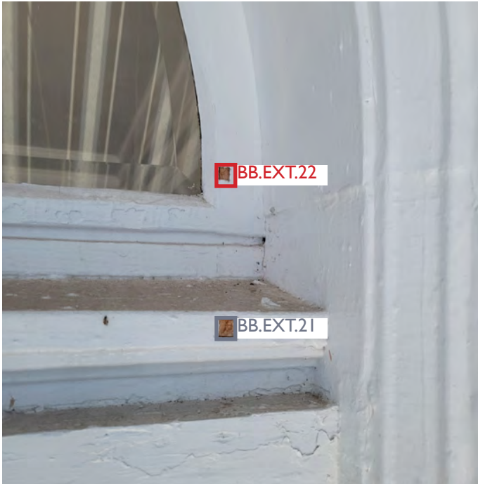
West elevation 1F, front door
