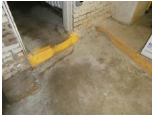
Figure 1.D.20. The floor height changes numerous times within the basement.
