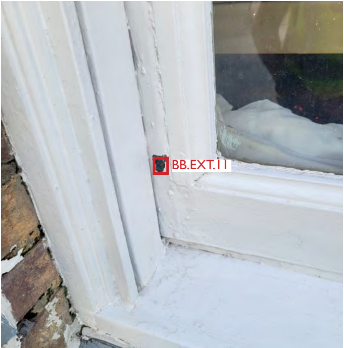
East elevation roof, window
