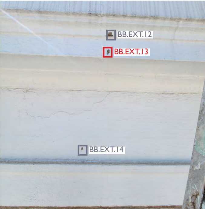
North elevation roof, cornice
