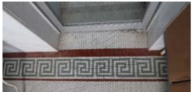
Figure 1.D.72. Mosaic tile floor patterns vary. Nine rooms have borders and field patterns, while six more have borders alone with white fields.
