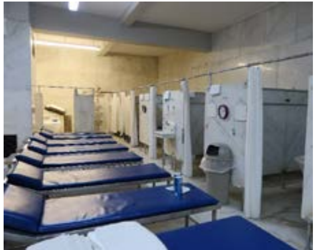
Figure 1.C.4. Character-defining features of the interior that can be seen in the men's bath hall (106) include flat plaster ceilings, mosaic tile floors, marble wall panels and partitions, and historic plumbing fixtures.
