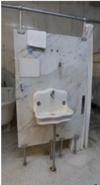
Figure 1.C.5. Character-defining historic plumbing fixtures in the bath halls including tubs, sitz baths, sinks, needle showers, and steam cabinets.
