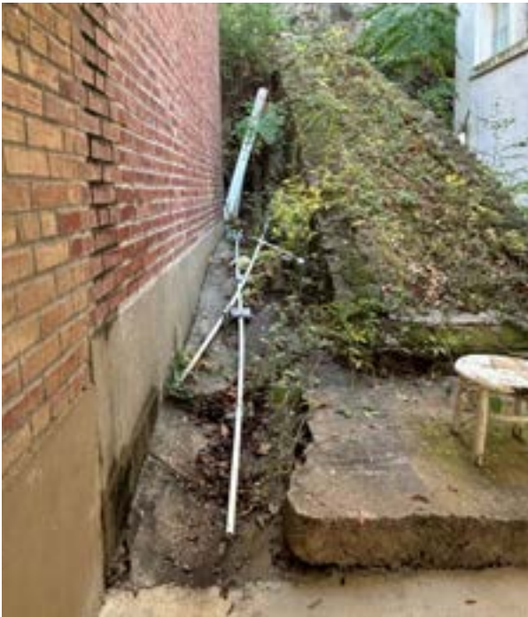
Figure 1.D.88. Paved area between the southeast corner of the bathhouse and the stone buttress/ramp is paved with concrete, sloped to facilitate drainage from behind the building to the surface drainage south of the building. The concrete is in fair condition with cracking and debris present (RATIO, 2025).
