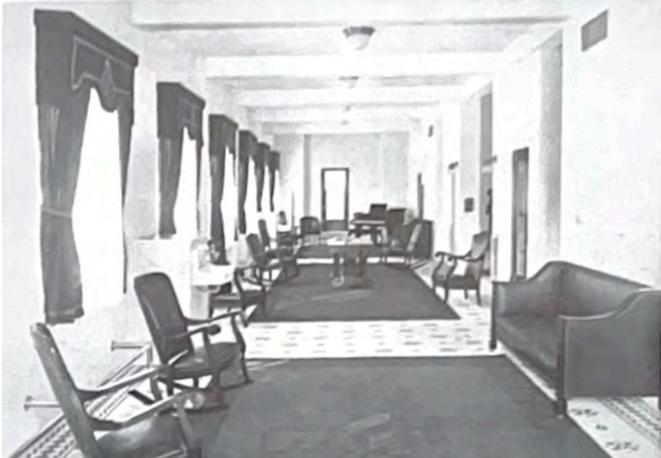
Figure 53. Image of third floor Lounge Room in 1912, now the Hall (Room 300A) and Manicure/Pedicure Room (300C), view looking north. (Image extracted from current HSR IB.18).
