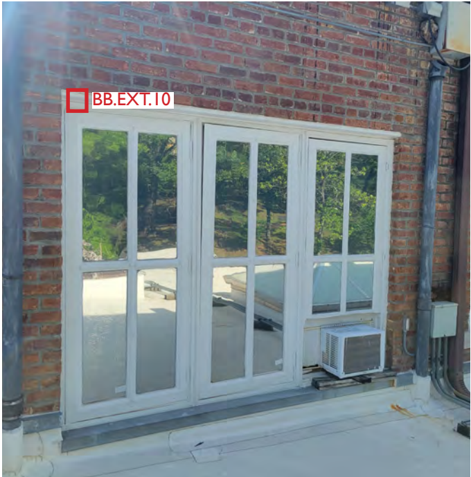
East elevation roof, window
