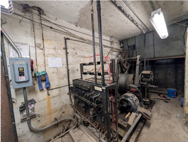
Elevator machine room
