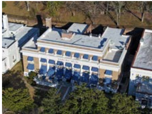
Figure 1.D.57. Aerial view of the various roof levels looking east.
