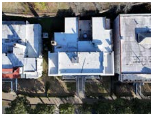
Figure 1.D.58. All of the major sections of roof are covered with a TPO membrane.
