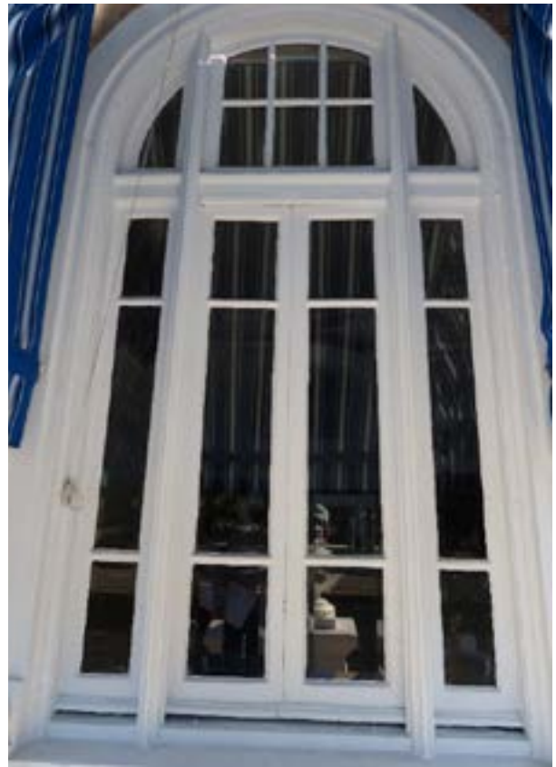
Figure 1.D.54. Typical wood windows at west façade.
