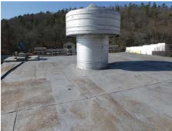
Figure 1.D.61. The roof of the elevator hoist is made of flat-lock terne metal.
