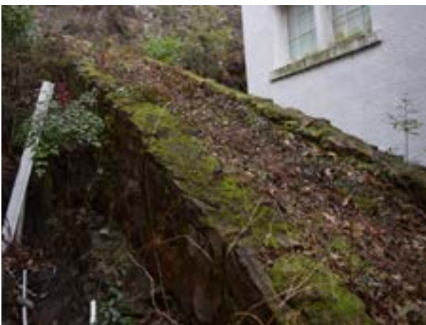
Figure 1.D.97. Stone ramp/buttness between Lamar and Buckstaff Bathhouses. The cheekwalls are mortared irregularly shaped stone. The surface once had turf growing in it, but vegetation now consists of moss, vinca, and nandina. View to southeast (WLA Studio, 2025).
