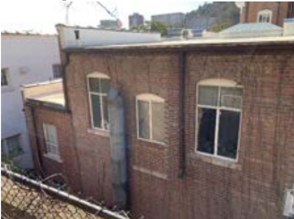
Figure 1.D.53. Some of the multiple types of steel sash windows at the rear wings.
