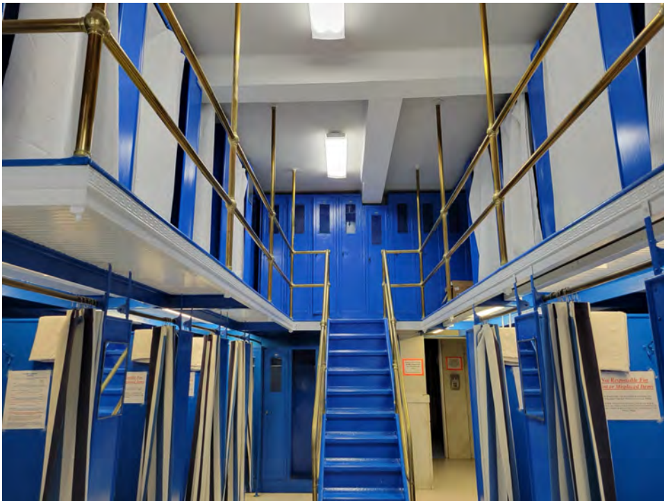
Figure 22. South Men's Dressing Room (Room 102) in 2025, view looking east.
