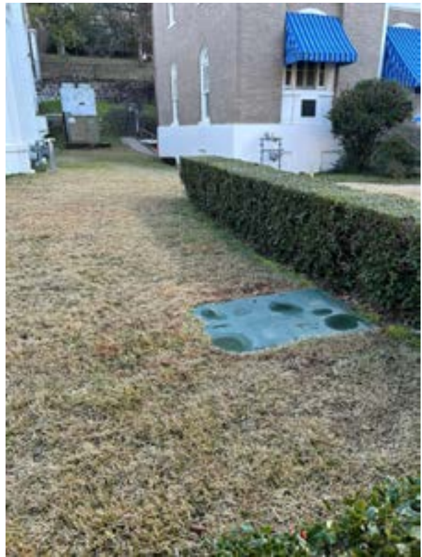
Figure 1.D.102. Access lid located on side lawn in front of the Buckstaff Bathhouse.
