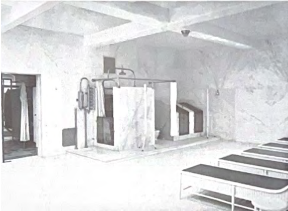
Figure 47. Image of Women's Bath Hall, 2025. (Image extracted from current HSR Figure 1B.17).
