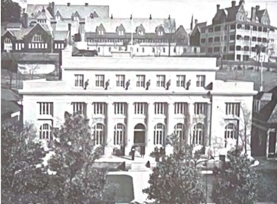
Figure 5. Photograph of Buckstaff Bathhouse in 1912. Note that all of the exterior elements have a very light color value except the front doors and its fanlight, which are very dark. (Image extracted from current HSR, Figure 1B.4)
