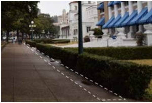
Figure 1.D.89. The east edge of the sidewalk is paved to facilitate drainage to three brass strip drains. While there is some ponding present, the system works to drain water from the concrete walk to a subsurface drainage system (WLA Studio, 2025).
