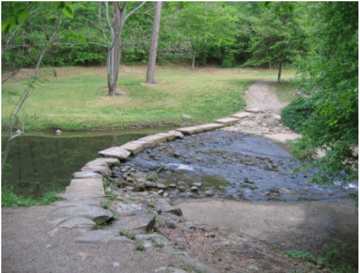
Remains of upper dam and current crossing steps (source: CLI inventory).
