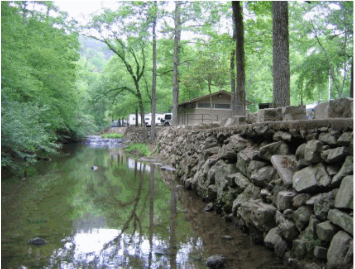
Stone retaining wall (source: CLI inventory)
