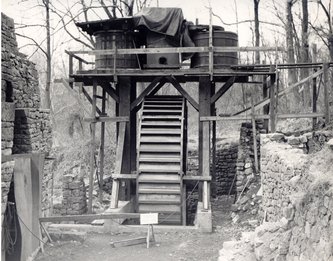
Figure 22 – Blast machinery and water wheel, 1951. (Hopewell Furnace National Historic Site Archives.)
