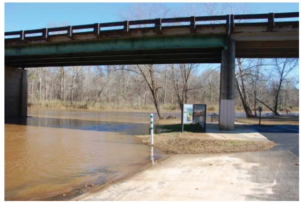
FIGURE 28. Boat ramp below Highway 49. NPS photo.
