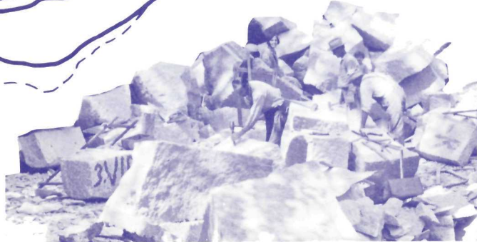
Hand-cutting stone to be used as facing for many of the Yosemite Valley bridges, 1929. Granite was quarried from rock slides or boulders within the park, and sand was taken from riverbeds or borrow pits. YRL
