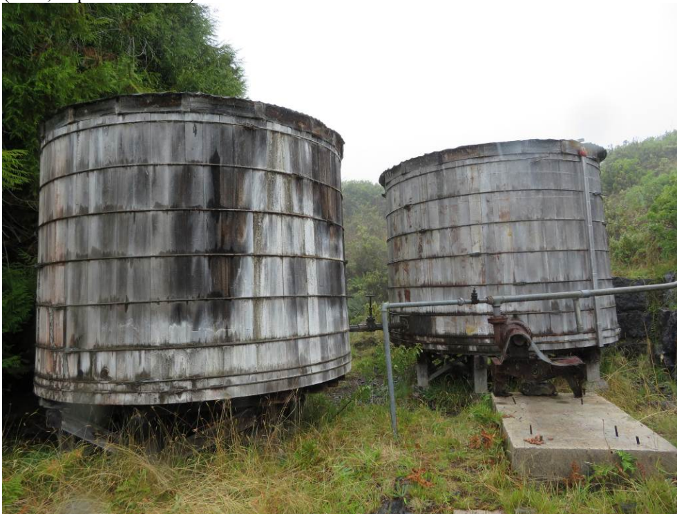
Buildings and Structures #3 McGee Spring Water Tanks (HS-14), view southeast (CRIS, 2018).
