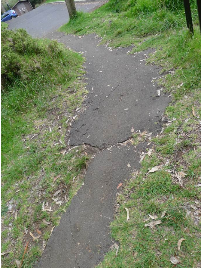
Circulation #5 Paved walkway to the Hosmer Grove Nature Trail trailhead, view south towards the parking lot (NPS, September 2018).
