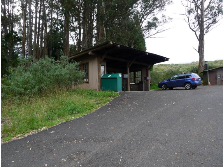
Land Use #2 Rain shelter and vault toilet to the east and southeast of the parking lot. View south-southeast (NPS, September 2018).
