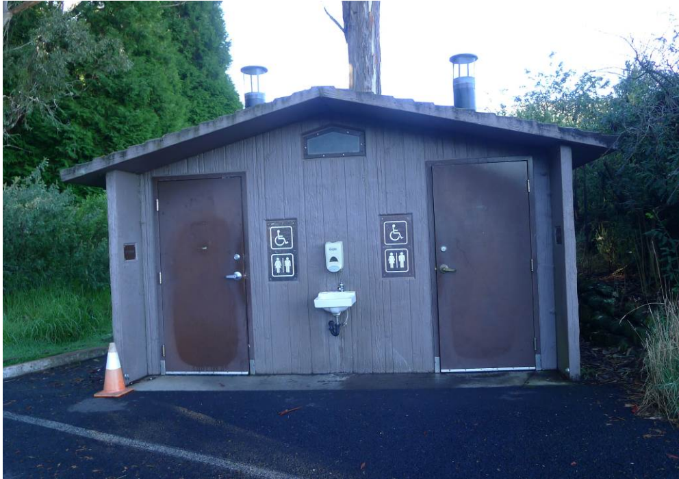
Buildings and Structures #4 Hosmer Grove Campground and Picnic Area vault toilet (HQ49), view southeast (NPS, September 2018).
