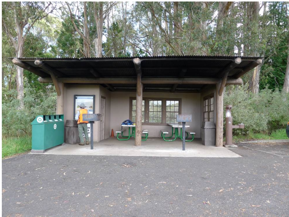
Buildings and Structures #1 Hosmer Grove Rain Shelter, view east (NPS, September 2018).
