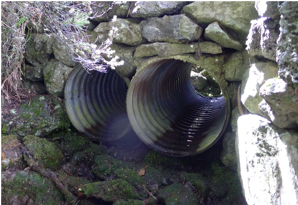
Buildings and Structures #7 Footbridge and culvert across the gully near the trail end of Hosmer Grove Nature Trail (NPS, September 2018).
