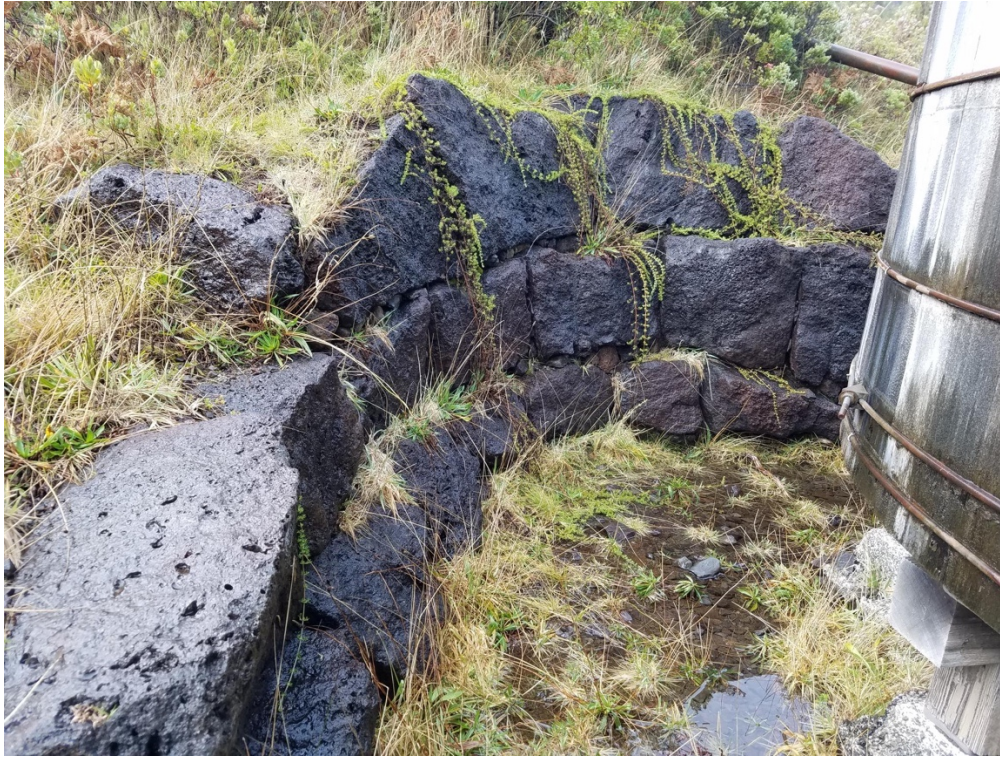
Buildings and Structures #8 McGee Springs rock retaining wall behind, upslope of the McGee Springs Water Tanks (NPS, 2019).
