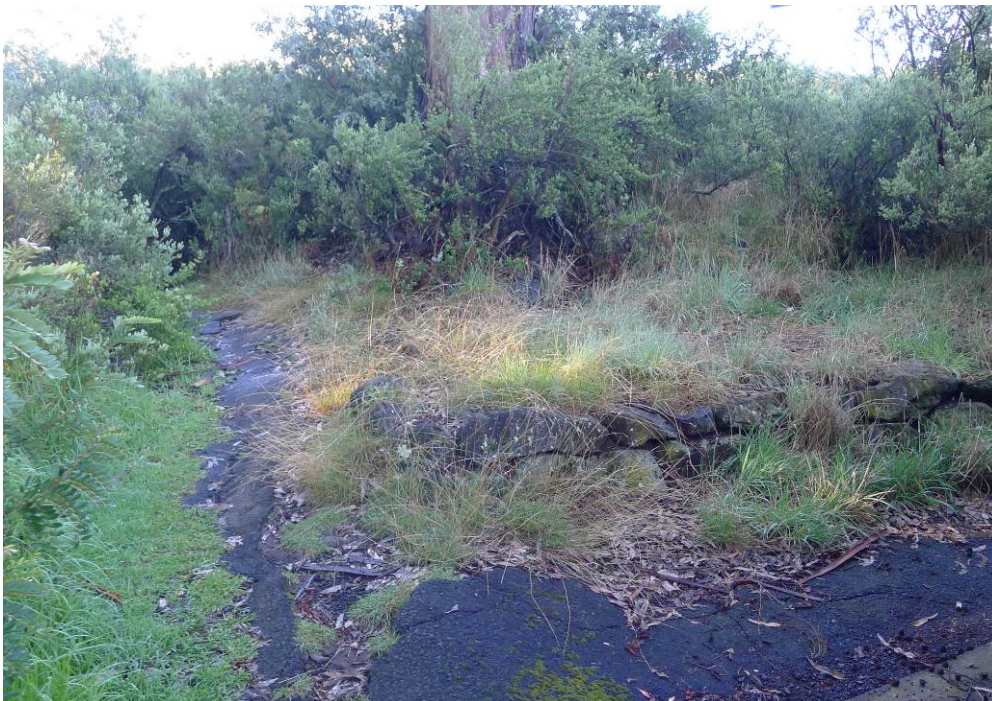
Buildings and Structures #5 Rock Retaining Wall behind the vault toilet, view southeast (NPS, September 2018).
