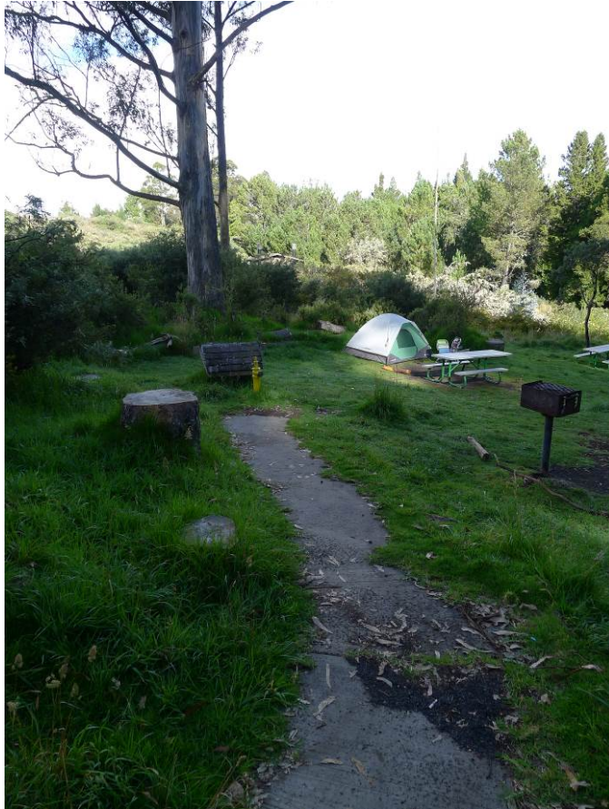
Circulation #4 Paved walkway into the campground and picnic area, view northwest (NPS, September 2018).
