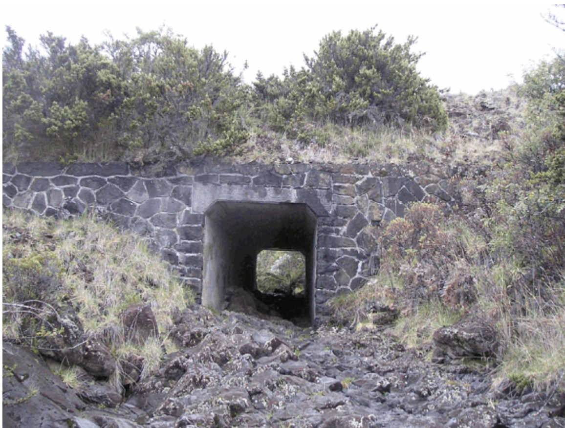
Example of a historic box culvert with a random course pattern along the Haleakala Highway. (PWRO 2006)
