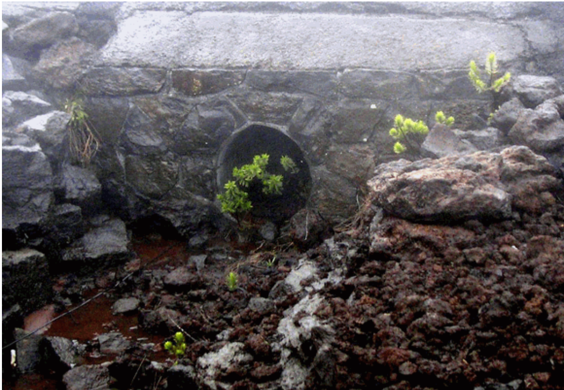
Historic culvert with a random course pattern along the Haleakala Highway. (PWRO 2006)
