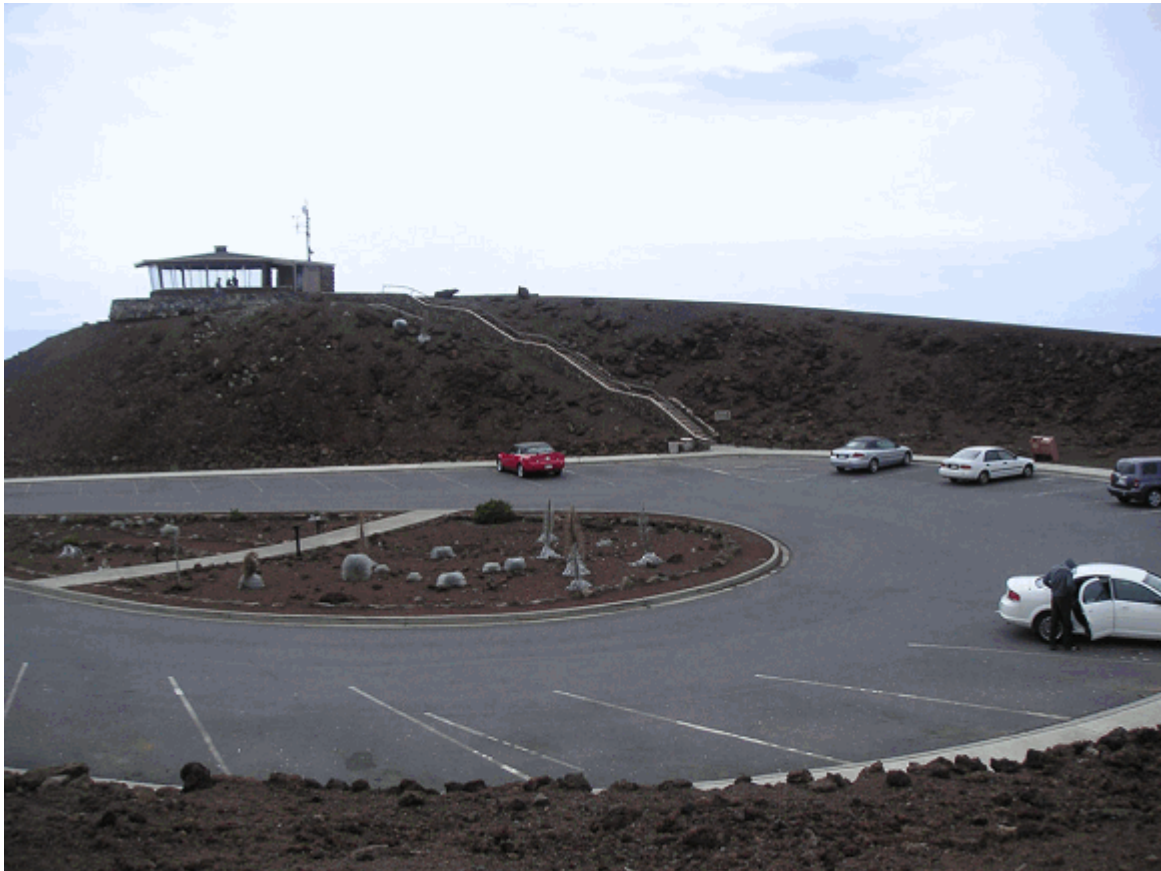
Red Hill parking lot, sidewalks, and stairs. (PWRO 2006)
