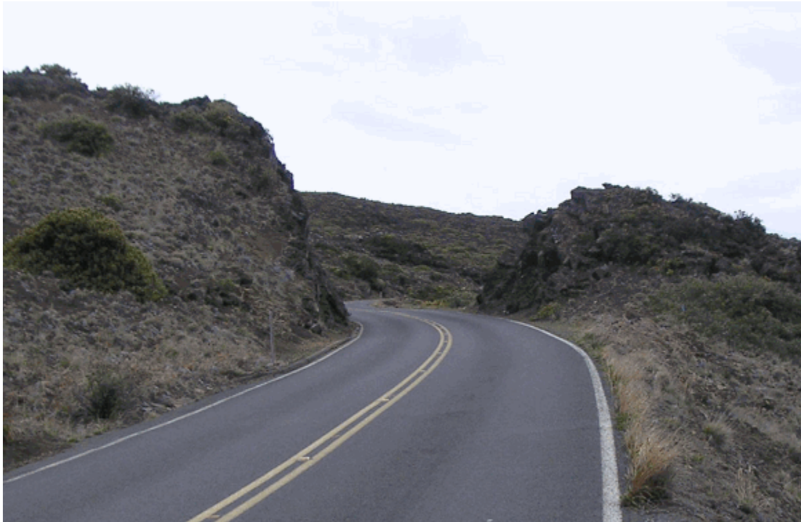
Road alignment winding through a rock cut. (PWRO 2006)
