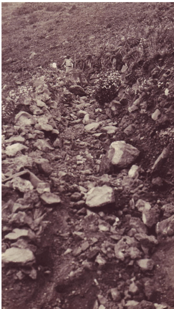
Halemau'u Trail storm damage, 1937 (Haleakala National Park archives).
