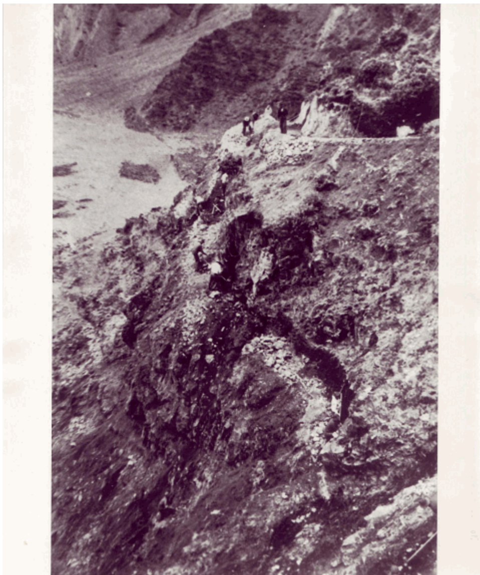
CCC crews working on the Halemau'u Trail switchbacks, 1937 (Haleakala National Park archives).
