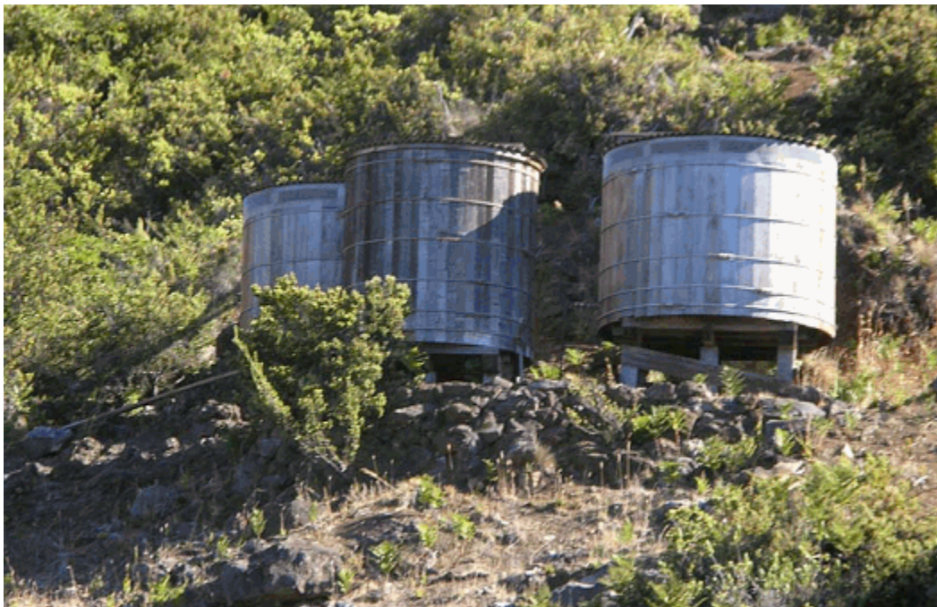
Buildings and Structures #5: Kapalaoa water tanks, located on a slope a short distance west of the Kapalaoa Cabin. In 2006, the middle tank was rehabilitated, while the two remaining tanks were replaced in-kind (PWRO, 2008).
