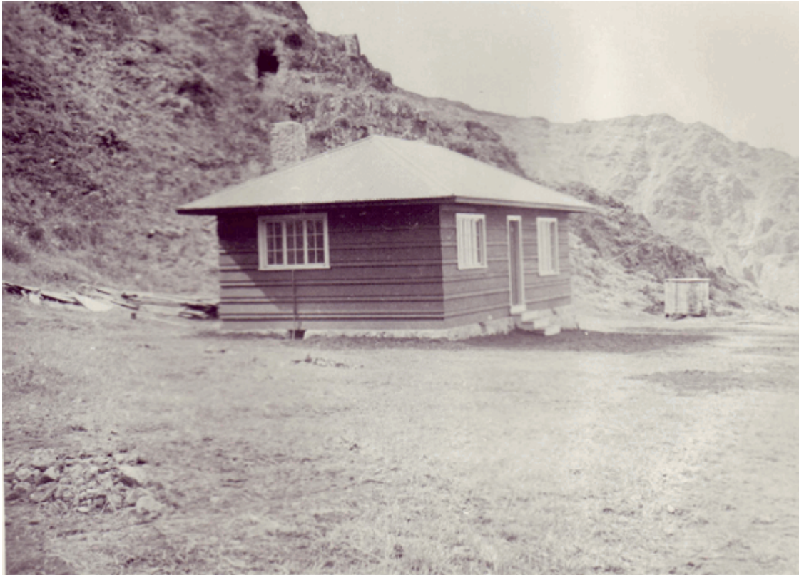
Holua Cabin, just after completion in 1937 (Haleakala National Park archives).
