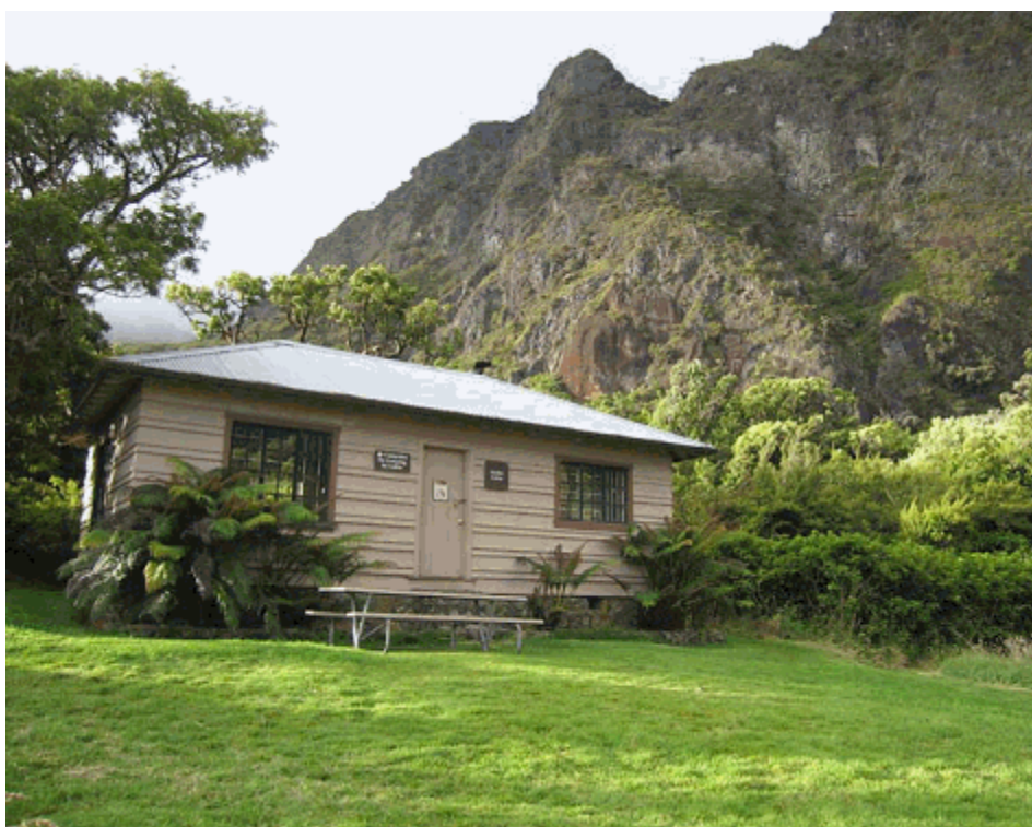
Buildings and Structures #2: Paliku Cabin, located in the lushly vegetated eastern extent of Haleakala Crater (PWRO, 2008).
