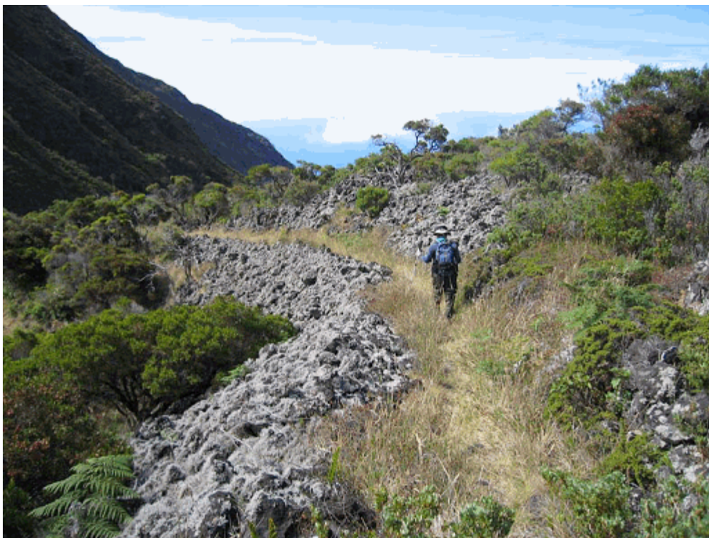
Circulation #6: Lichen-covered rip rap retaining wall along Kaupo Trail (PWRO, 2008).
