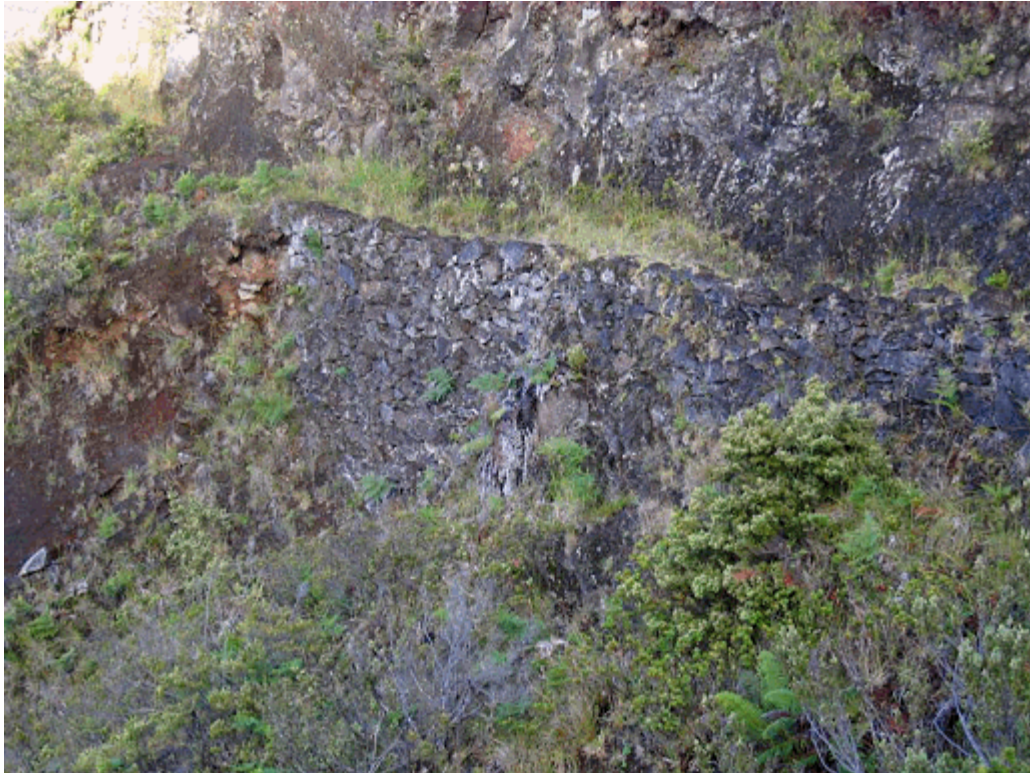
Buildings and Structures #7: Stone retaining wall associated with the Halemau'u switchbacks. Note the rustic character of the wall as it seamlessly blends with its surrounding environment (PWRO, 2008).
