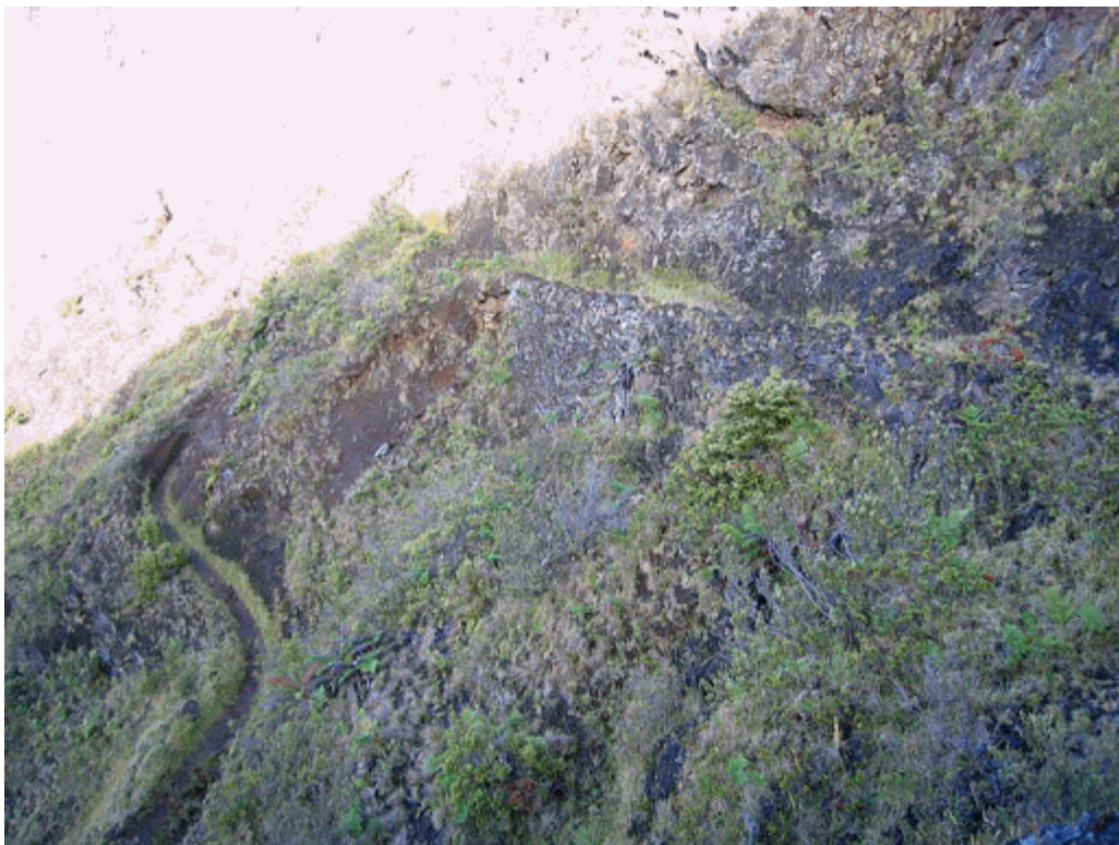
Circulation #4: Switchbacks and associated stone retaining walls along the Halemau'u Trail as it ascends out of the crater. Notice how the trail follows the topography, while blending with the natural environment (PWRO, 2008).
