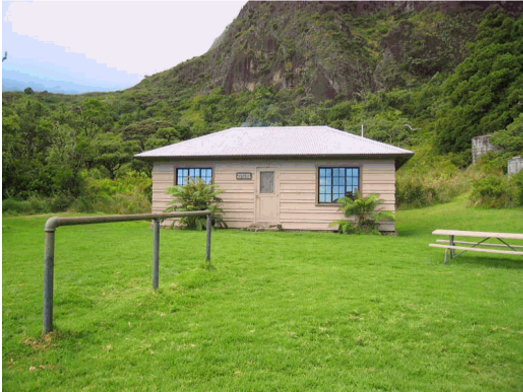
Buildings and Structures #3: The Paliku Patrol Cabin, located a short distance northeast of the Paliku Cabin in Haleakala Crater. Note the two water tanks situated on the slope behind the cabin (PWRO, 2008).
