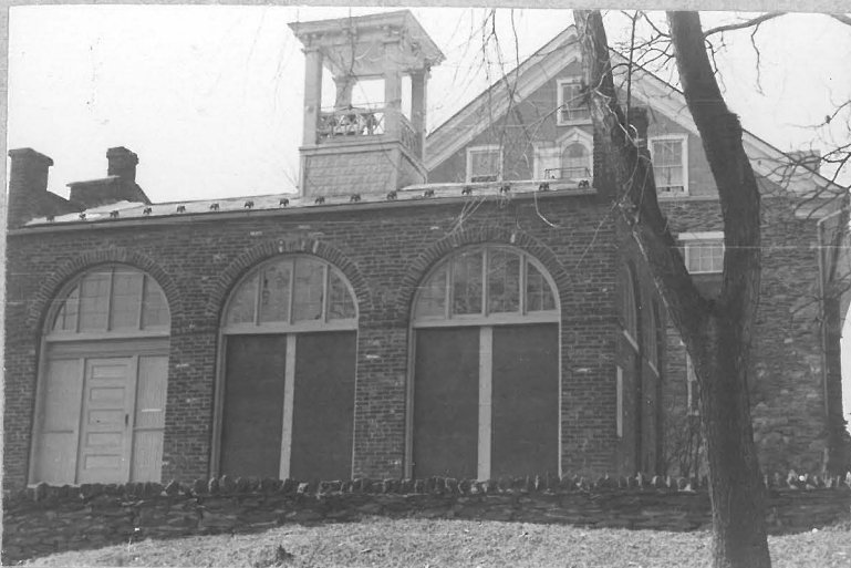
7. Side view of engine house.
