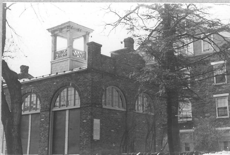
8. Corner view of engine house.
