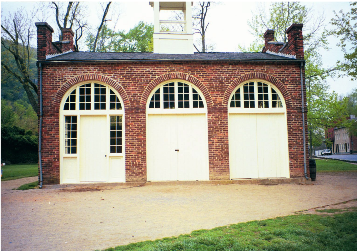
Photo 8: John Brown's Fort at close of project.
