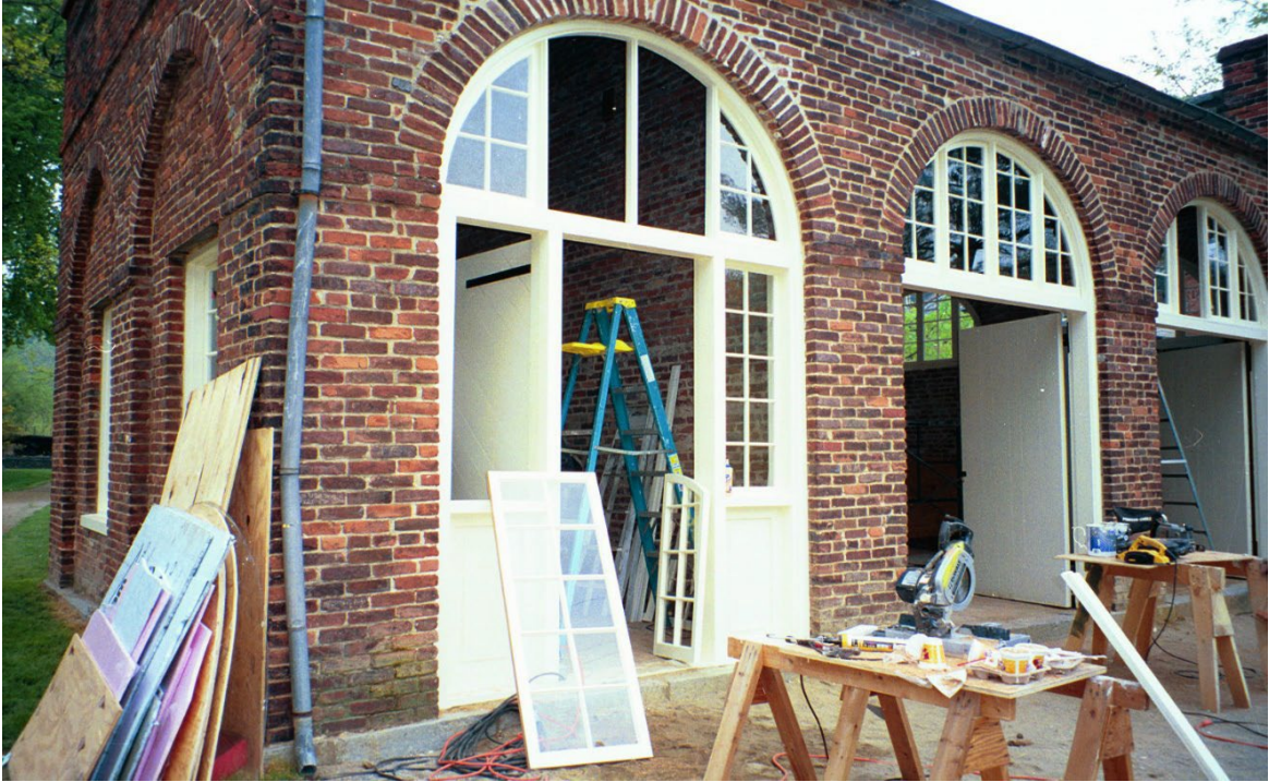
Photo 7: Installation of transom and side-lite sash.
