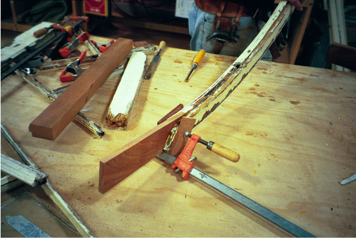
Photo 5: Dutchman repair of arched sash, using mahogany.
