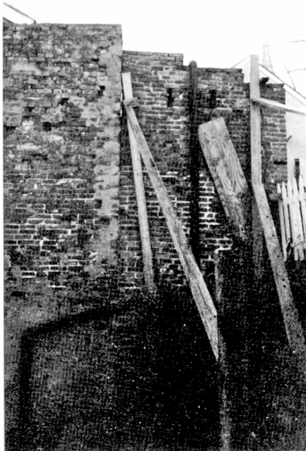
PHOTOGRAPH 19 (1980) Brick Addition to North Wall
