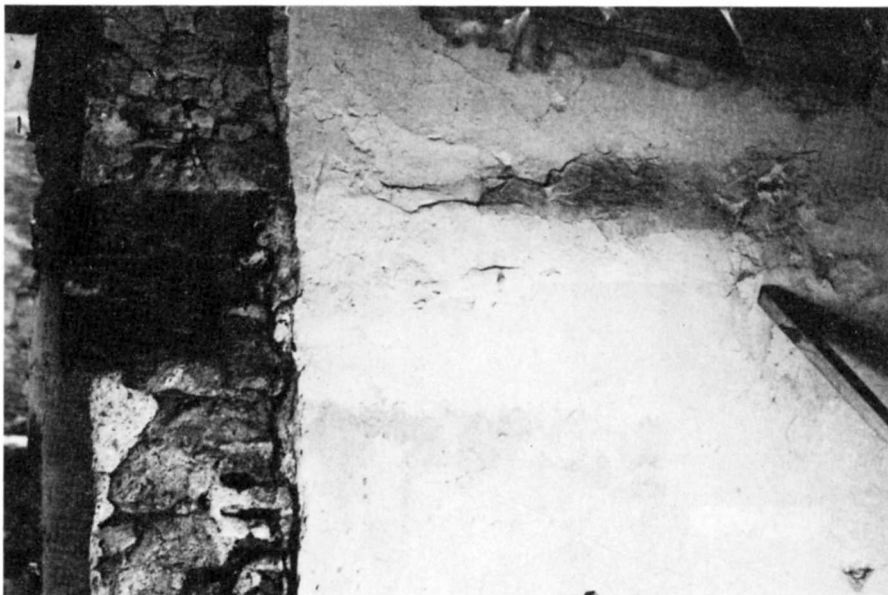
PHOTOGRAPH 43 (1981) Wood Lintel above Nonextant Window
