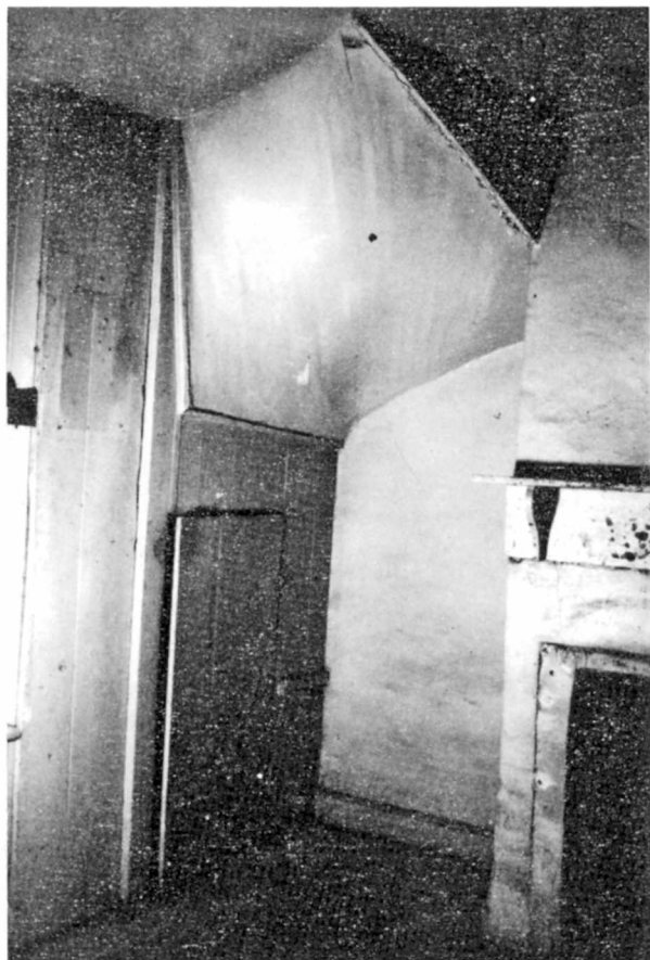
PHOTOGRAPH 69 (1981) Door 211, Closet Door under North Stairs
