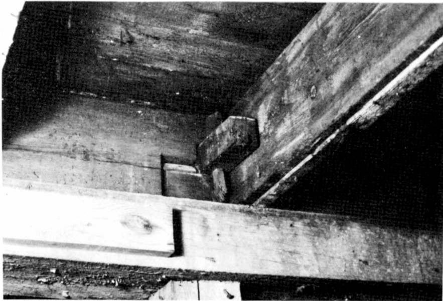
PHOTOGRAPH 47 (1981) Second-Floor Girder, Splice Detail
