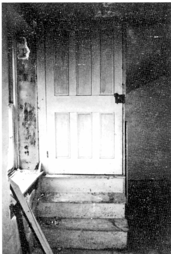
PHOTOGRAPH 70 (1981) Door 212 at North Stairs
