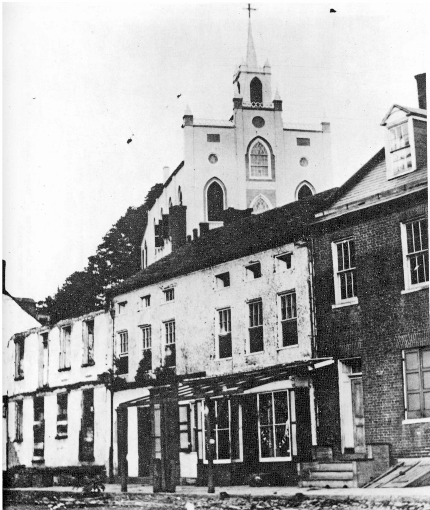
PHOTOGRAPH 3 (ca. 1865-1879) Building 38, Front or East Elevation
