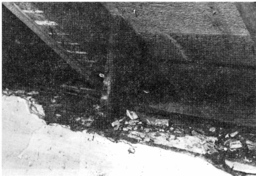
PHOTOGRAPH 53 (1981) Rafter End Brace
