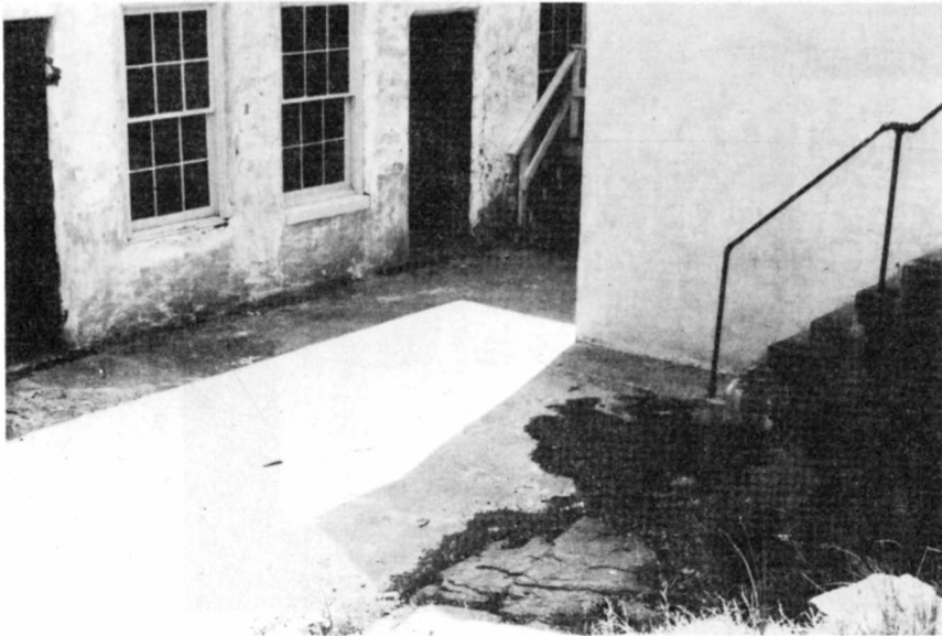
PHOTOGRAPH 23 (1977) Second-Level Concrete Porch
