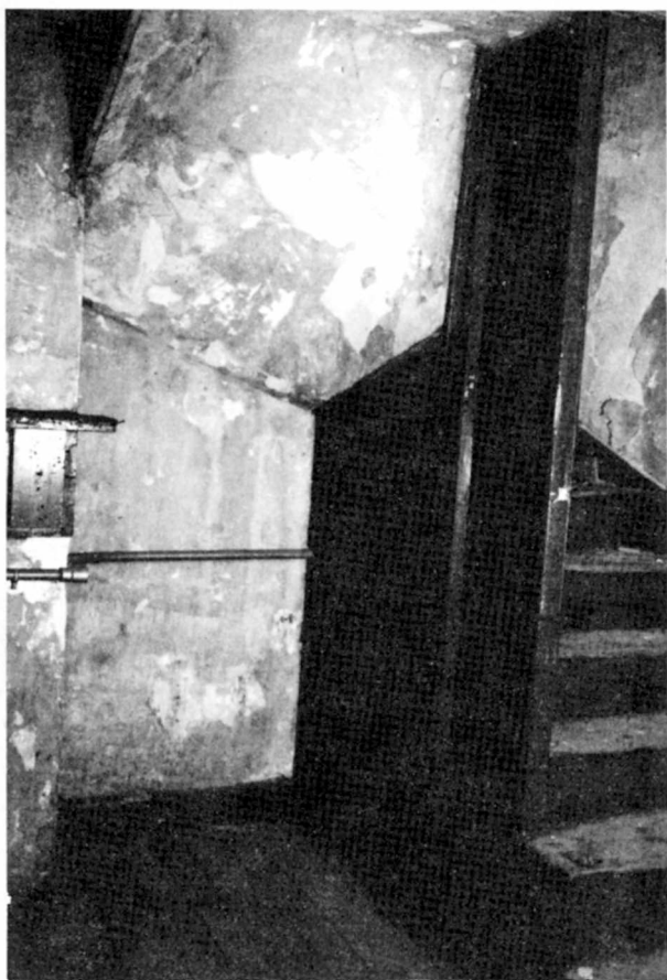
PHOTOGRAPH 66 (1981) Door 204, Clbset Door under South Stairs
