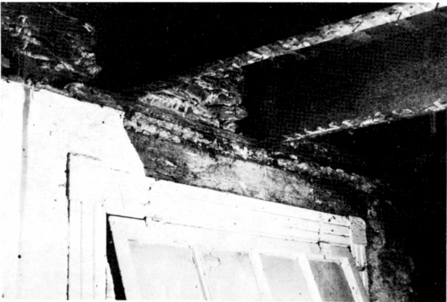
PHOTOGRAPH 48 (1981) Second-Floor Joists and Front Wall
