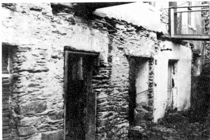
PHOTOGRAPH 39 (1980) Rear or West Elevation, First Floor
