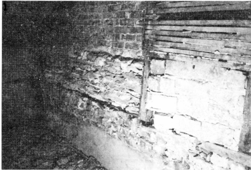
PHOTOGRAPH 54 (1981) South Wall, Room 302
