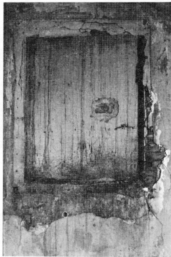
PHOTOGRAPH 55 (1981) Bricked-Up Window, South Wall of Room 301
