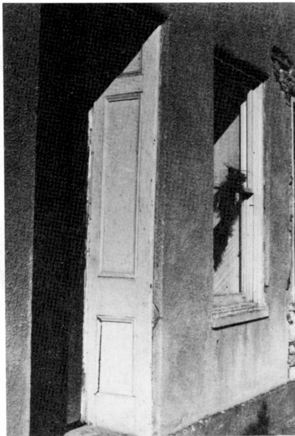
PHOTOGRAPH 37 (1980) Wooden Paneled Frame Reveal, Door 102
