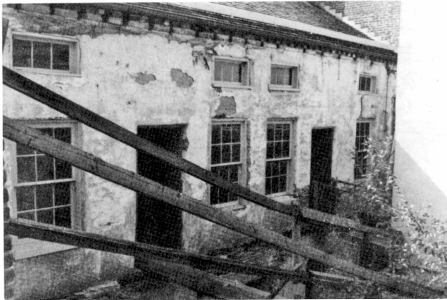
PHOTOGRAPH 38 (1981) Rear or West Elevation, Upper Floors
