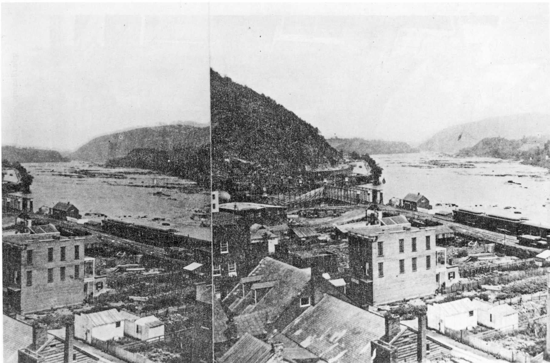
PHOTOGRAPH 4 (ca. 1877-79) Roof and South Gable of Building 38
