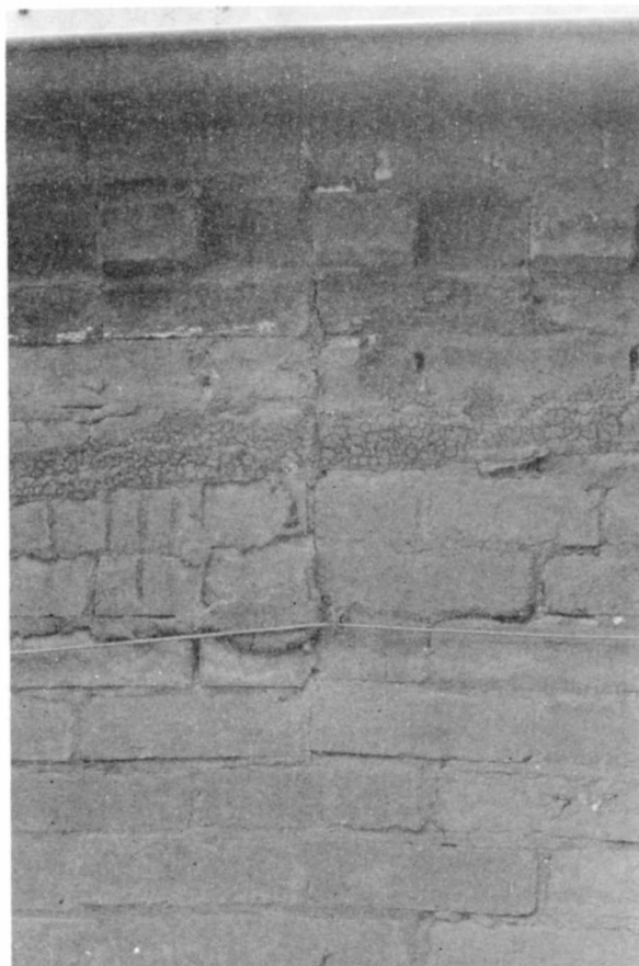
PHOTOGRAPH 16 (1980) South Elevation Near Roof Line
