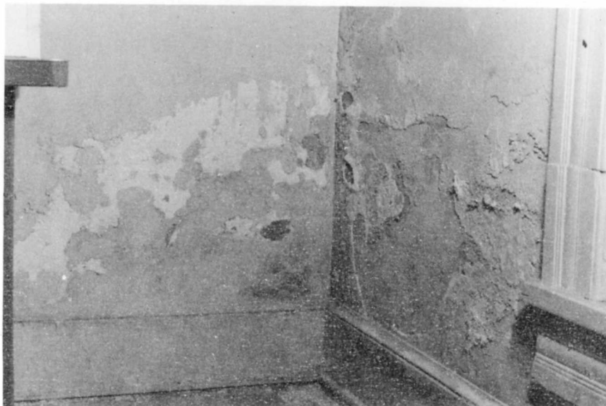
PHOTOGRAPH 29 (1980) Room 307, Southeast Corner
