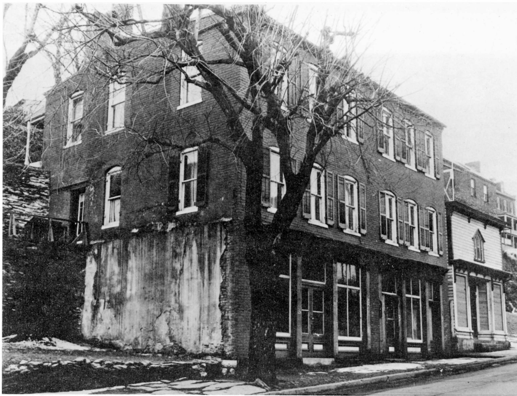
PHOTOGRAPH 55 (1955) Building 3, East and North Elevations
