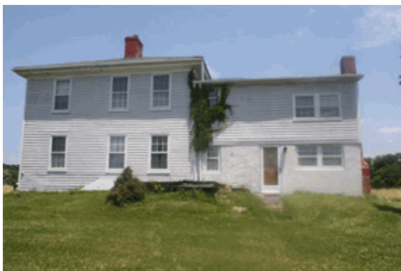
Figure 16: Photograph of the south side of the Chambers-Murphy farmhouse. the delineation between the older, eastern portion and the newer, western portion is easily visible. Note the covered cistern in the middle foreground.
