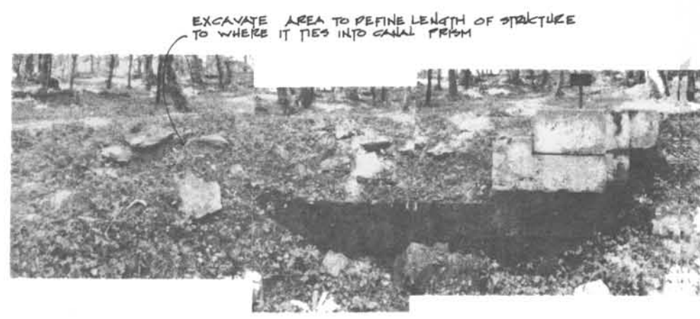
4 HEAD GATE - WEST ELEVATION 29 (PRIORITY 1E)
