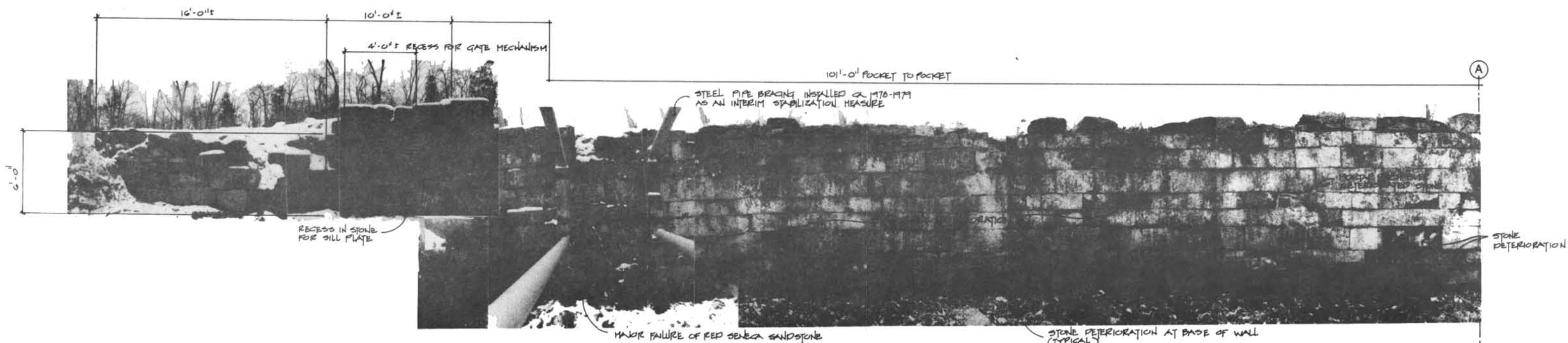
1 18 LOCK 1 - RIVER WALL AT NORTH END
