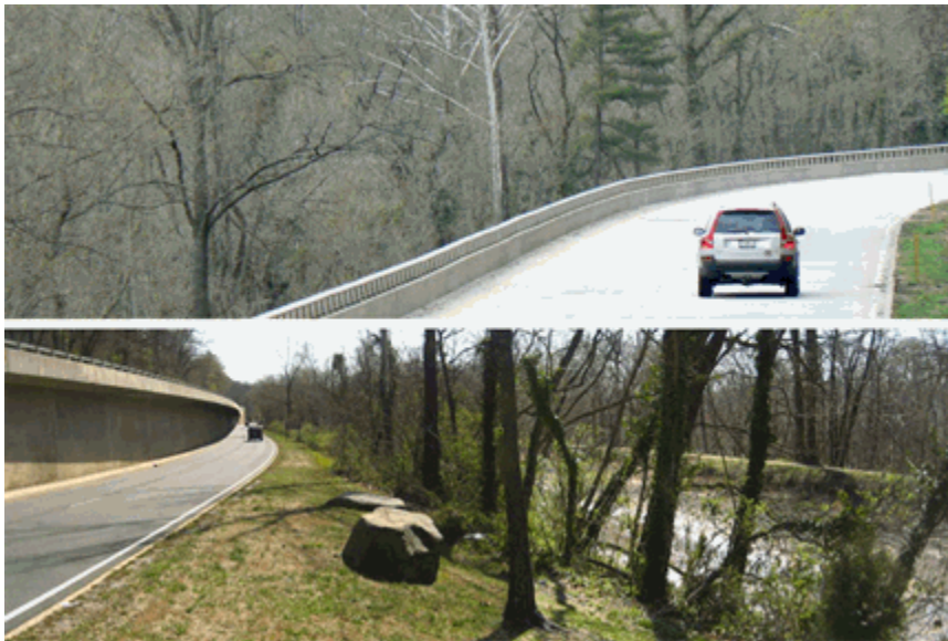
Cantilever. Top deck, westbound (top), lower level, eastbound (bottom) NPS-CLP 2012
