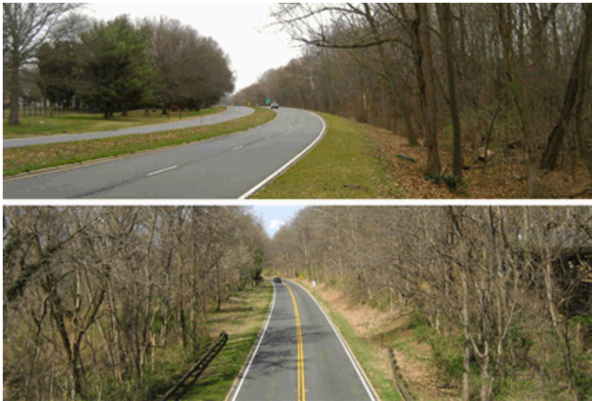
Opposite views from Brookmont pedestrian bridge. two-lane character at bottom.
