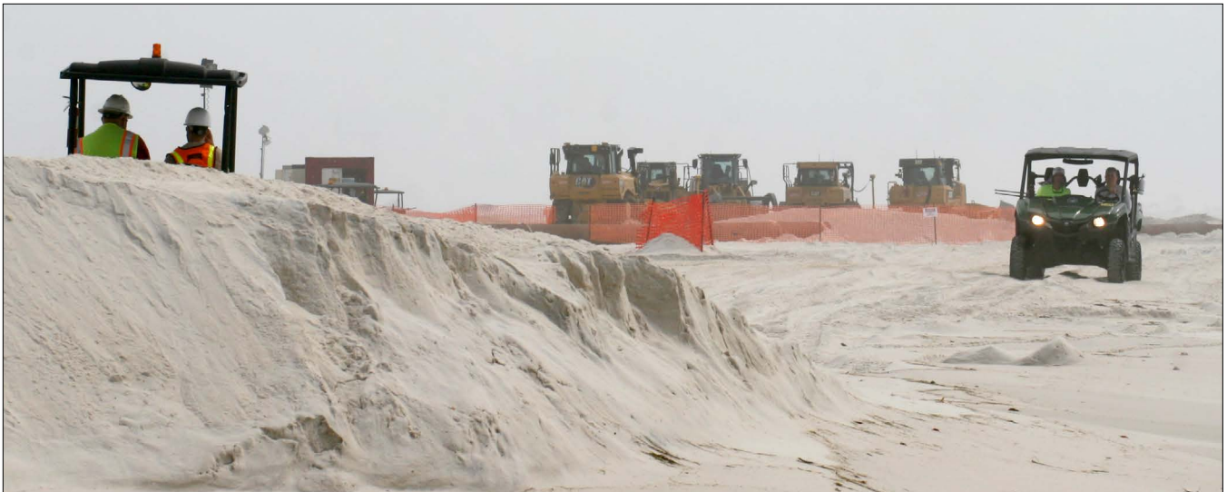
Figure 14. Heavy equipment and enclosure fencing associated with restoration work at Perdido Key.
