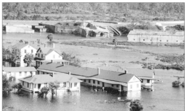
Fort Pickens Area historic structures were submerged in six feet of seawater for days.
