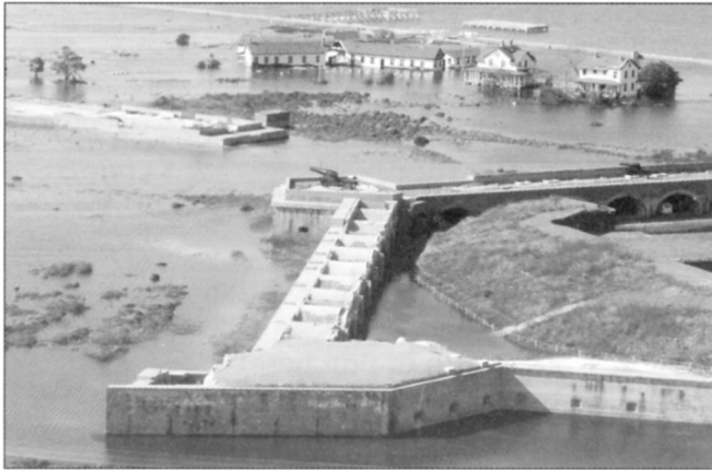
Fort Pickens sustained flooding damage, but this structure built from 1829-1834, with 21.5 million bricks, still stands. Pickens is part of an elaborate third system fortification constructed after the British devastated America's seaports in the War of 1812.
