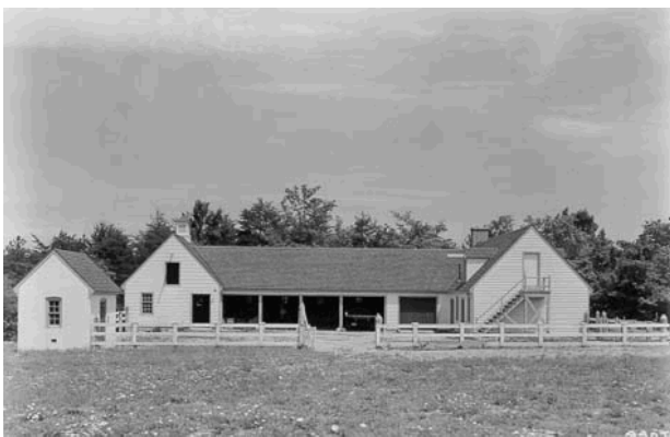
Utility Building and Inflammable Storage Unit, 1935
