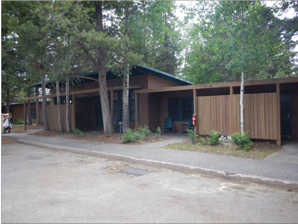
Photograph 2.6. Screening panels comprised of vertical wooden boards outside of room 531 (JL-324/529), facing southwest, 2014 (Source: Logan Simpson).
