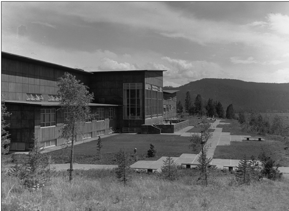
Figure 1.4. Western elevation of Jackson Lake Lodge, depicting the geometric concrete promenade with north and south terrace lawns, ca. 1960 (Source: GTLC Archives, Jackson Lake Lodge).
