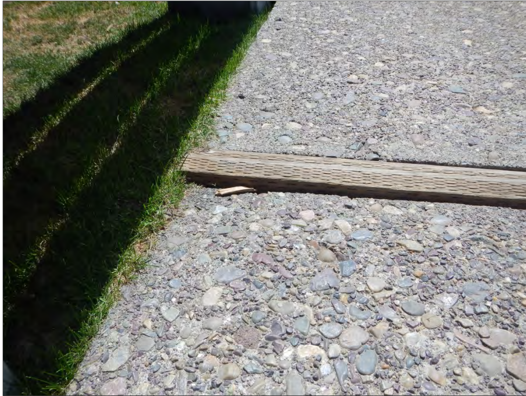
Photograph 2.14. Close-up of the promenade showing original wood band replaced with pressure treated lumber, facing south, 2014 (Source: Logan Simpson).
