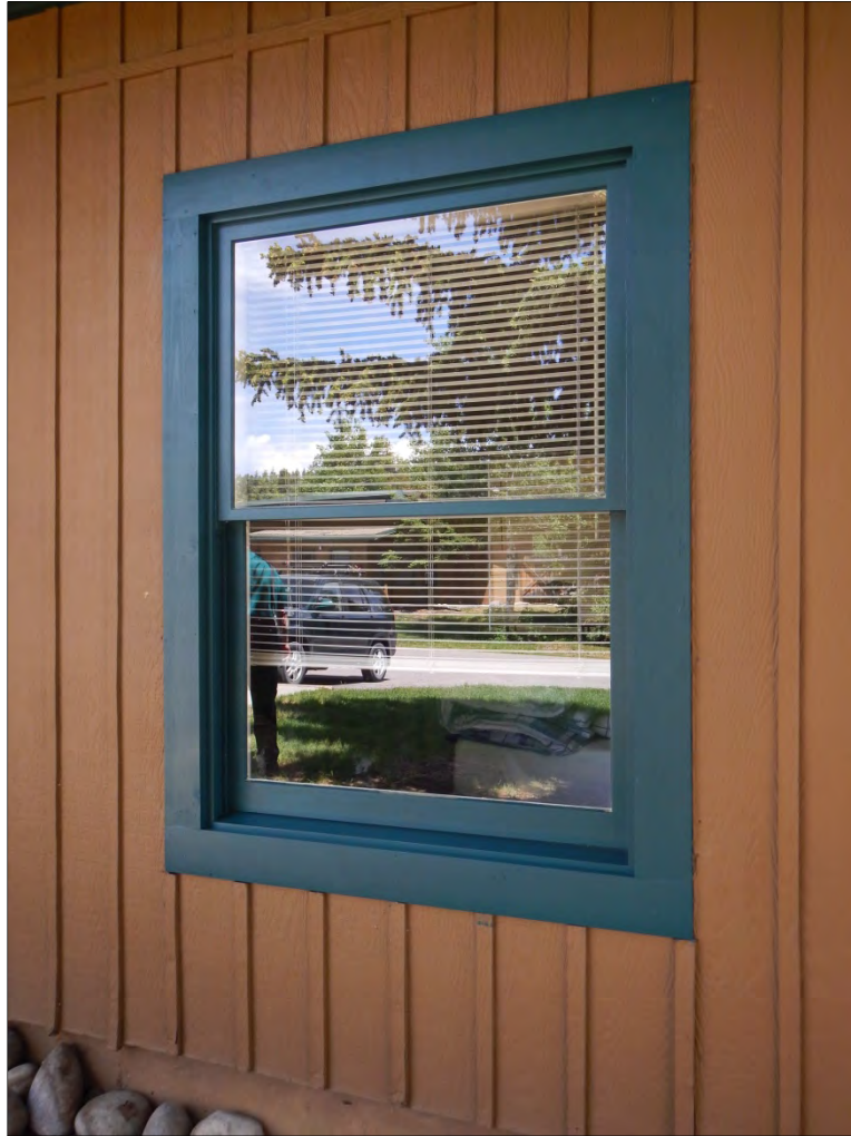
Photograph 2.9. Modern replacement window on Staff Housing no. 10 (JL-43) in the employee housing area, facing east, 2014 (Source: Logan Simpson).
