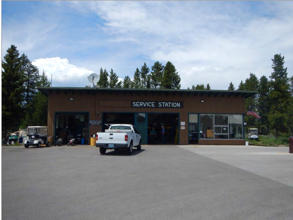
Photograph 2.10. Service station (JL-18), facing west, 2014 (Source: Logan Simpson).
