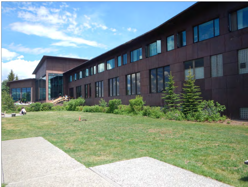
Photograph 2.2. Same view of the lodge, taken in 2014 (Source: Logan Simpson). Note the replacement windows and the northwestern Blue Heron Lounge addition.
