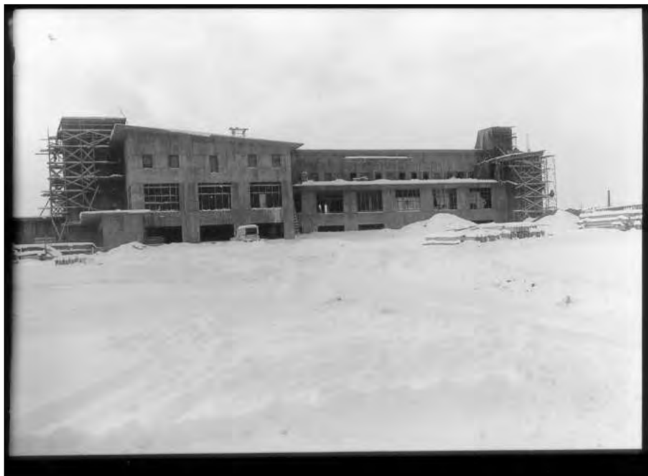
Figure 1.2. Eastern elevation of Jackson Lake Lodge, showing the initial construction, ca. 1954 (Source: GTLC Archives, Jackson Lake Lodge).
