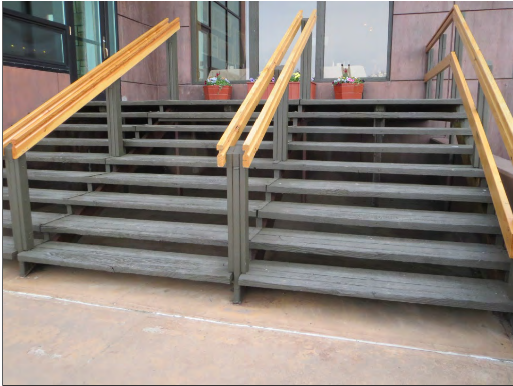
Photograph 2.3. Wooden stairway leading to the lodge's rear terrace, facing east, 2014 (Source: Paula Reed, Paula Reed & Associates Inc.).
