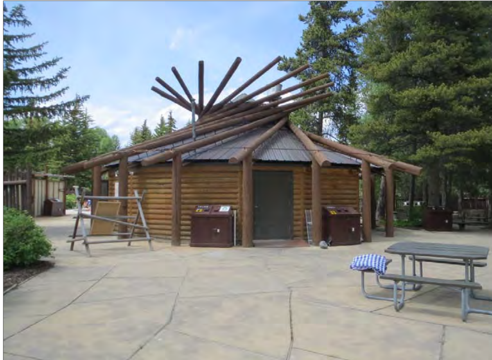
Photograph 1.4. Interior of the pool complex, showing the pool house (JL-21) (center) and maintenance shed (JL-21) (left center), facing east, 2014 (Source: Paula Reed, Paula S. Reed and Associates, Inc.).
