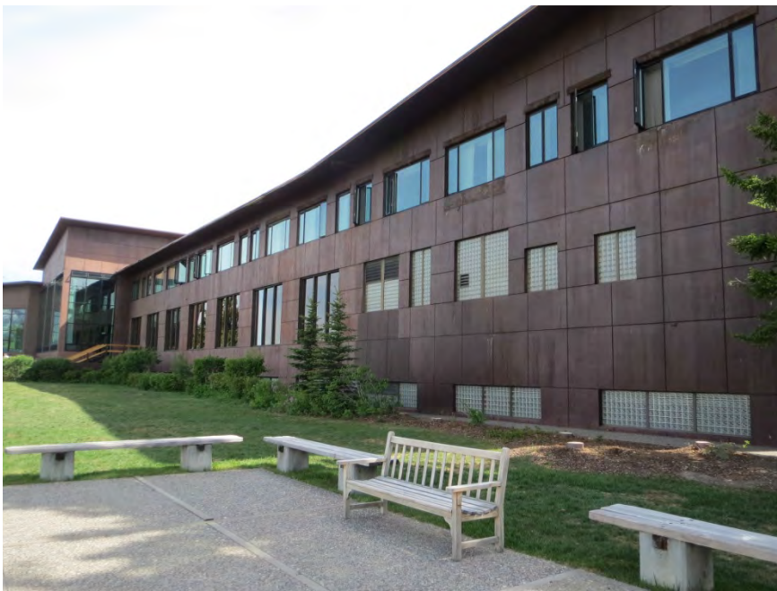
Photograph 4.3. Non-historic landscaping along the lodge's western foundation (Source: Logan Simpson).
