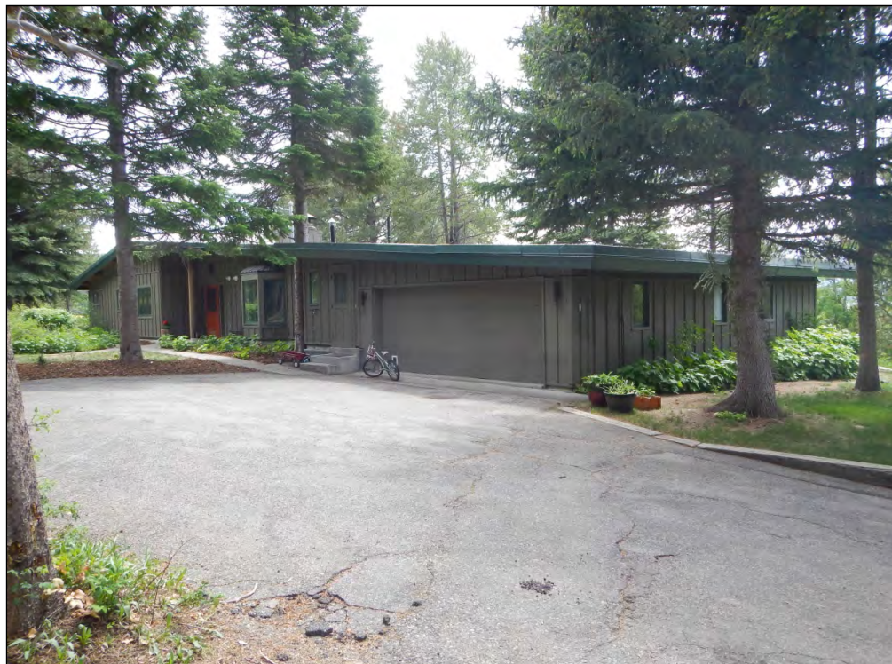
Photograph 1.5. Eastern and northern facades of the manager's residence, facing southwest, 2014 (Source: Logan Simpson).
