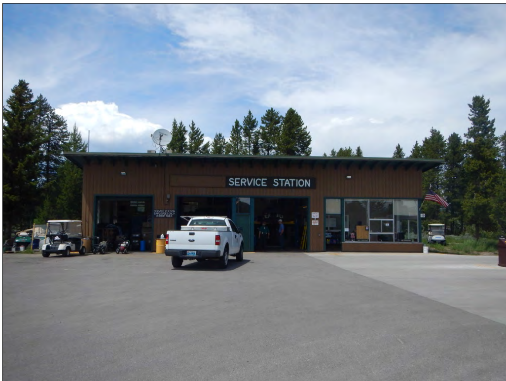
Photograph 1.8. Service station (JL-18), facing west, 2014 (Source: Logan Simpson).
