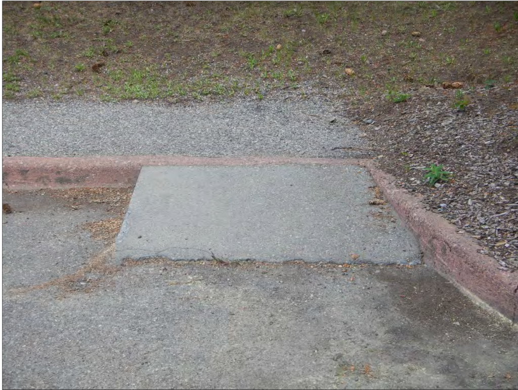
Photograph 2.12. Concrete ramp in the south guest cottage area, facing east, 2014 (Source: Logan Simpson).
