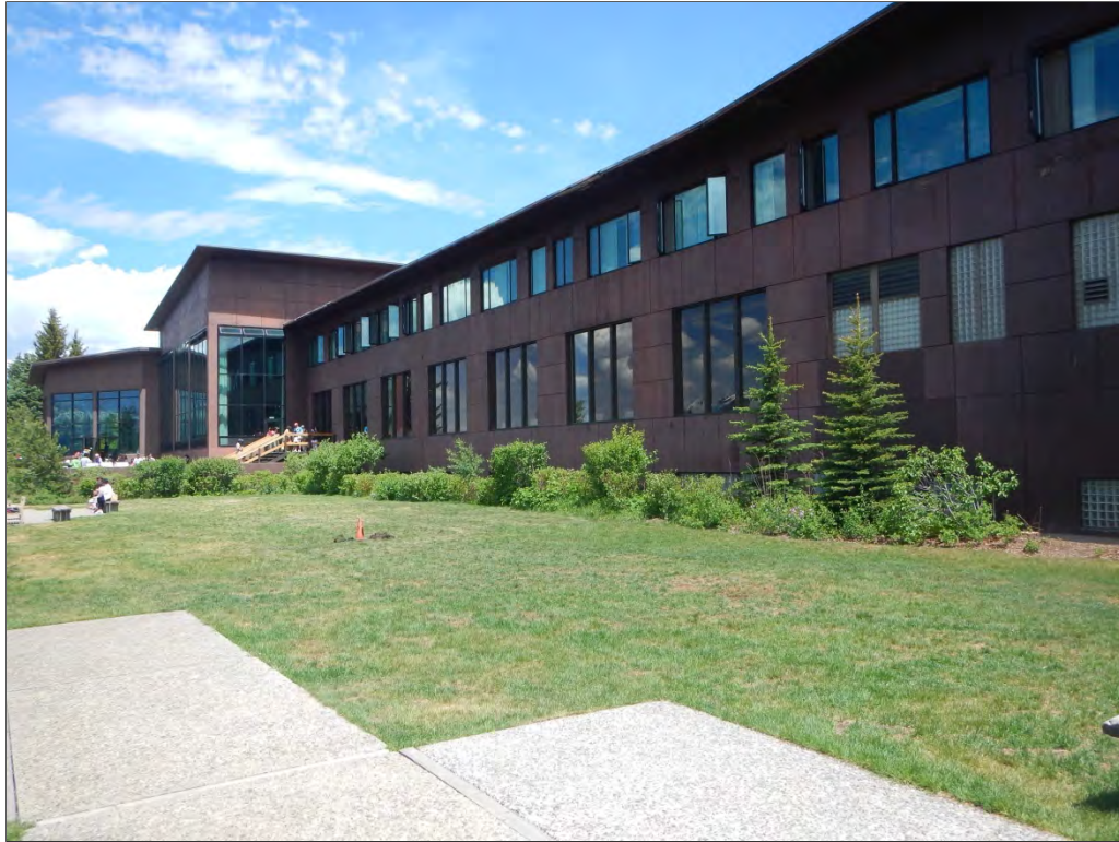
Photograph 1.1. Western façade of the lodge, facing northeast, 2014 (Source: Logan Simpson).
