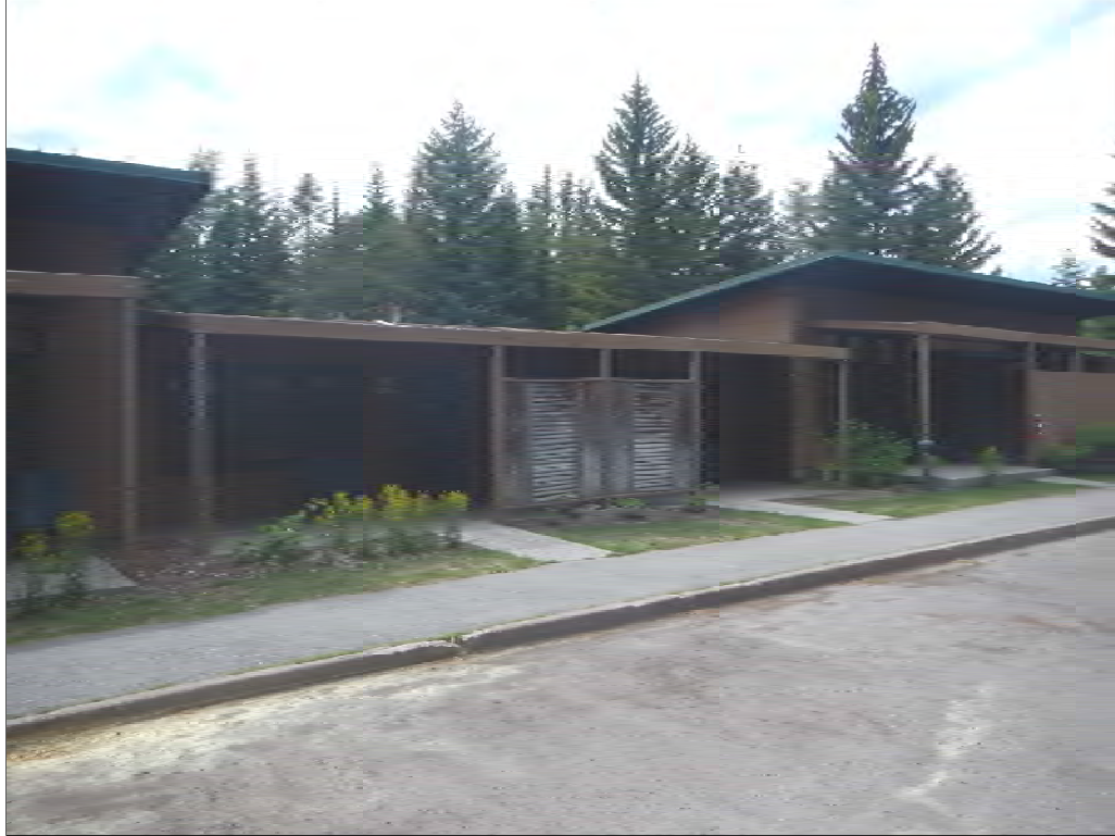
Photograph 2.4. Combined vertical and horizontal lodgepole pine screening panels outside of rooms 304-309 (JL-9), facing west-northwest, 2014 (Source: Logan Simpson).
