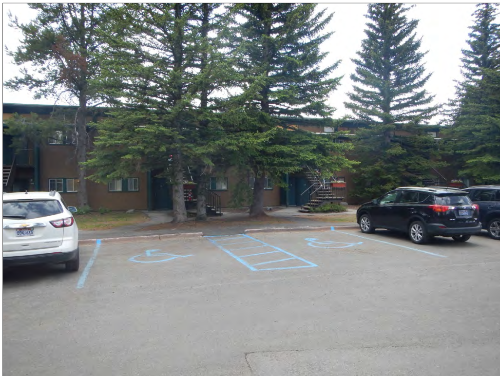
Photograph 2.18. Curb cut to create ADA accessible ramp in front of rooms 560–579 in the south guest cottage area, facing southwest, 2014 (Source: Logan Simpson).
