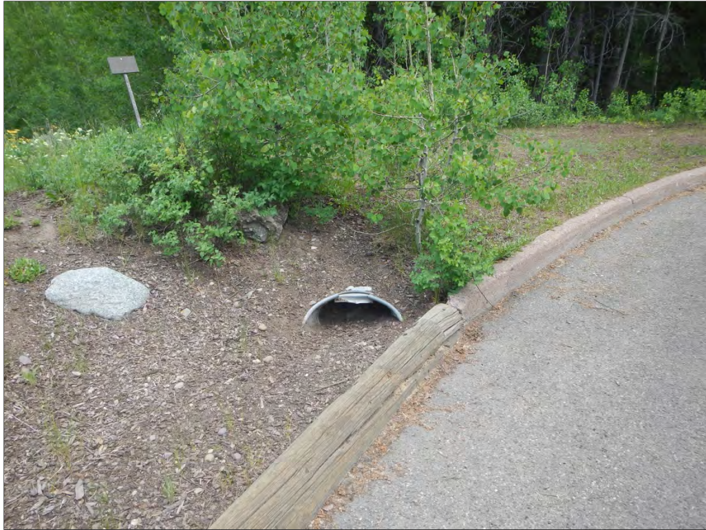
Photograph 2.17. Replacement of concrete at the southern end of the south guest cottage area with wooden logs, southeast, 2014 (Source: Logan Simpson).
