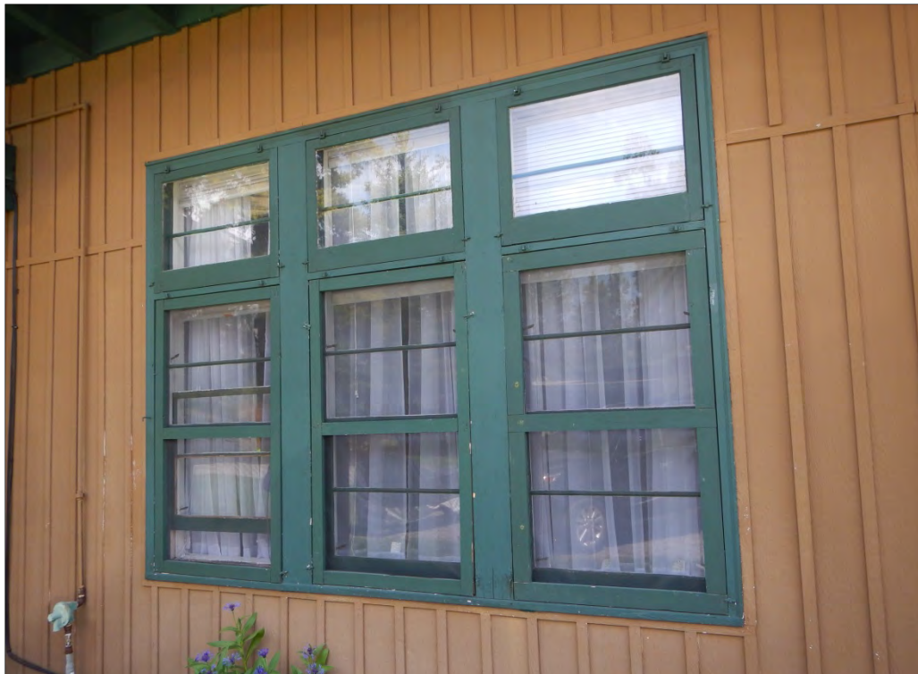
Photograph 2.8. Original wood frame windows on Staff Housing no. 8 (JL-42) in the employee housing area, facing east, 2014 (Source: Logan Simpson).
