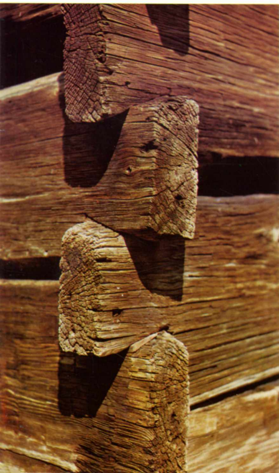
Chamfer and Notch Joint
