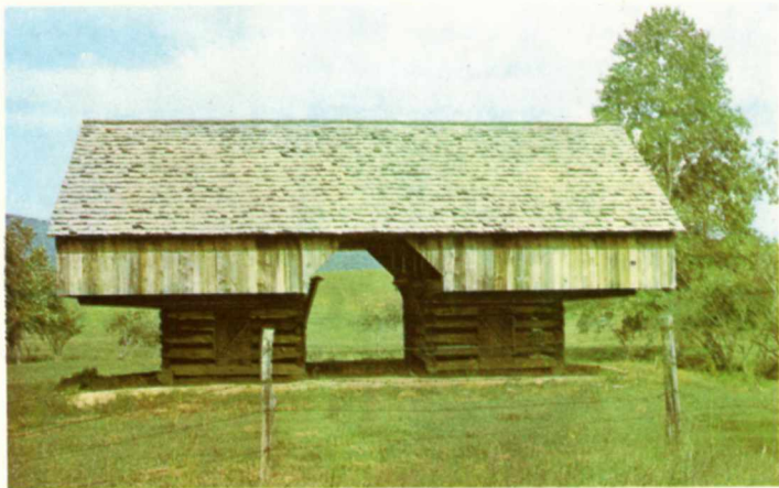
Cantilevered Barn—Tipton Oliver Place
