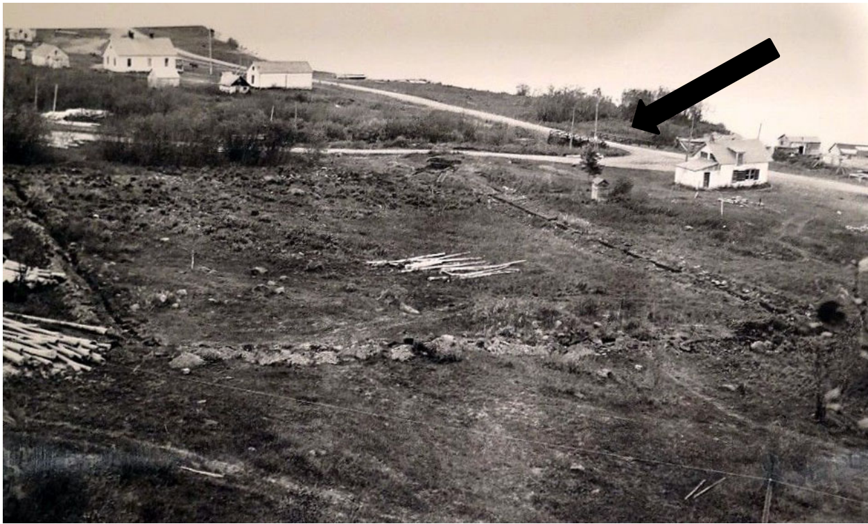
Figure 2: View of original road and bridge, marked by arrow. Courtesy of Grand Portage Museum, Mary Ann Gagnon.
