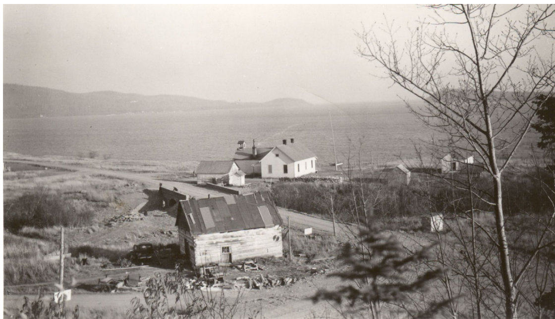
Figure 3: Completed road and bridge. Courtesy of Grand Portage National Monument.
