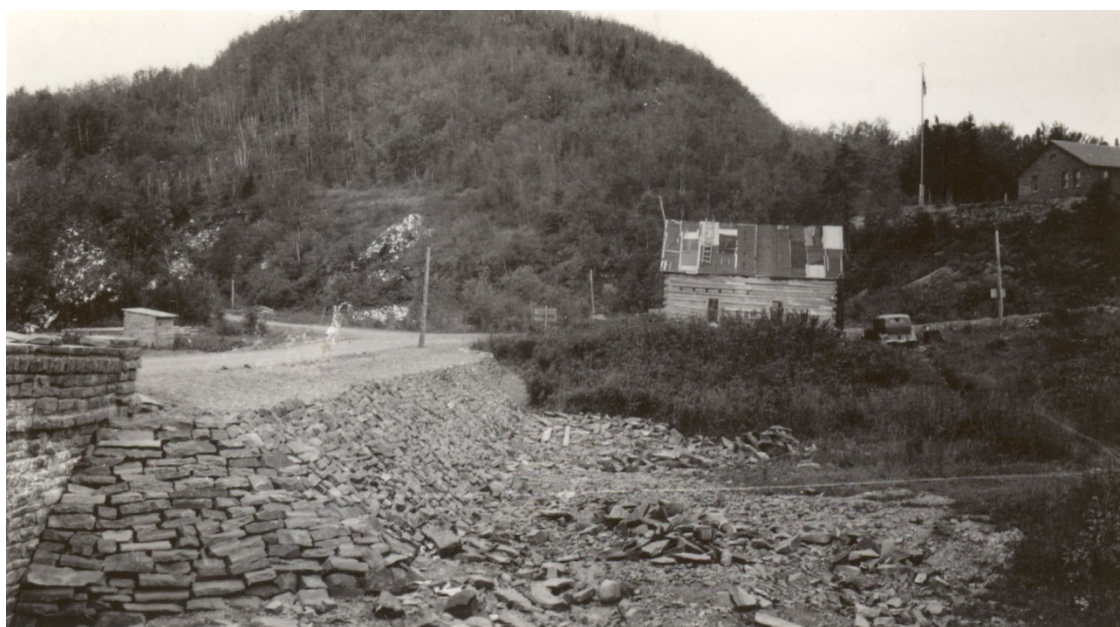
Figure 4: View of stonework on bank, some of which is still visible. Courtesy of Grand Portage National Monument.
