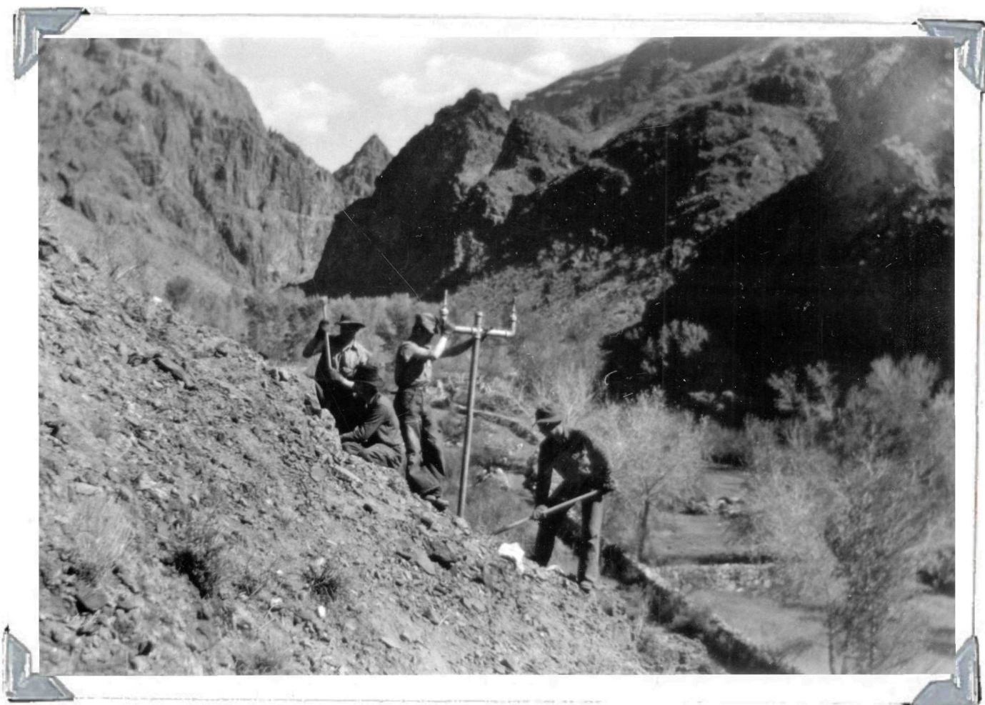
Figure 8. CCC workers installing the line north of Phantom Ranch.
