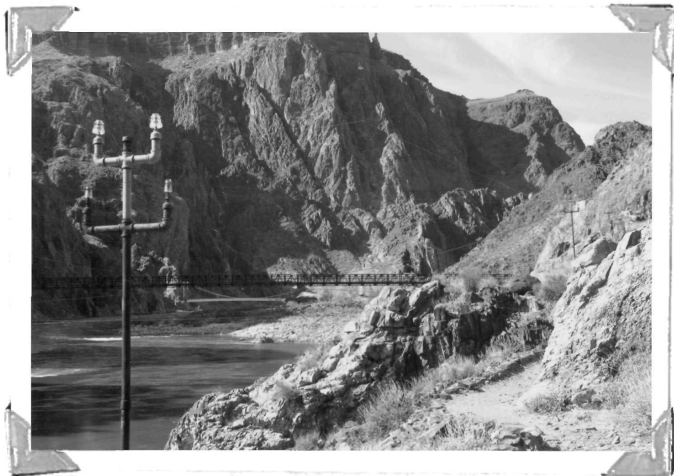
Figure 4. The trans-canyon telephone line at the Colorado River.
