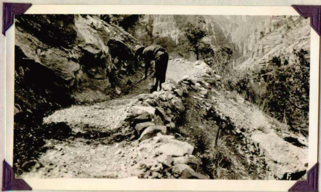
Maintainer repairing damaged wall on the Kaibab Trail in the Bright Angel Creek "Box".
