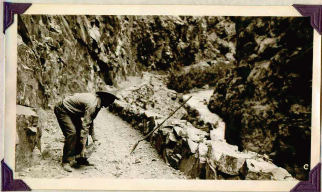
Maintainer repairing damaged wall on the Kaibab Trail in the Bright Angel Creek "Box".
