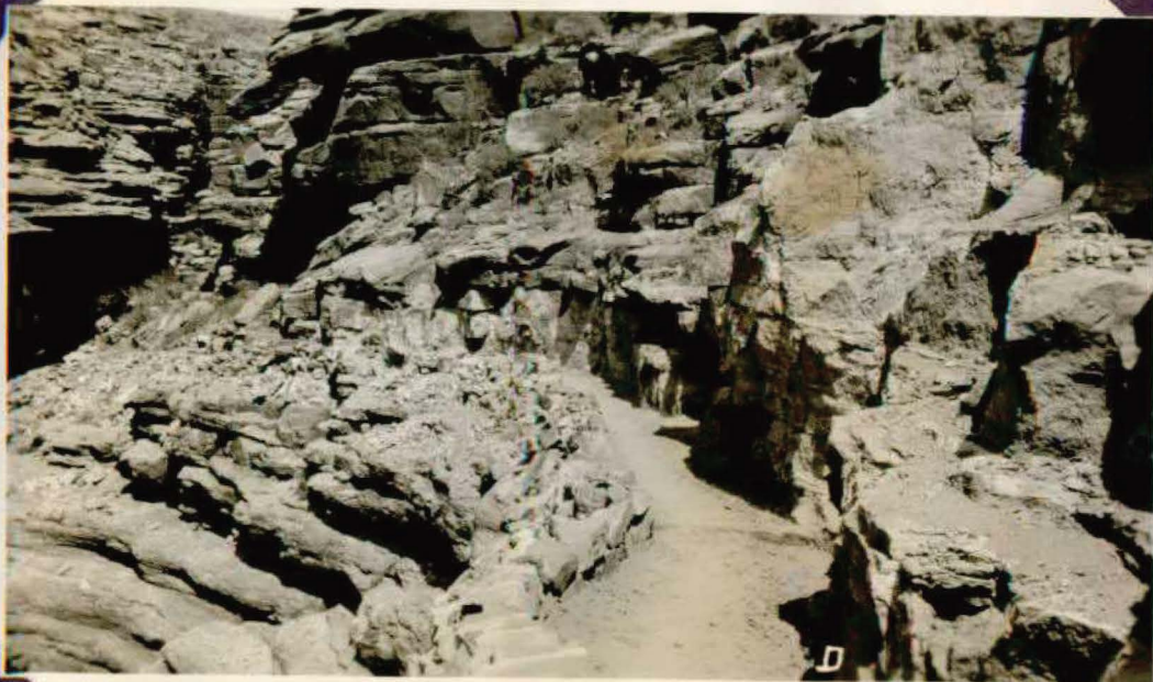
A section of the Bright Angel Trail below Indian Gardens. Note water break in foreground.
