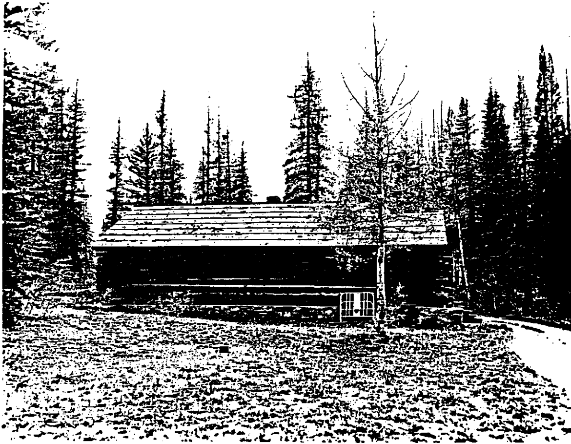
Figure 14. GCNP Building #122, formerly the north rim entrance station toll collector's residence, later used by miscellaneous park forces. This photo taken in June 1949. (GRCA Image #1768, GCSC)
