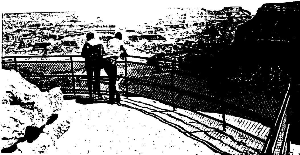
Figure 22. 1962 modifications: New guardrail and chain link fencing at Trailview pullout.
