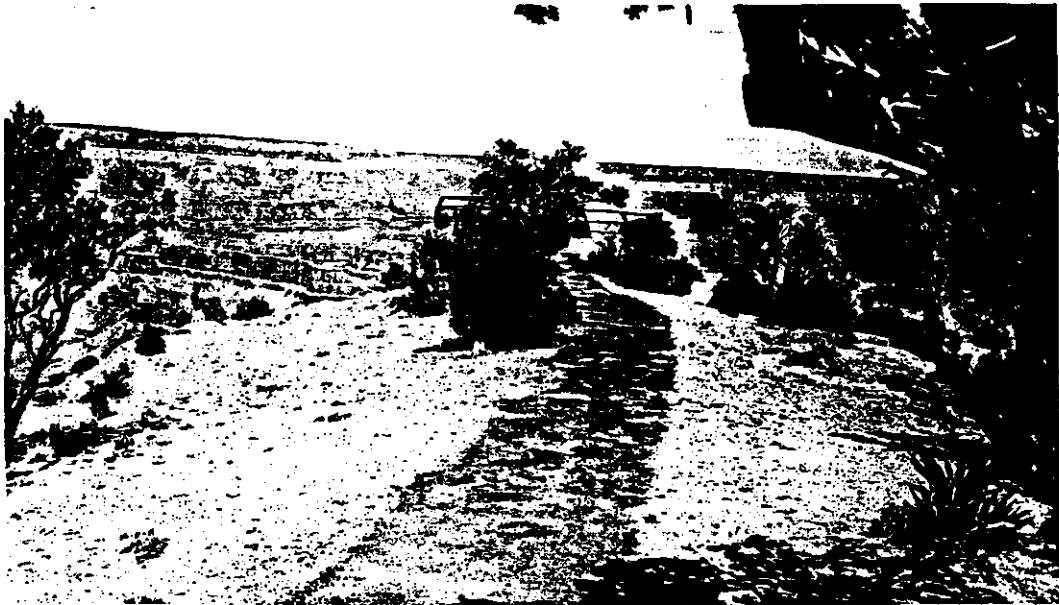
Figure 20. 1962 modifications: Bituminous walk leading to Maricopa Point viewpoint.
