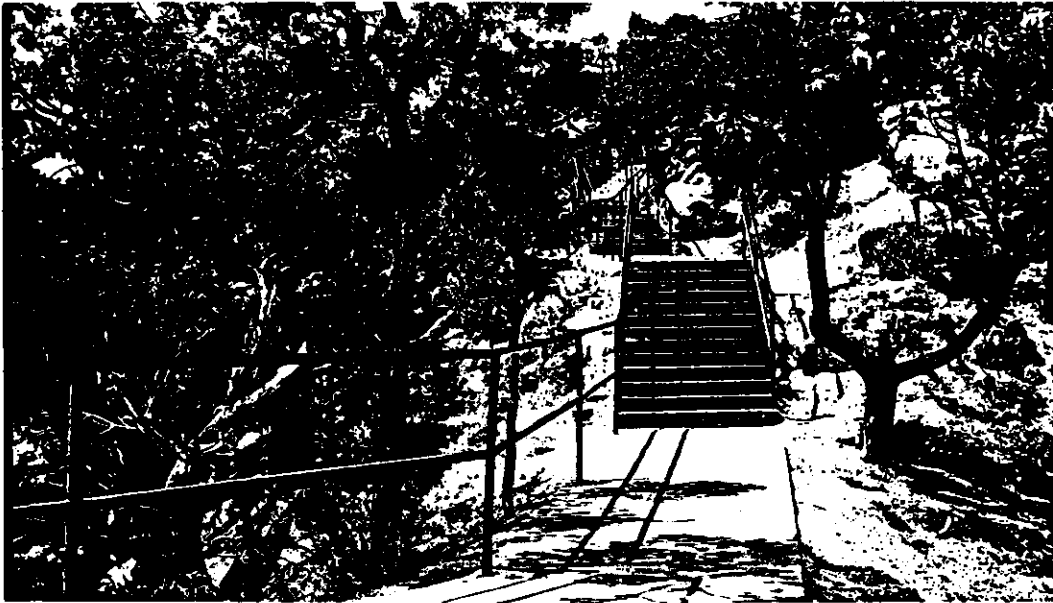
Figure 23. 1962 modifications: Lower level concrete walk, steps, and pipe handrail at Trailview Point.
