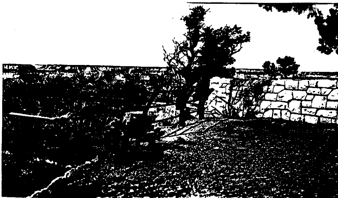
Figure 18. Fine masonry wall beside pedestrian guardrails at a pullout, 1935. (GRCA Image #8873, GCSC)
