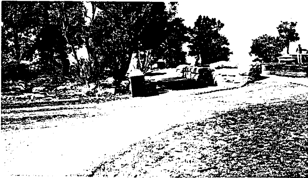
Figure 19. 1962 modifications: Bituminous walk with masonry curb and wall (background) at Hermits Rest. (From completion report, GRCA 61773, Box 6, GCSC; all following photos from same report)
