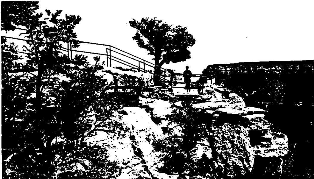
1962 modifications: Lower level concrete walk, steps, and pipe handrail at Trailview Point.
