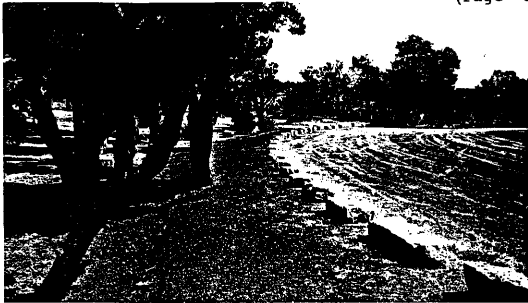
Figure 21. 1962 modifications: Bituminous walk behind rock curbing at Maricopa Point parking loop.
