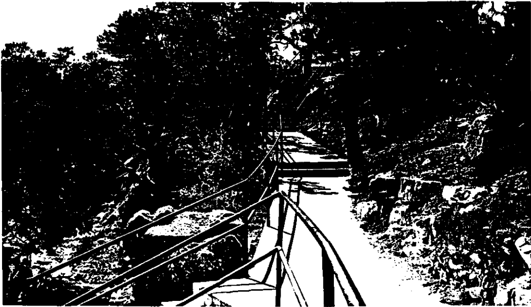
Figure 25. 1962 modifications: Upper level concrete walk, steps, and pipe handrail at Trailview Point.
