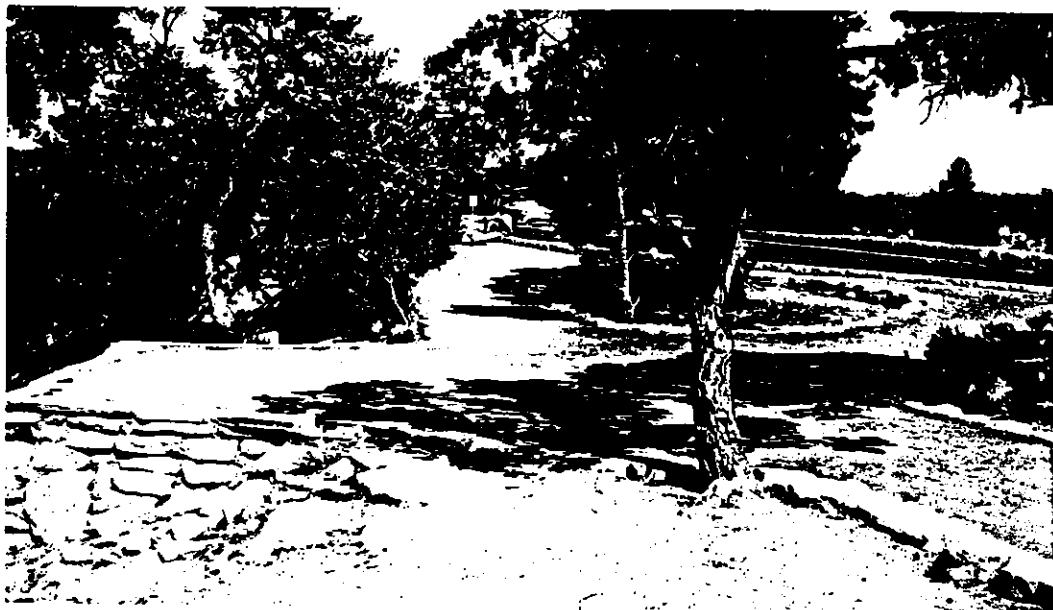
1962 modifications: Bituminous walk with masonry curbing at Hermits Rest.
