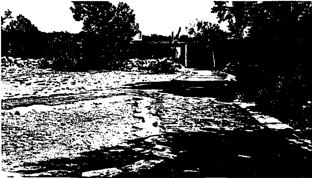
1962 modifications: Bituminous walk with masonry curb leading to "comfort station" at Hermits Rest.
