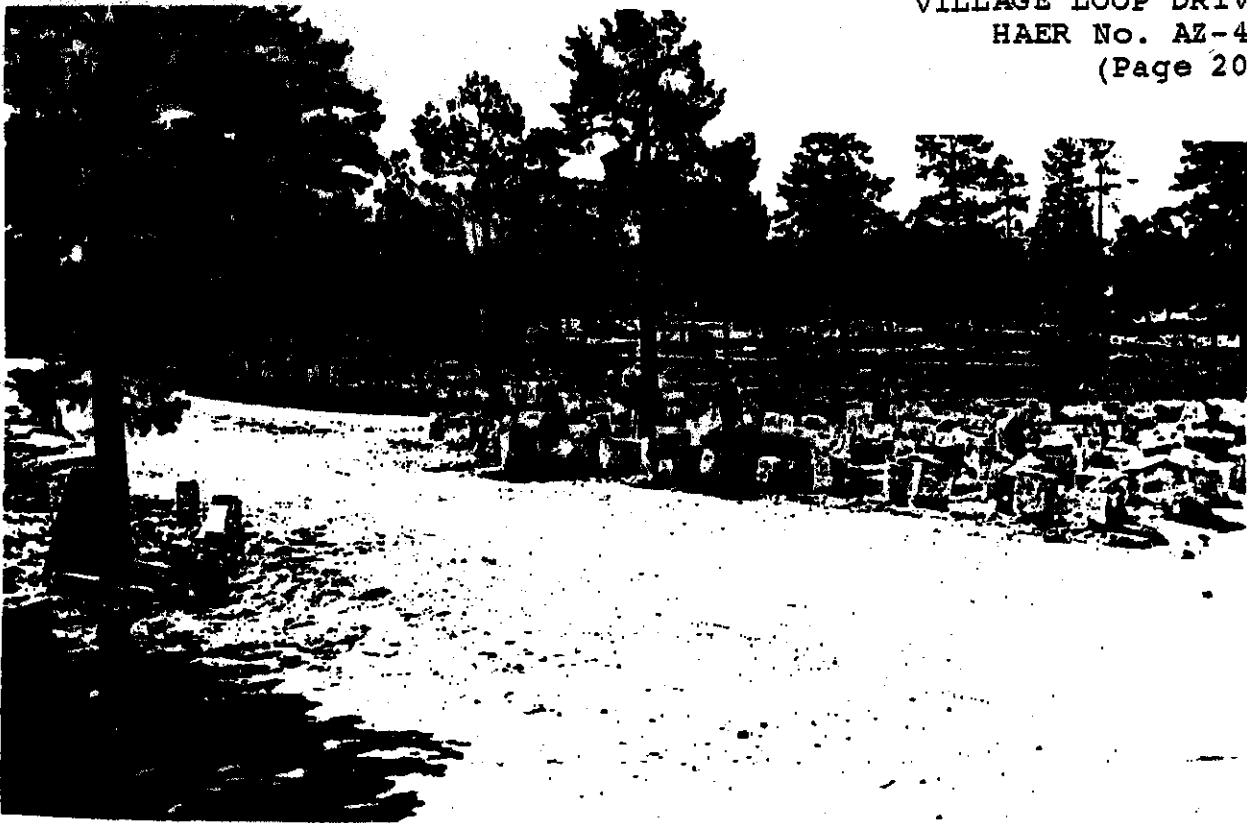
Figure 11. Village Loop construction at Station 26, facing southeast from the first pullout of West Rim Drive, 1935. Masons working on walls and curbs. (GRCA Image #2981, GCSC)
