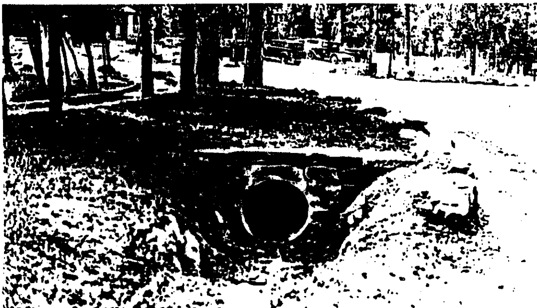
Figure 17-18. Construction of culvert headwall on the southeast corner of Village Loop and Center Road, September 1934. This headwall is being replaced in 1994 construction project. (CCC Reports photo, GCSC)
