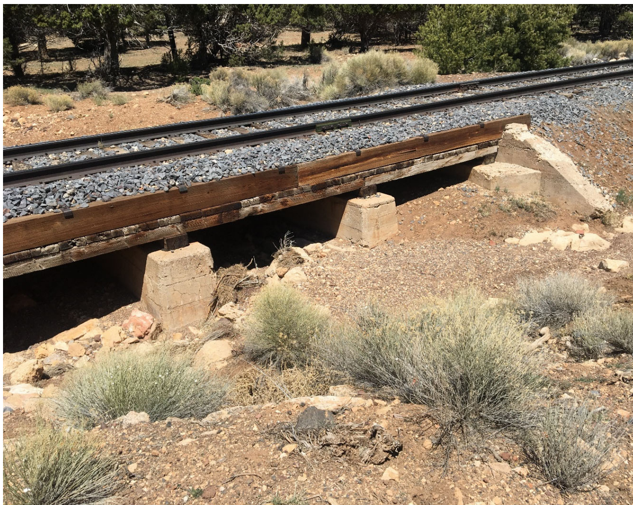
Figure 19. Bridge No. 79 (B-64), a 28'-4"-long ballast deck bridge located at Milepost 63.2. David Vago photo, April 2022.
