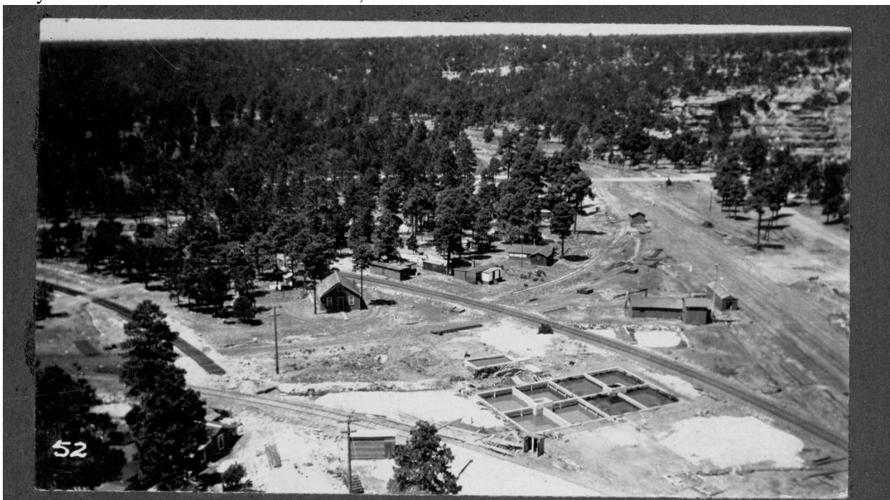
Figures 7-8. Ballast laid by contractor W.J. Burton for the new north wye prior to the box culvert being constructed across Bright Angel Wash. The ballast at left is for the new powerplant wye. M.E.J. Colter photo, Grand Canyon National Park Museum Collection, GRCA 13641. Below: Similar view from the chimney top of the new powerhouse showing newly laid track of the north wye. Although outside the frame, Bridge No. 82 would have been erected by this date, Aug. 18, 1926. James L. Morris photo, Grand Canyon National Park Museum Collection, GRCA 61004.
