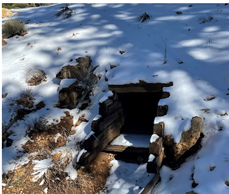
Figure 18. 3' x 3'-1" x 78'-4" wooden box culvert built in 1926 located at tail of wye. David Vago photo, March 2022.
