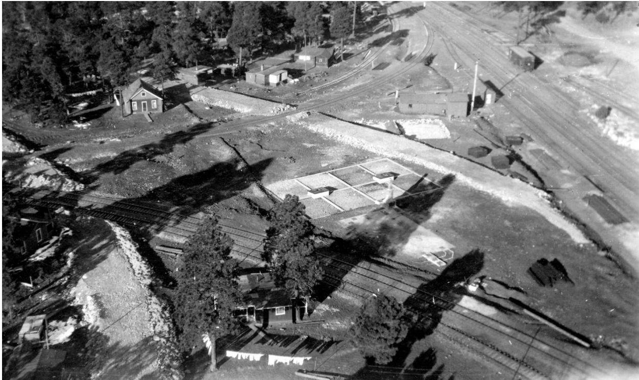
Figures 7-8. Ballast laid by contractor W.J. Burton for the new north wye prior to the box culvert being constructed across Bright Angel Wash. The ballast at left is for the new powerplant wye. M.E.J. Colter photo, Grand Canyon National Park Museum Collection, GRCA 13641. Below: Similar view from the chimney top of the new powerhouse showing newly laid track of the north wye. Although outside the frame, Bridge No. 82 would have been erected by this date, Aug. 18, 1926. James L. Morris photo, Grand Canyon National Park Museum Collection, GRCA 61004.
