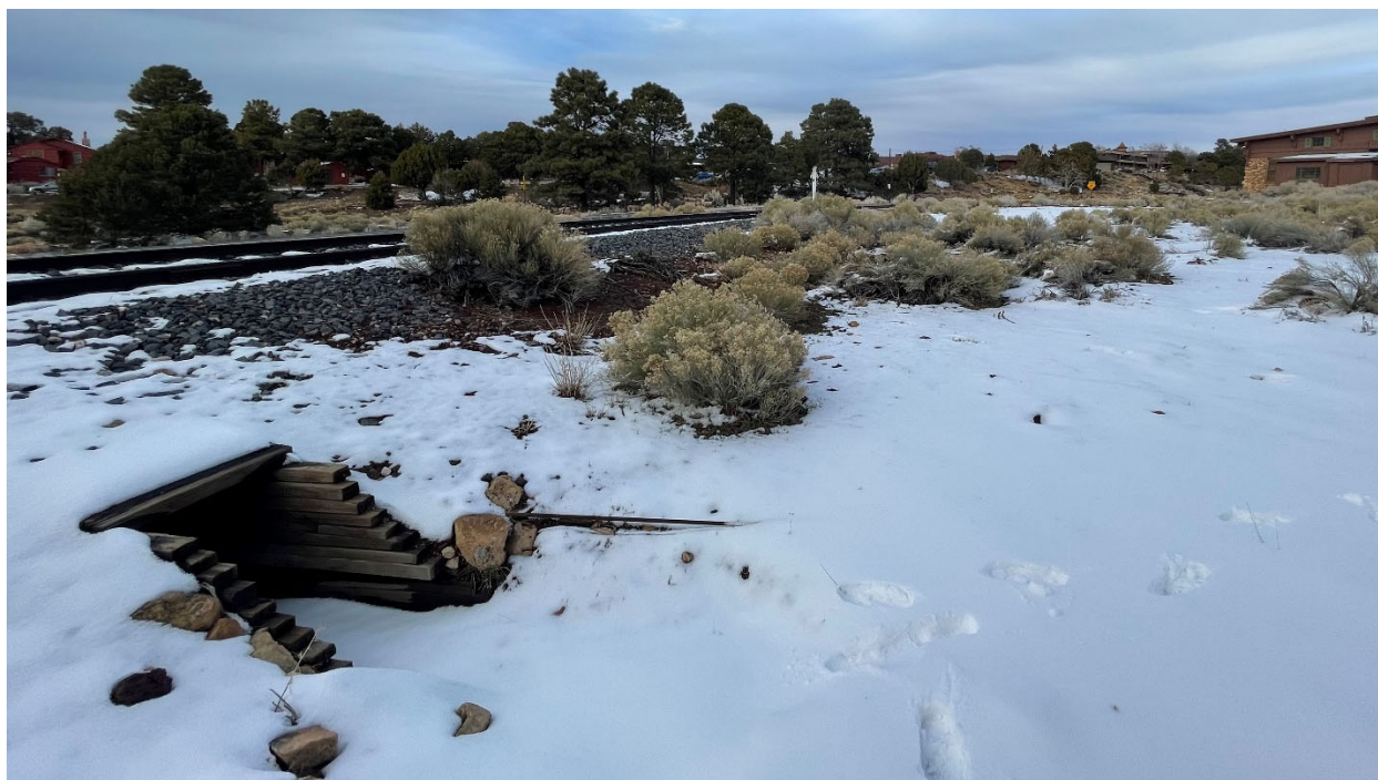
Figure 17. 2' x 2'-2" x 33'-2" wooden box culvert beneath north leg of wye with the laundry in the distance. David Vago photo, March 2022.
