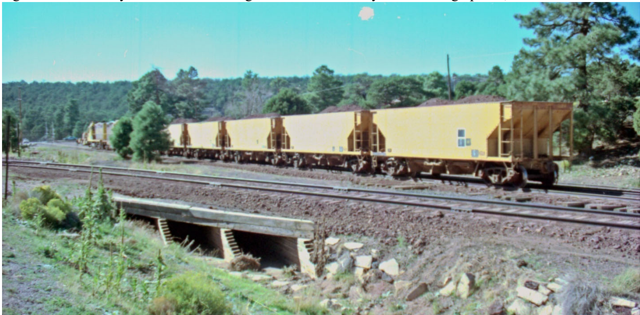
Figure 15. View of Bridge No. 82 looking west with loaded gondolas in the background, ca. 1985-89. Grand Canyon National Park Museum Collection, # C-0951.
