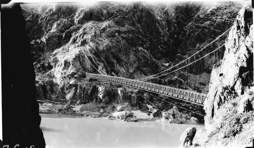
1. View of completed bridge looking toward North Abutment.
