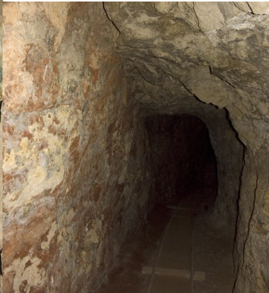
PIC-10: 7 th level fissure #6
