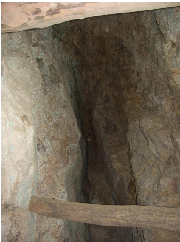
PIC-12: Looking up at main fissure #3 on 4 th level
