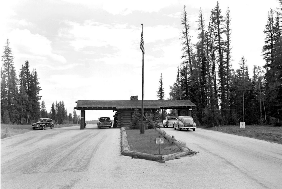
Entrance Road from South looking North, 1930. (Source: North Rim Developed Area Cultural Landscape Report, 2004).
