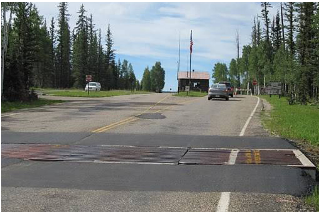
Entrance Station, displaying the curbed asphalt-paved parking lot to the left and the cattle guard in the forefront. Photograph by Meaghan Heisinger, August 2010
