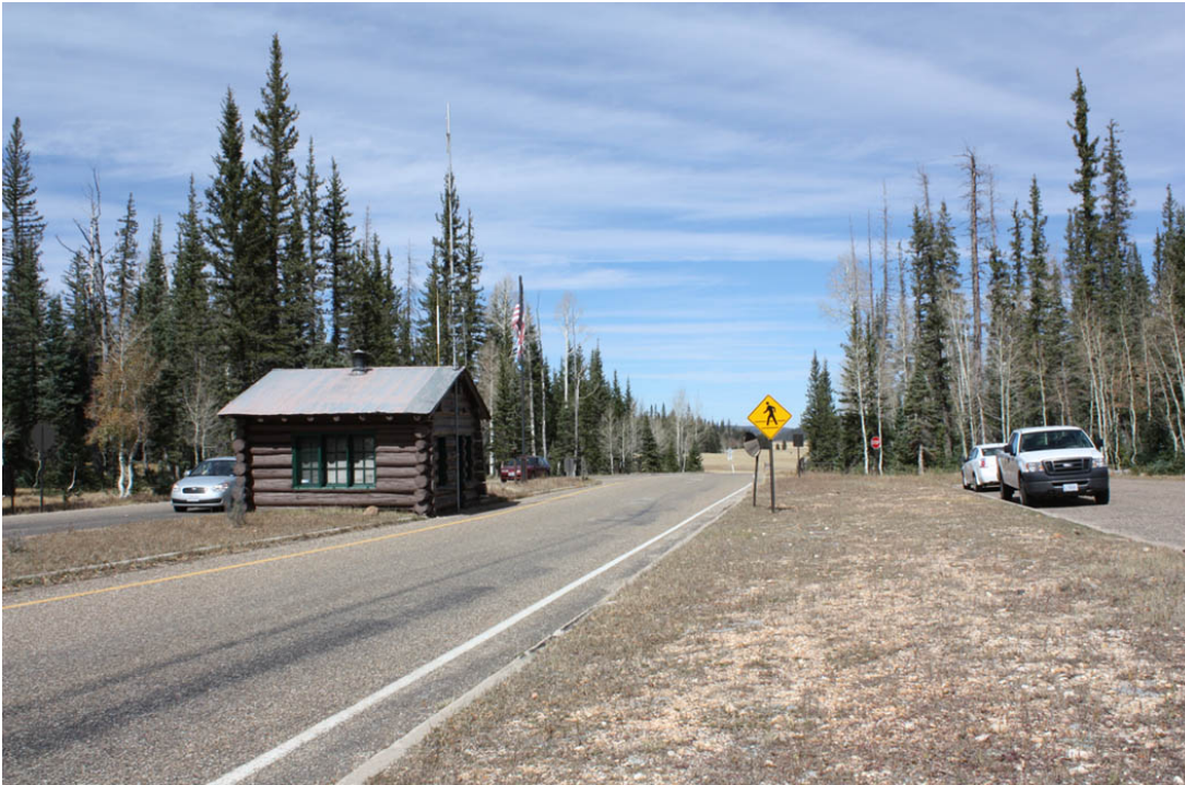
Entrance Road from South looking North, 2010. Photograph by Carrie Mardorf, October 2009.
