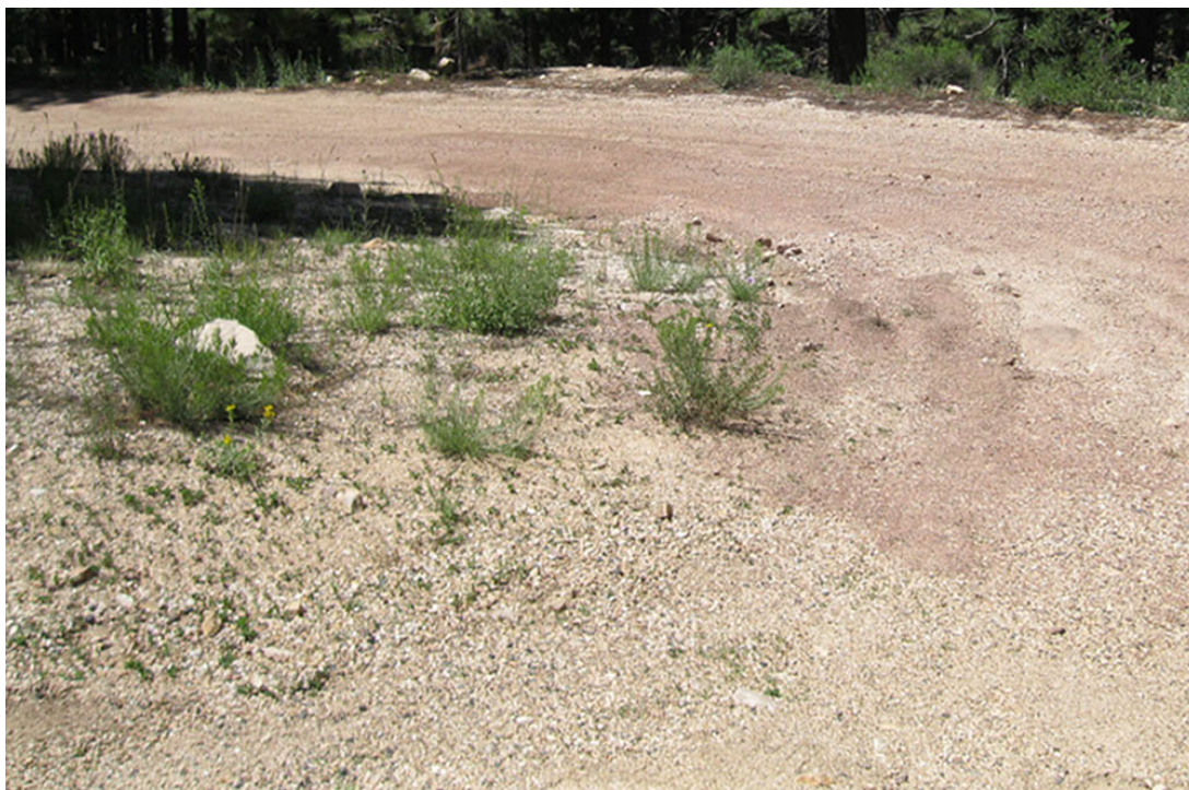
Motel access road, built by the CCC, facing west, August 2010. Source: NPS.
