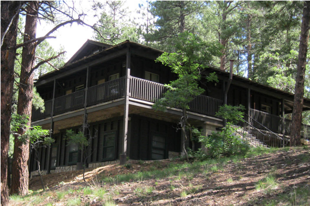
Motel from unpaved pathway, facing northeast, August 2010. Source: NPS.
