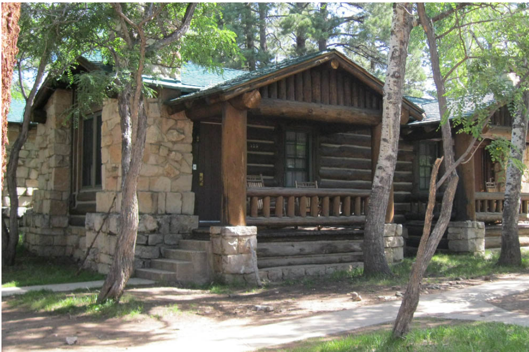
Deluxe cabins, facing north, August 2010. Source: NPS.
