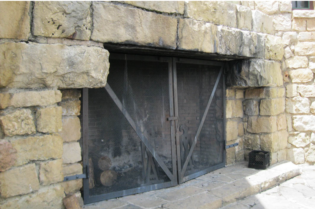
Fireplace on east lodge terrace, facing northwest, August 2010. Source: NPS.
