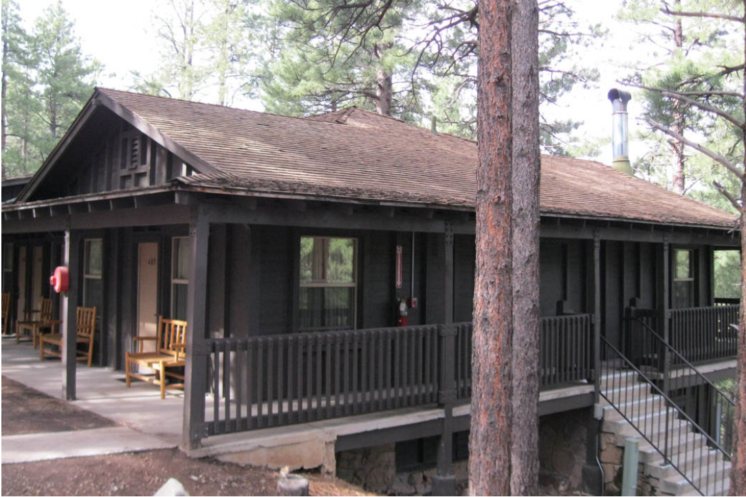
Motel building off of entrance road, facing southwest, August 2010. Source: NPS.
