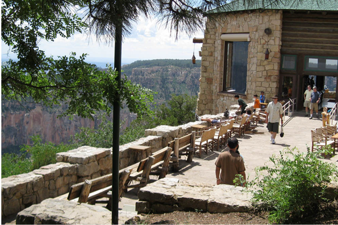
The main lodge building is sited on the canyon rim, facing southwest, August 2010. Source: NPS.
