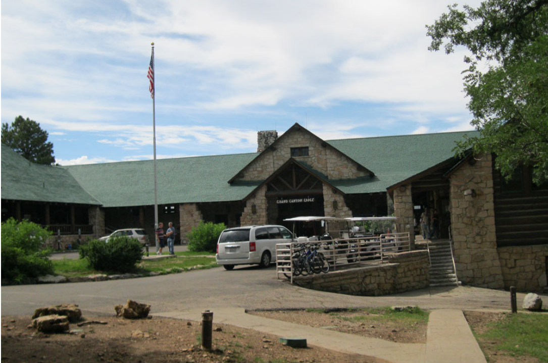
View of the main lodge building from the entrance road corridor, facing south/southeast, August 2010. Source: NPS.
