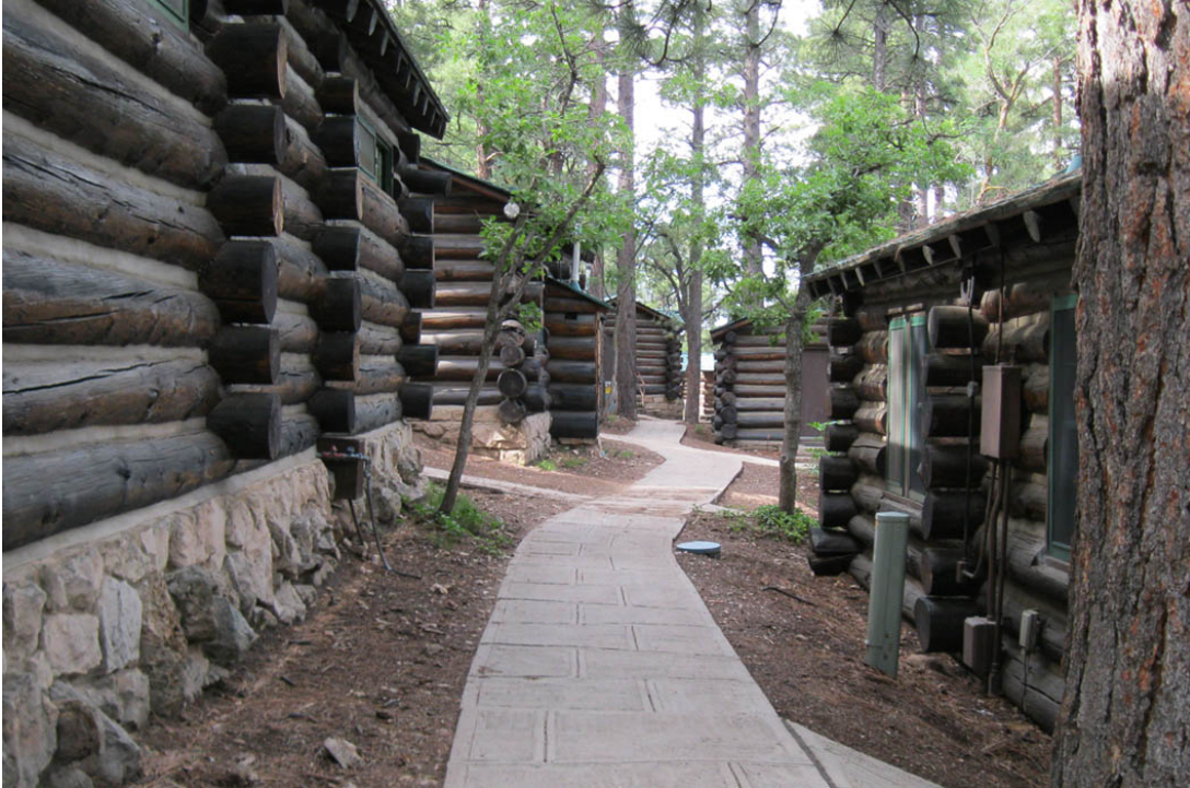
Organization of standard cabins on west side of Bright Angel Peninsula, facing south, August 2010. Source: NPS.
