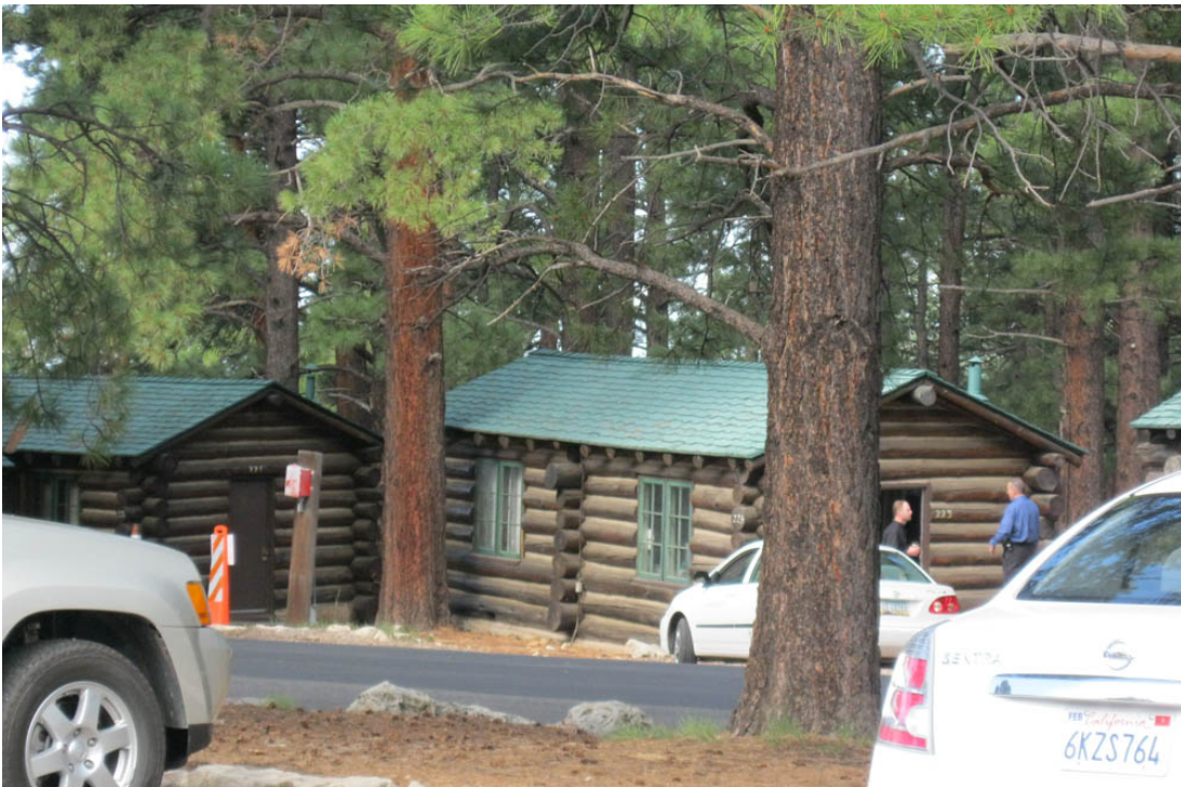
View of standard cabins from main parking area, demonstrating the density of the cabin area, facing west, August 2010. Source: NPS.
