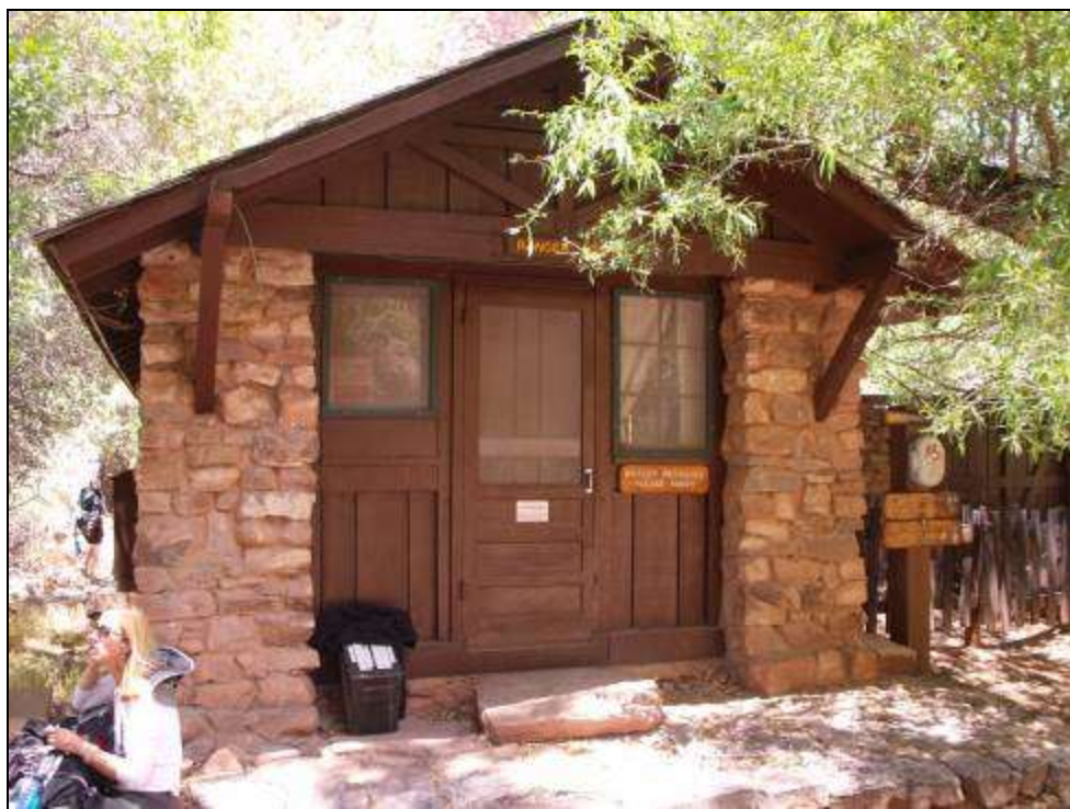
Photograph 61. Main elevation of the Cottonwood Ranger Residence, looking north, 2011. Source: LSD.
