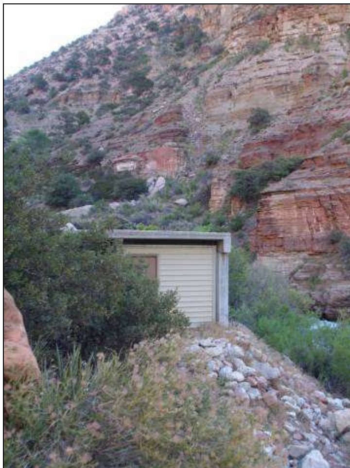
Photograph 70. Modern helipad and storage building in the vicinity of the Roaring Springs Pumphouse Operator's Residence, looking north, 2011. Source: LSD.
