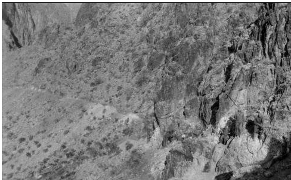
Photograph 8. Photograph of a trail crew building the Yaki (Kaibab) Trail, date unknown. Note the use of air and power tools (visible at right) (Photograph courtesy of the GRCA Archives, Grand Canyon National Park).
