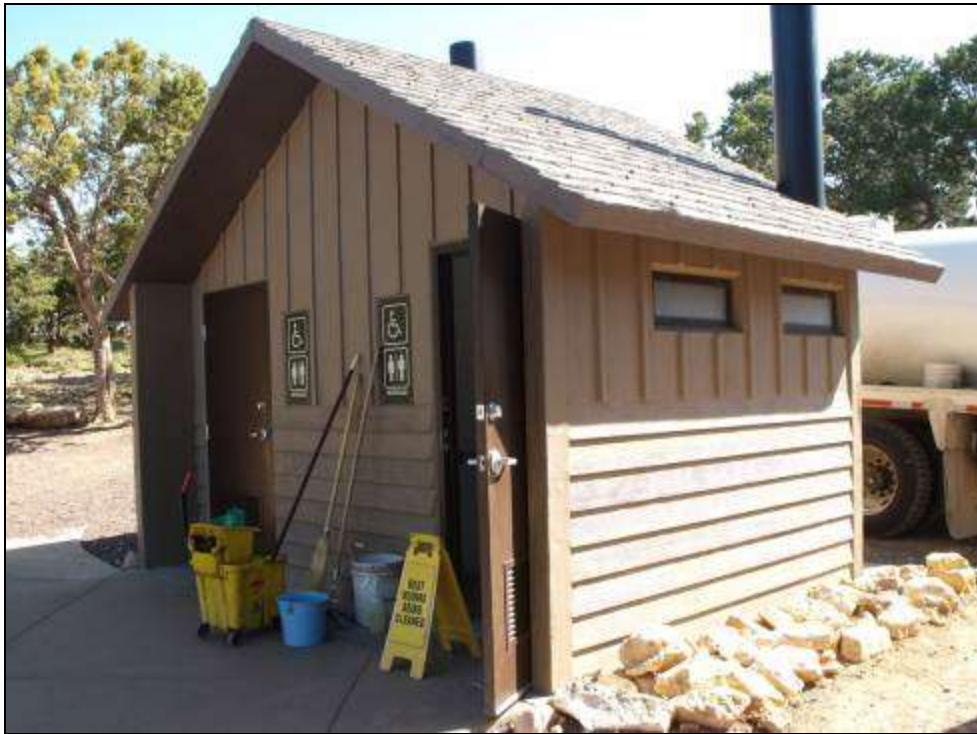
Photograph 54. Restroom building at Yaki Point, looking north, 2011. Source: LSD.
