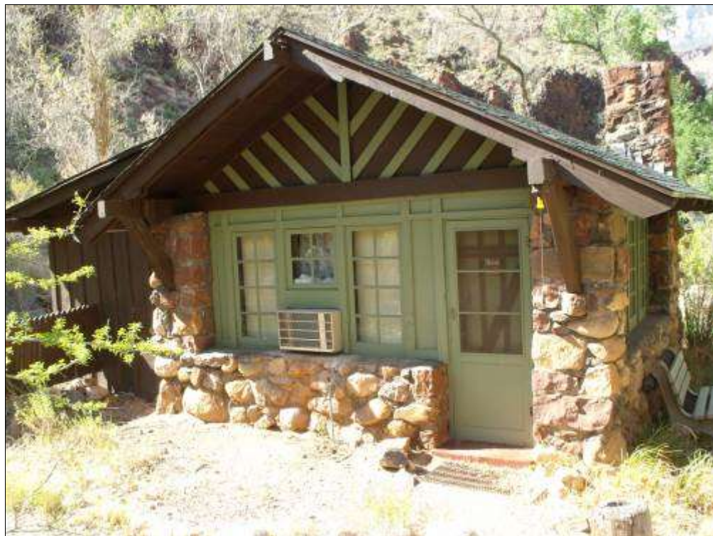
Photograph 36. Northern elevation of the Manager's Cabin, looking south, 2011. Source: LSD.
