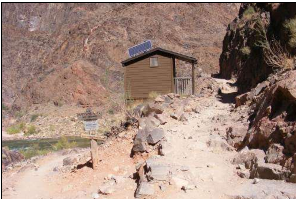
Photograph 31. Pipe Creek restroom building, looking north, 2009. The Colorado River Trail is visible to the right of the building. Note the stone edging along the left edge of the trail. Source: LSD.
