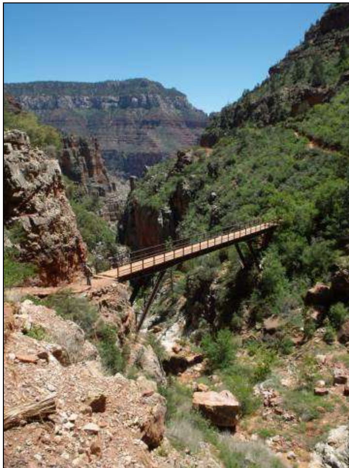
Photograph 60. Bridge in the Redwall, looking north, 2011. Source: LSD.
