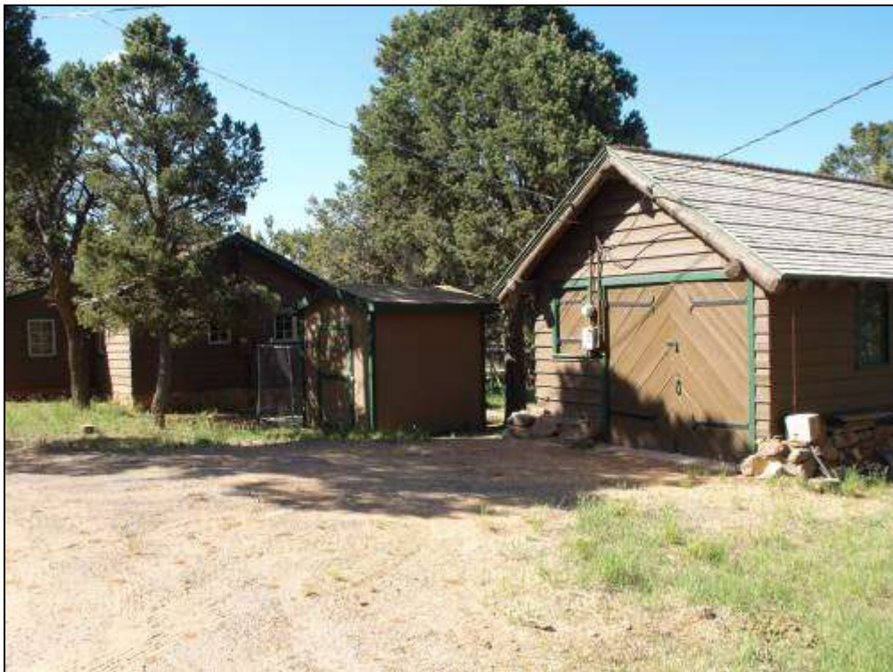
Photograph 52. The NPS Residence (at left), NPS Garage (at right), and a modern storage shed (in center) at Yaki Point (South Kaibab Trailhead), looking northeast, 2011. Source: LSD.
