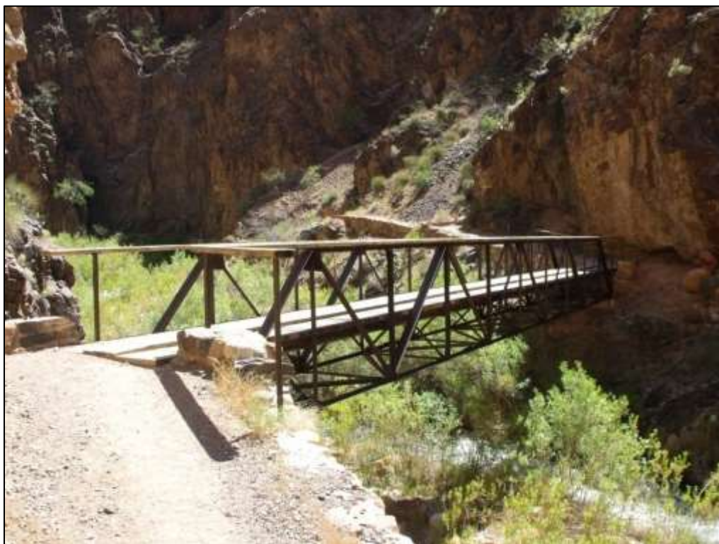
Photograph 116. Approaching footbridge within “The Box” along the North Kaibab Trail looking north, 2011. Source: LSD.
