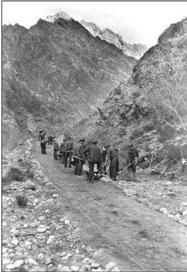
Photograph 15. CCC enrollees performing side ditching along the North Kaibab Trail, date unknown (Photograph courtesy of the GRCA Archives, Grand Canyon National Park).
