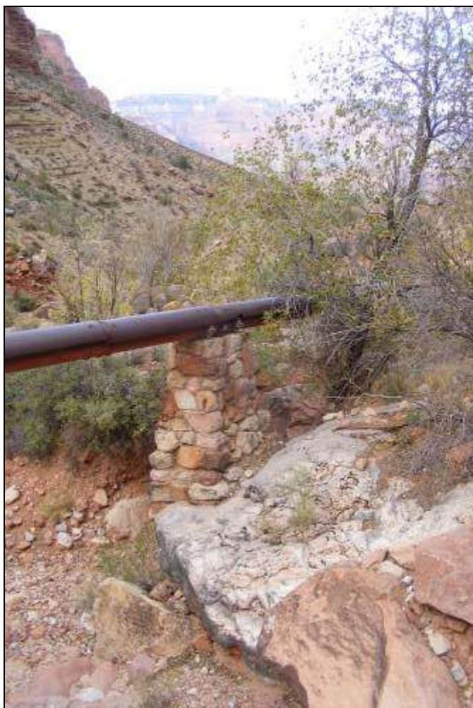
Photograph 27. Support pier of the original SPRR Trans-canyon Water System, looking northeast, 2009. Source: LSD.
