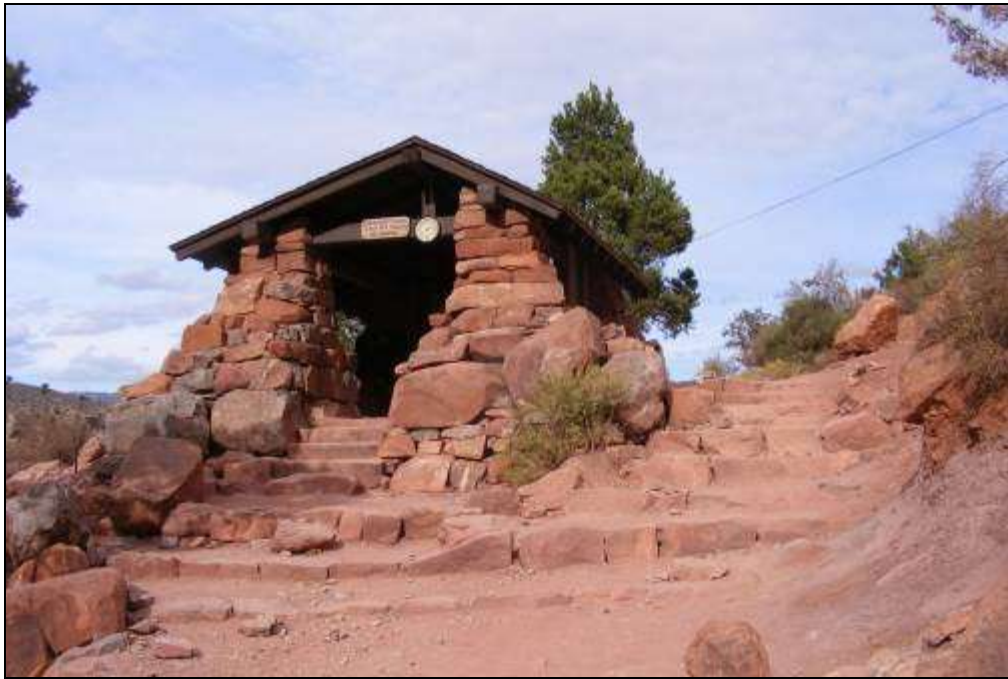
Photograph 24. Three Mile Rest House, looking north, 2009. Source: LSD.
