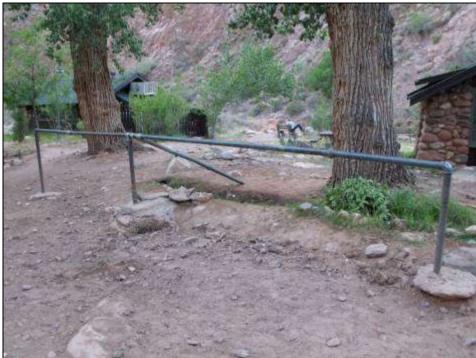
Photograph 86. Earthen irrigation ditch in the vicinity of Guest Cabins No. 10 and 11 at Phantom Ranch, facing southwest, 2011. Source: LSD.
