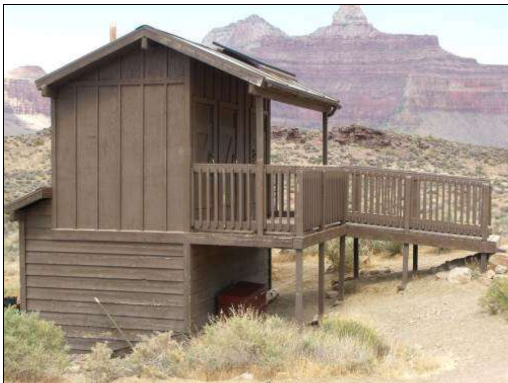
Photograph 50. Restroom building at the Tip-off, looking north, 2011. Source: LSD.
