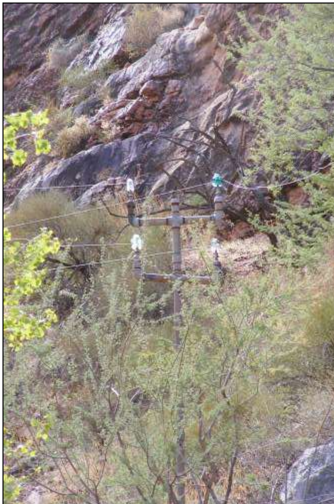
Photograph 26. Steel pole of the CCC-constructed Trans-canyon Telephone Line, ca. 1935, looking west, 2009. Source: LSD.
