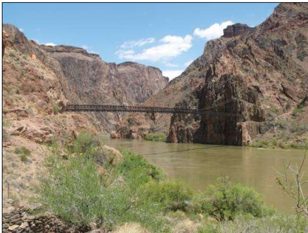
Photograph 43. Kaibab Suspension Bridge, looking southeast, 2011. Source: LSD.
