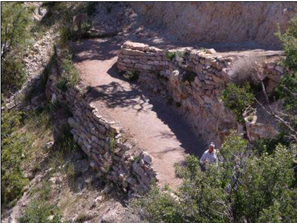
Photograph 46. Dry-laid stone retaining walls near the South Kaibab Trailhead, looking southeast, 2011. Source: LSD.
