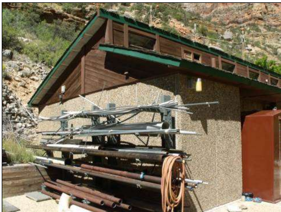
Photograph 68. Pumphouse located within the Roaring Springs Landscape Area, looking southeast, 2011. Note the non-contributing wooden retaining wall to the left of the pumphouse. Source: LSD.
