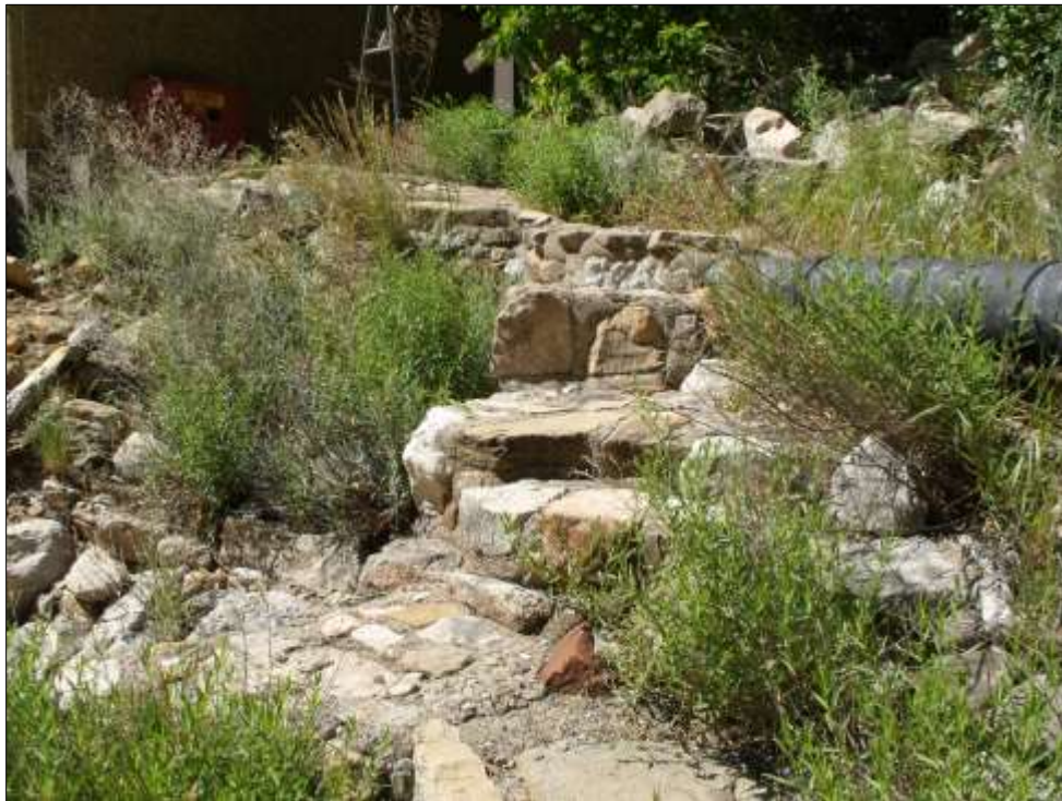
Photograph 112. Stone steps leading from a footpath to the modern Pumphouse facility at Roaring Springs, looking northeast, 2011. Source: LSD.
