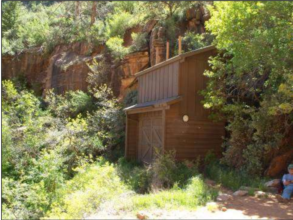
Photograph 57. Waterless restroom building at Supai Tunnel, looking northeast, 2011. Source: LSD.
