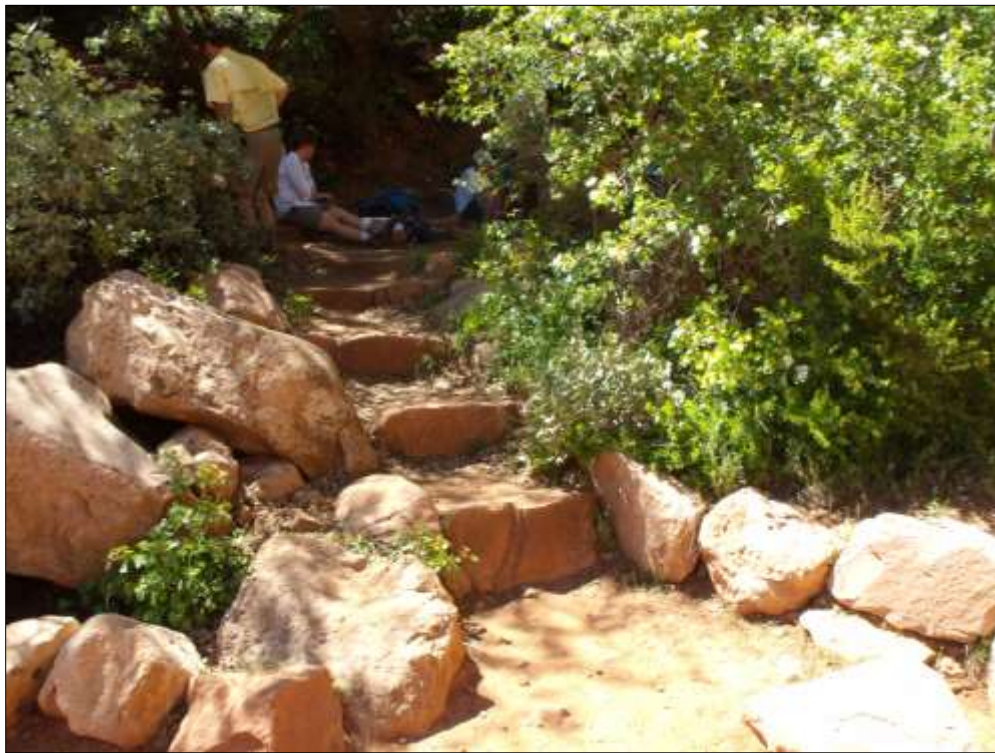
Photograph 107. Stone steps leading from the North Kaibab Trail to the Supai Tunnel restroom building, looking northwest, 2011. Source: LSD.
