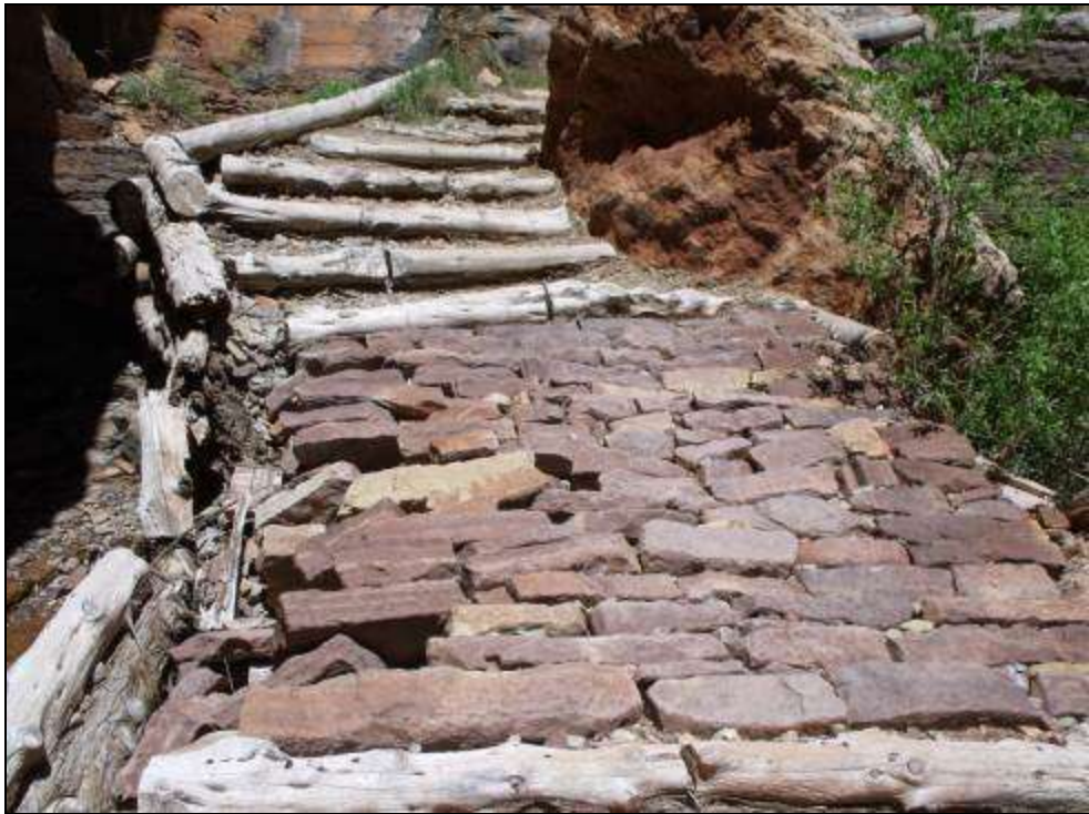
Photograph 59. North Kaibab Trail, showing stone paving and log steps in the vicinity of the Needle, looking west, 2011. Source: LSD.
