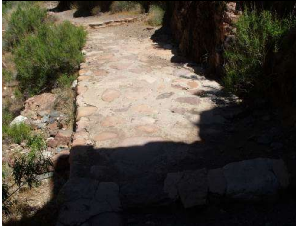
Photograph 58. Native stone water bar and concrete and stone spillway located along the North Kaibab Trail within the "Box" formation, looking northeast, 2011. Source: LSD.
