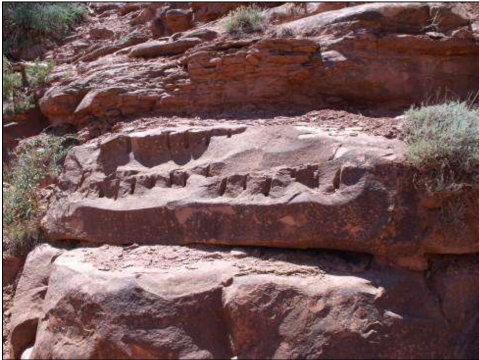
Photograph 90. Series of charge holes visible along the South Kaibab Trail, resulting from the trail's construction in 1924–1925, looking west. Source: LSD.
