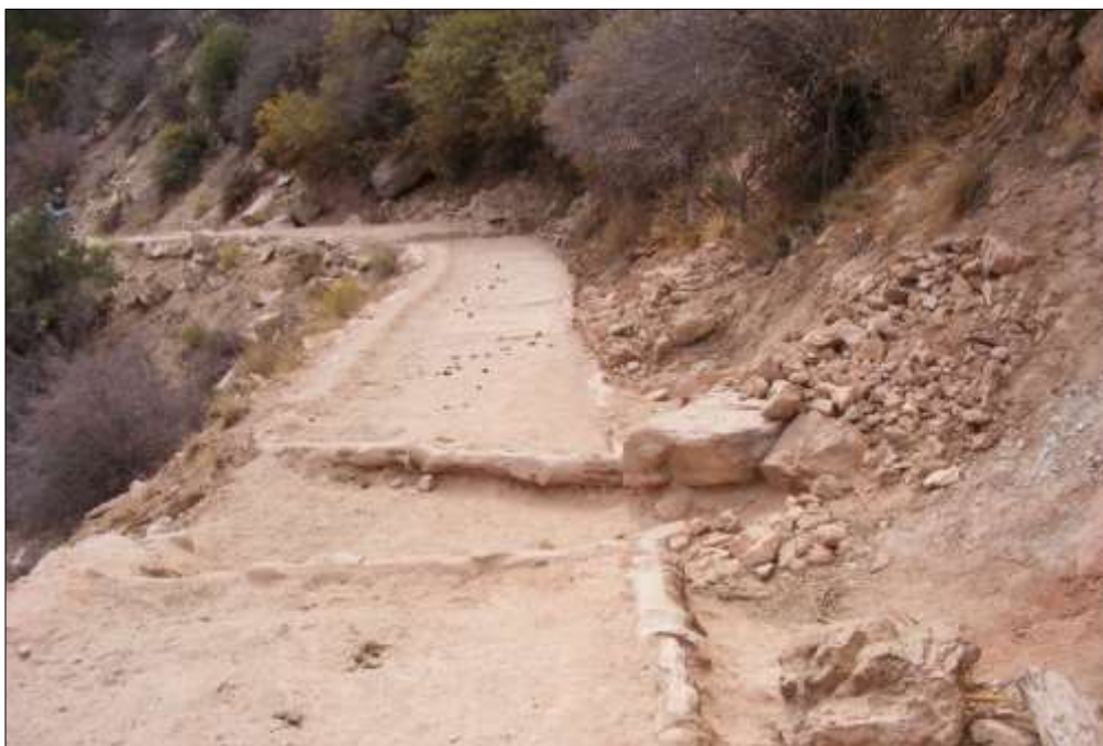
Photograph 99. Log water bars along the Bright Angel Trail, facing north, 2009. Source: LSD.
