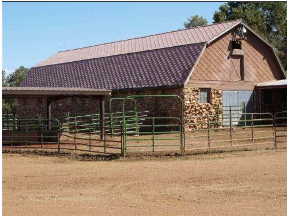
Photograph 53. Fred Harvey Mule Barn, showing the southern and western elevations, a detached shade structure, and corral fencing, looking north, 2011. Source: LSD.
