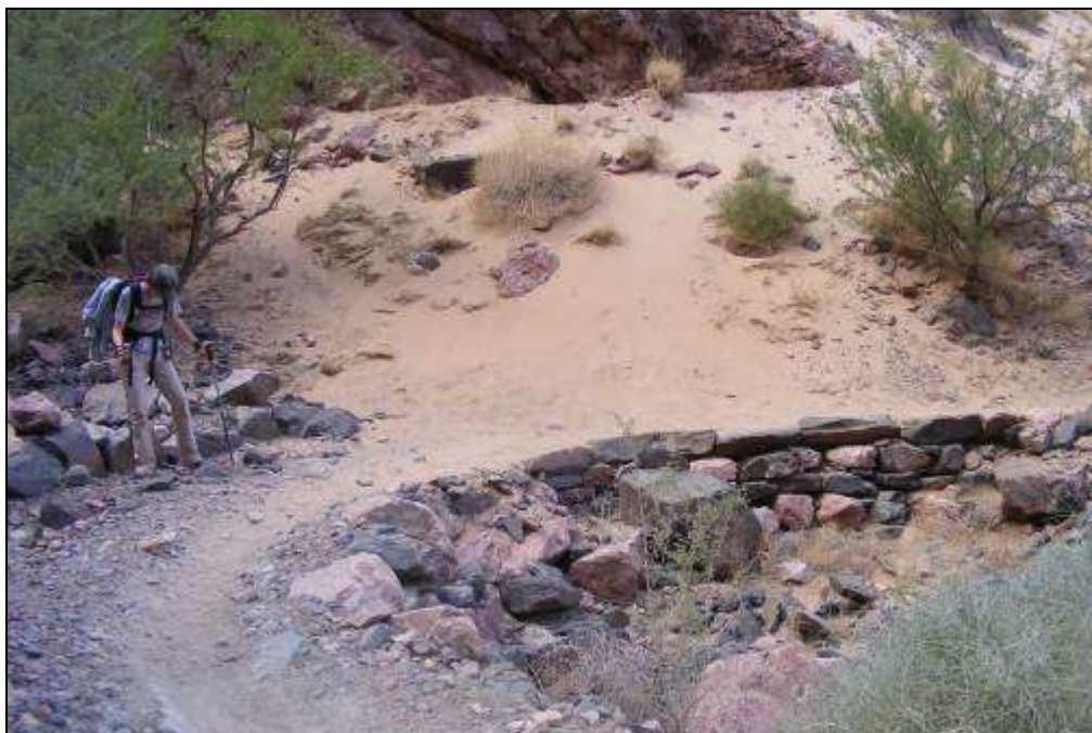
Photograph 33. Stacked stone retaining wall along the Colorado River Trail, looking southwest, 2009. Source: LSD.
