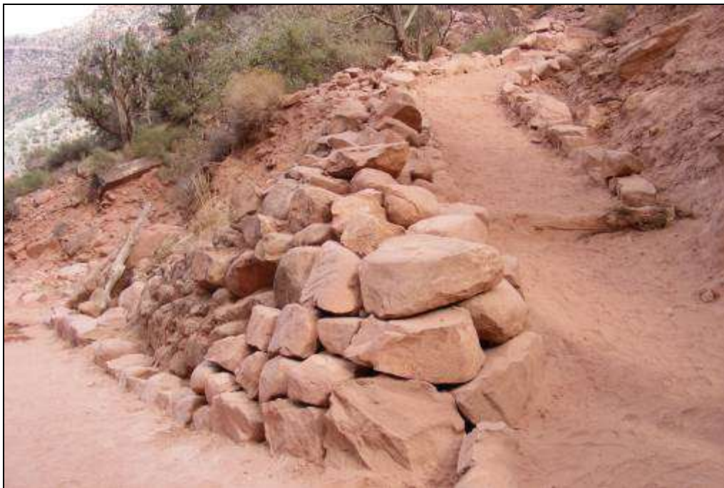
Photograph 72. Switchback with dry-stacked stone infill, looking north, 2009. Source: LSD.
