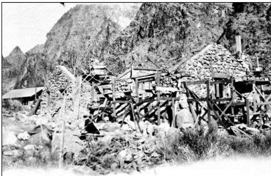
Photograph 7. Photograph showing construction of the main lodge at Phantom Ranch, ca. 1922. Note the stone walls and wood lintels above the windows (Photograph courtesy of the GRCA Archives, Grand Canyon National Park).
