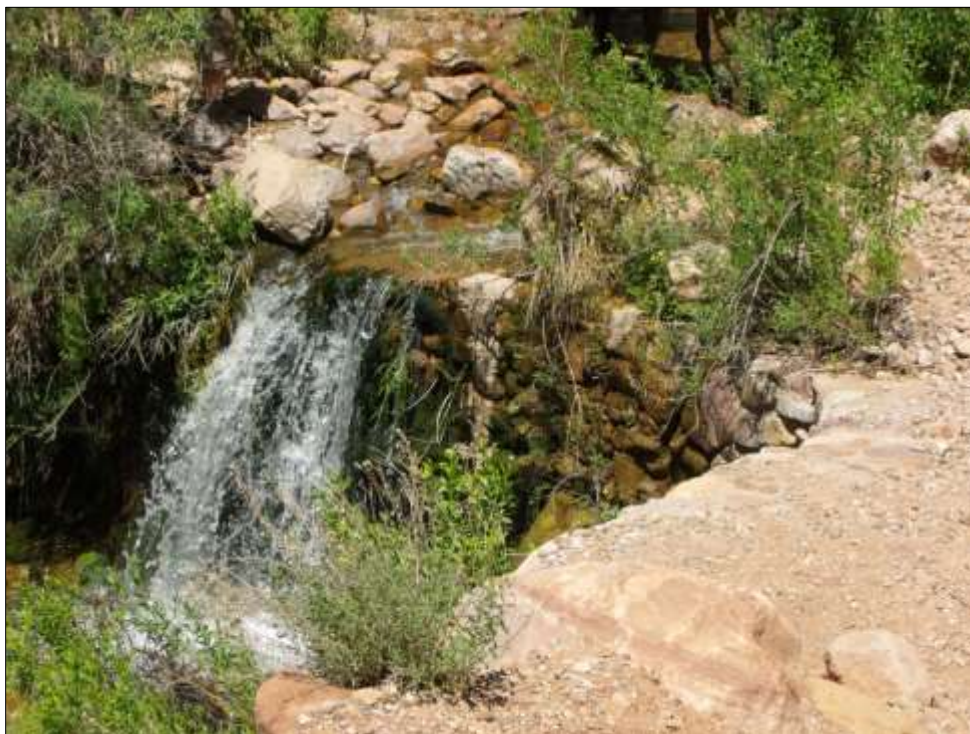
Photograph 126. Concrete and rock retaining wall at the Wall creek crossing on the North Kaibab Trail, facing east, 2011. Source: LSD.
