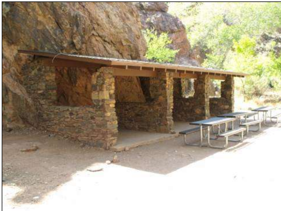
Photograph 65. Adirondack Shelter at Bright Angel Campground, looking northeast, 2011. Source: LSD.
