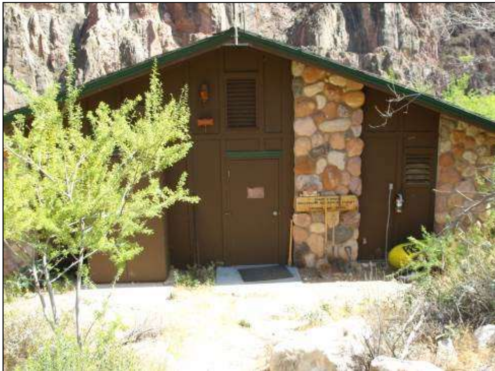
Photograph 42. Northern elevation of the Sewage Treatment Plant on the Bright Angel Creek delta, looking south, 2011. Source: LSD.
