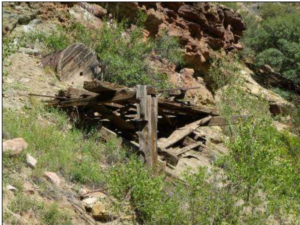
Photograph 67. Remnant of the UPRR cable tramway documented in the Day Use Area at Roaring Springs, looking northwest, 2011. Source: LSD.
