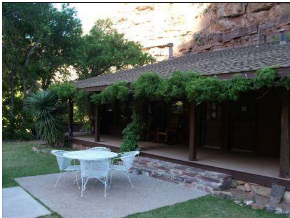
Photograph 69. Main elevation of the former Pumphouse Operator's Residence at Roaring Springs, looking southwest, 2011. Source: LSD.
