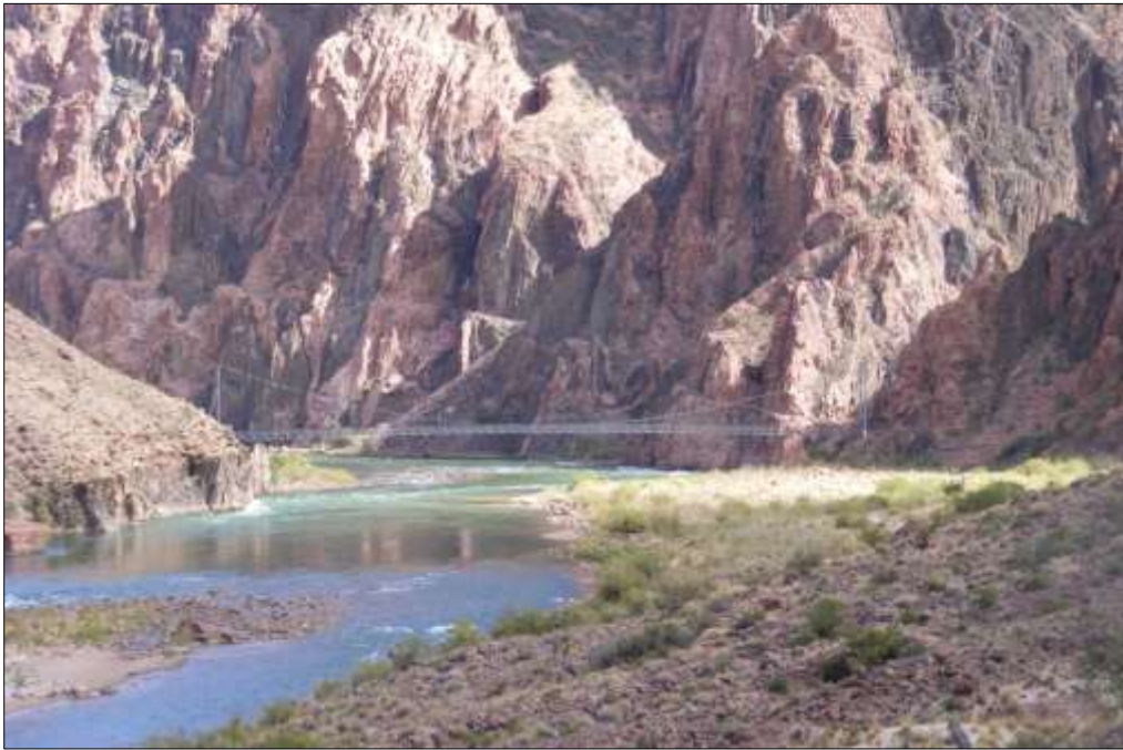
Photograph 141. View of the Colorado River and Silver Bridge from the Colorado River Trail, looking east, 2011. Source: LSD.
