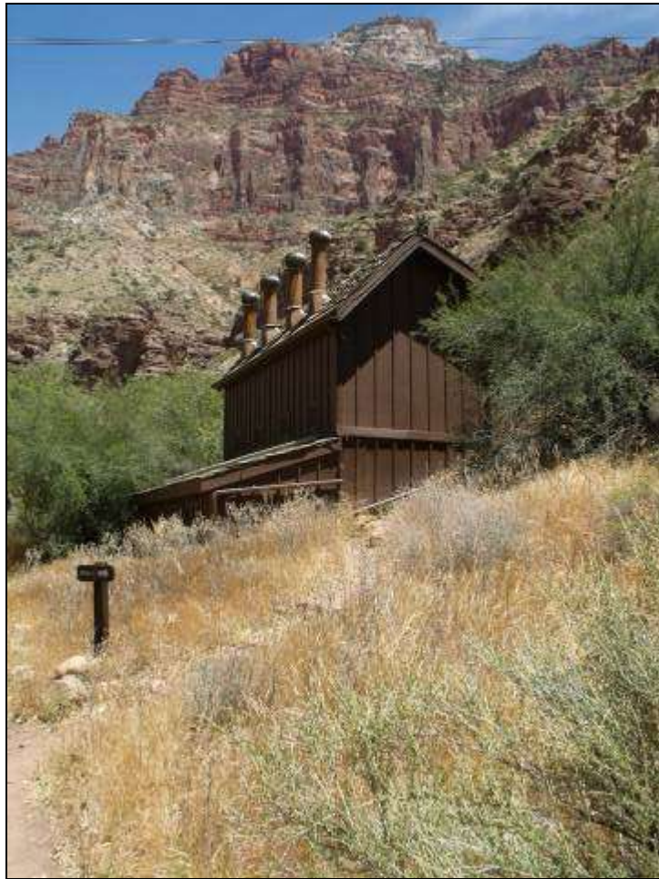
Photograph 62. Cottonwood Campground restroom building, looking north, 2011. Source: LSD.
