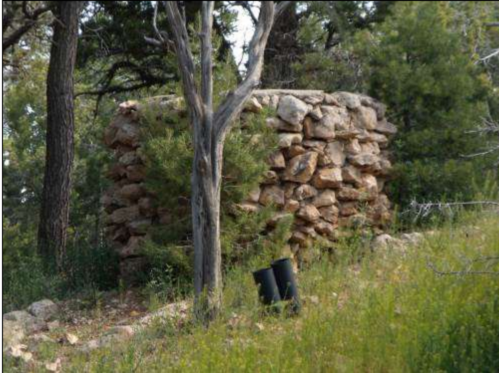
Photograph 51. Yaki Point (South Kaibab Trailhead) Residence Cistern, looking north, 2011. Source: LSD.
