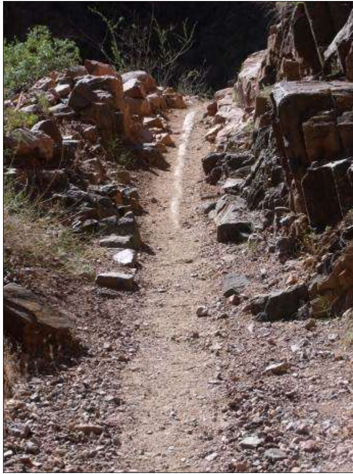
Photograph 82. Exposed pipeline of the Trans-canyon Water System visible along the North Kaibab Trail, facing east, 2011. Source: LSD.
