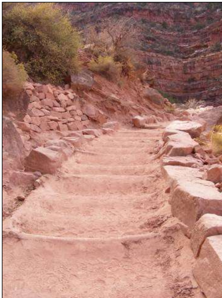
Photograph 77. Native stone and wood features used for trail stabilization, 2011. Source: LSD.
