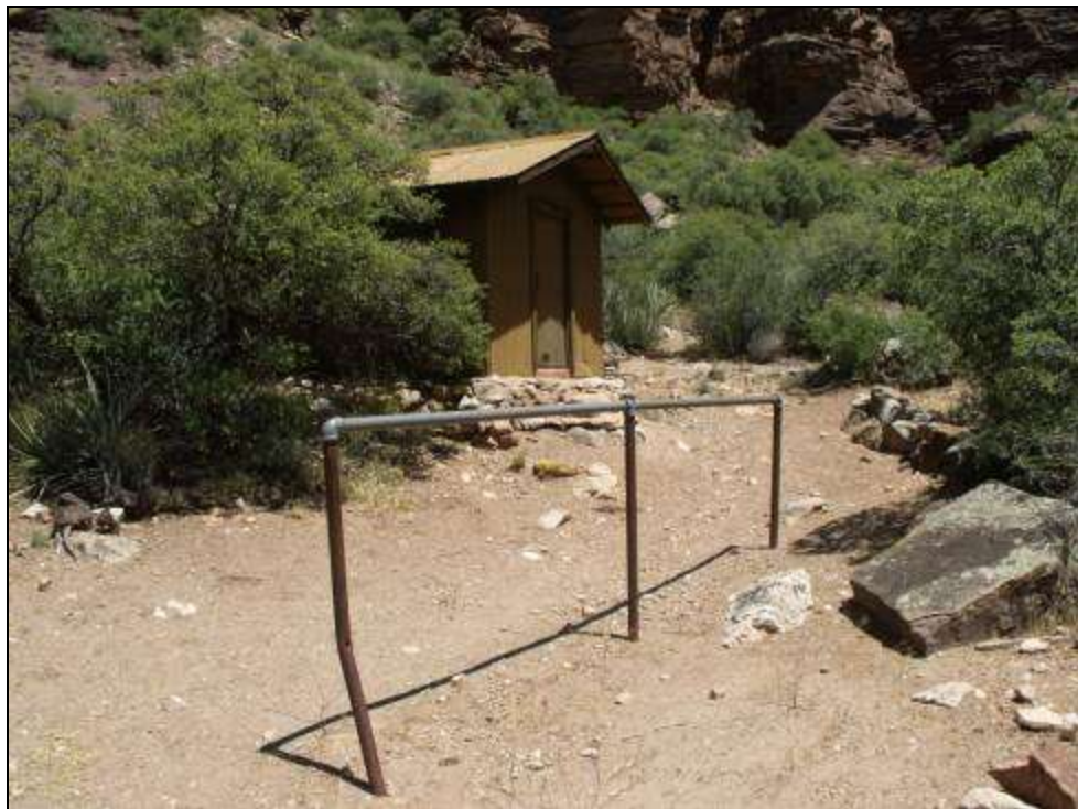
Photograph 63. Storage building to the southeast of the Cottonwood Campground Mule Corral, looking east, 2011. Source: LSD.
