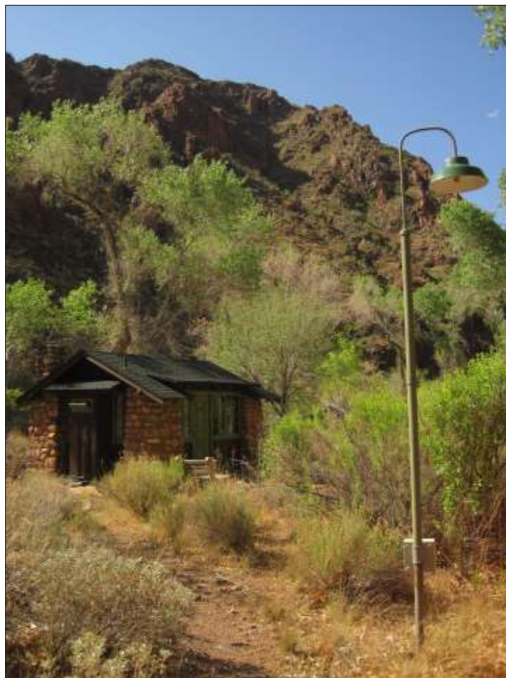
Photograph 101. Lamppost to the southeast of Guest Cabin No. 1, facing northwest, 2011. Source: LSD.
