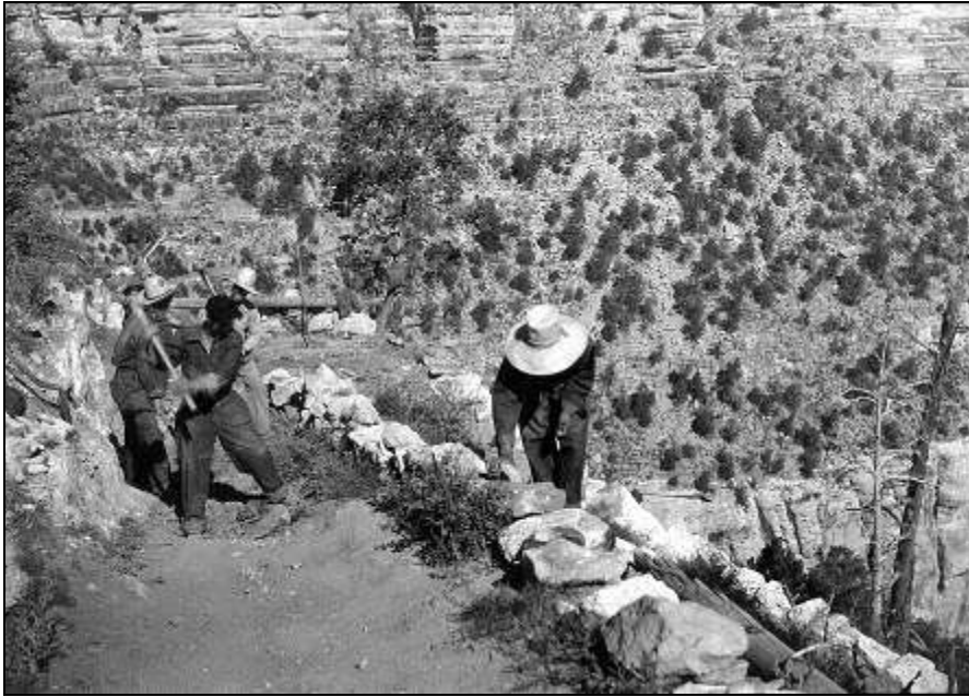
Photograph 14. Photograph showing a CCC work crew repairing a switchback retaining wall along the upper Bright Angel Trail just below Kolb Studio, ca. 1935 (Photograph courtesy of the GRCA Archives, Grand Canyon National Park).
