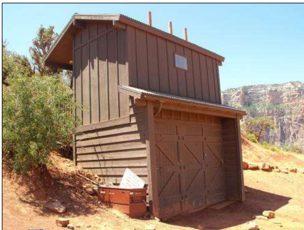
Photograph 49. Cedar Ridge restroom building, looking southeast, 2011. Source: LSD.
