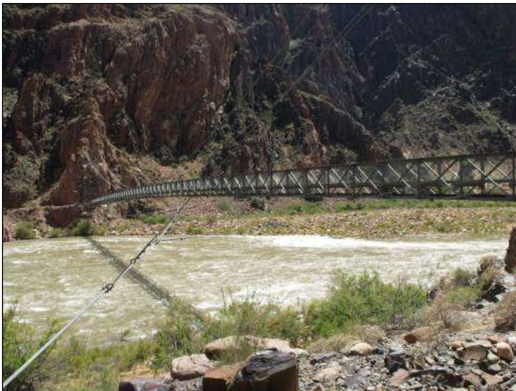
Photograph 32. Silver Bridge, showing cables and steel decking, built in 1966 as part of the Trans-canyon Water System, looking northeast, 2009. Source: LSD.
