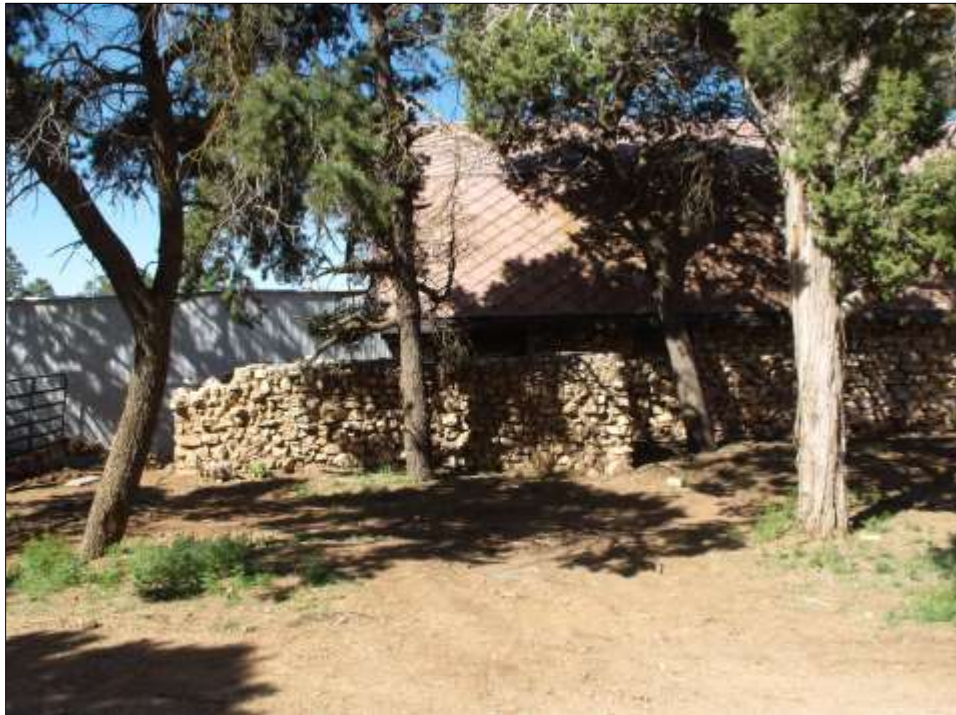
Photograph 84. Rectangular stone cistern to the east of the Harvey Mule Barn, facing southwest, 2011. Source: LSD.
