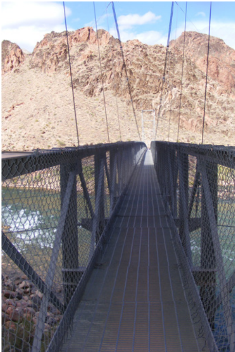
Photograph 7. Silver Bridge, showing cables and steel decking, built as part of the trans-canyon water system, looking northeast, 2009. Source: Logan Simpson Design (LSD).
