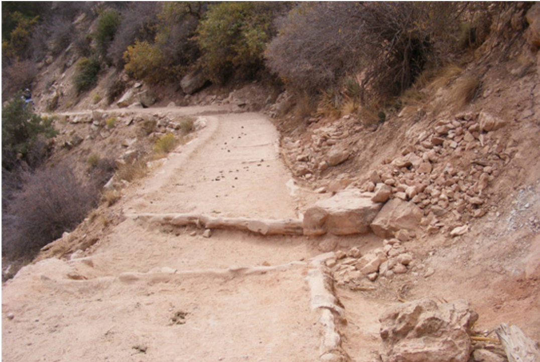
Photograph 16. Wood pine log water bars along the Bright Angel Trail, facing north, 2009. Source: Logan Simpson Design (LSD).
