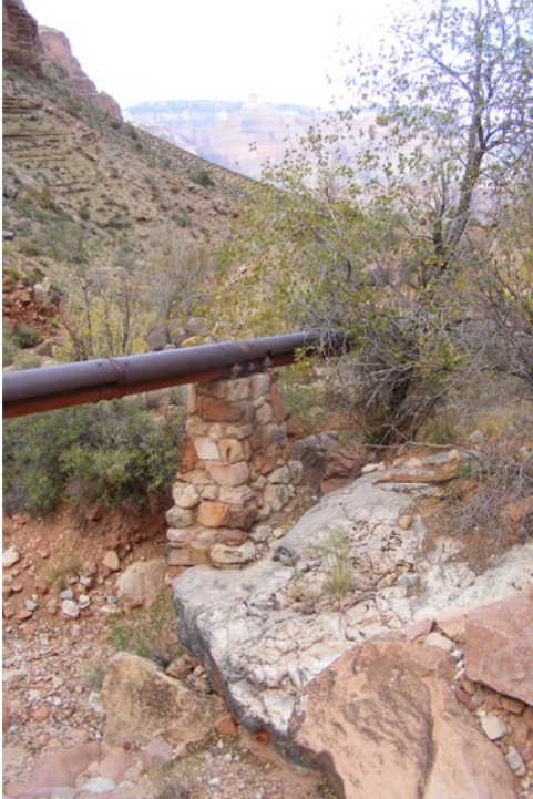
Photograph 5. Steel water line and stone support pier of the trans-canyon water system, looking northeast, 2009. Source: Logan Simpson Design (LSD).
