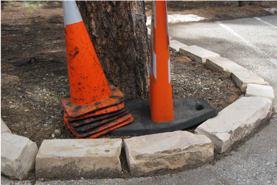
Sandstone curbing lines the edges of the Camper Store parking node within the Campground Sub-Area, looking southeast, August 2010. Source: National Park Service.
