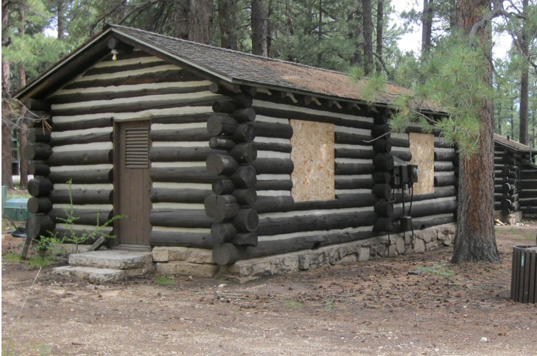
The duplex cabins are situated west of the exposed-frame cabins within the Campground Sub-Area, looking west, August 2010. Source: National Park Service.
