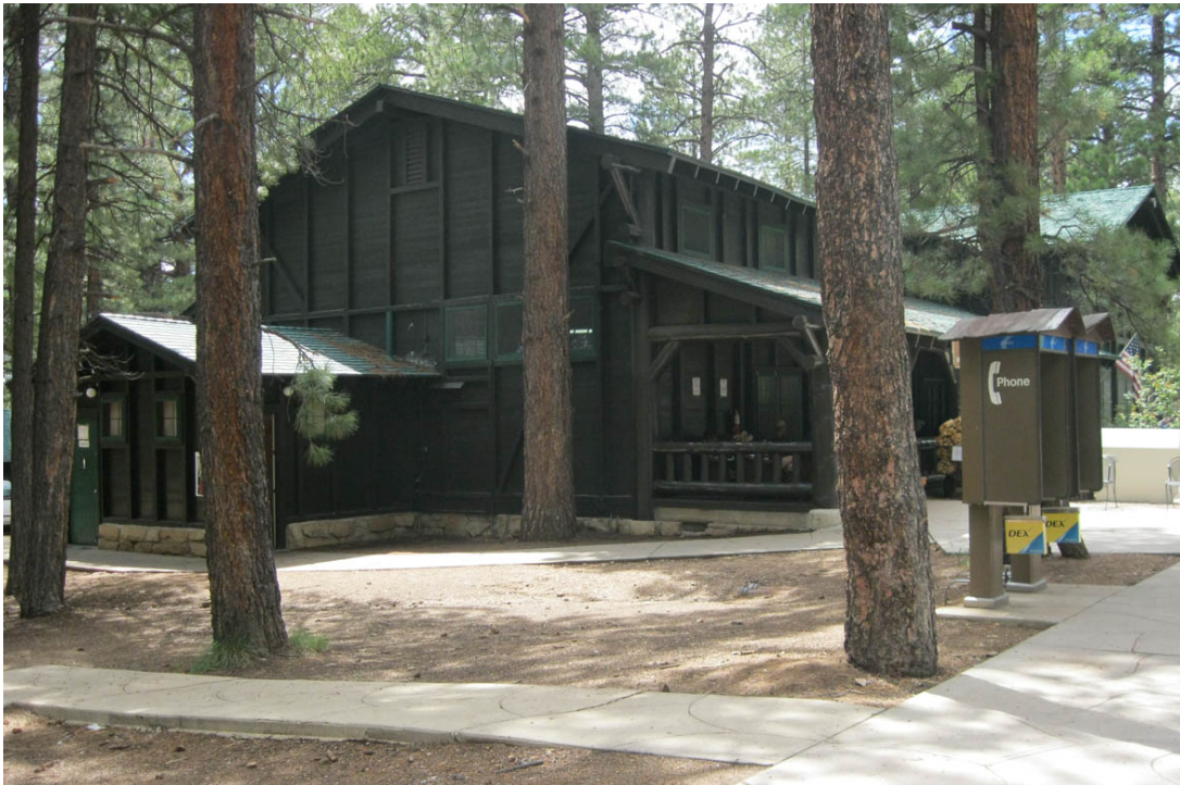
The Camper Store, a Rustic-style building, serves as the cornerstone of the Campground Sub-Area, looking west, August 2010. Source: National Park Service.
