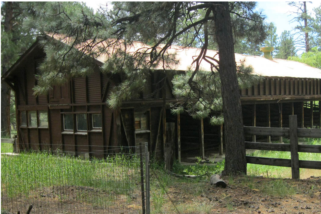
The Mule Stable anchors the western border of the Concessionaire Sub-Area, looking west, August 2010. Source: National Park Service.
