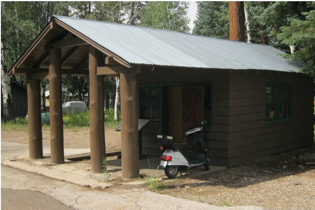
The Rustic-style Gas and Oil Station is located in the Headquarters, Housing, and Maintenance Sub-Area, looking west, August 2010. Source: National Park Service.
