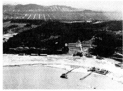
figure 40. This view, taken 1,000 feet over the field, clearly shows the overall layout of the airfield in the mid-1920s: the "airmail" and "reserve" hangars, added to the east (left) portion of the field in 1921-23; the administration and barracks complex at mid-field (right center); and one of the hangars to the west (far right). Crissy Field Road leads uphill and off the right edge to "officers' row" on the bluff above. (National Air and Space Museum)
