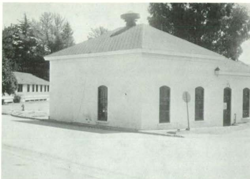
7. Pumphouse, Fort Baker, 1977.
