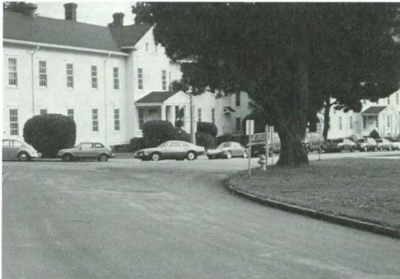
6. Coast Artillery Barracks, Fort Baker, 1977.
