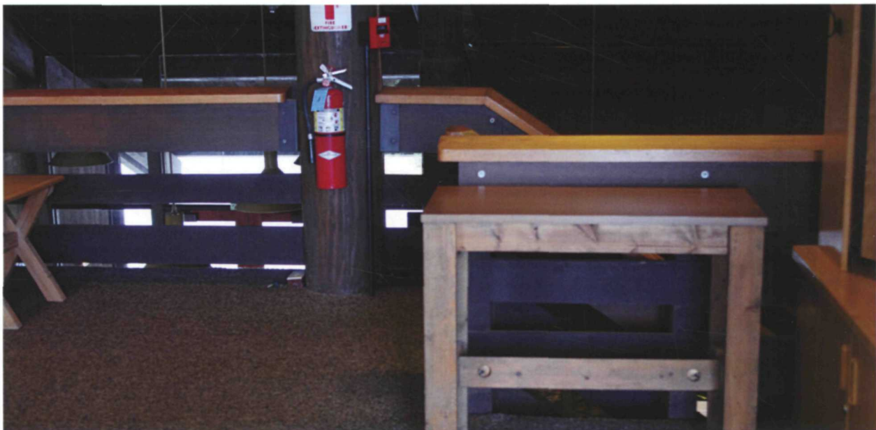
Figure 168. Railing on southeast corner of mezzanine room, May 2017.
