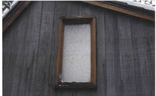
Figure 120. Casement window, March 2017.
