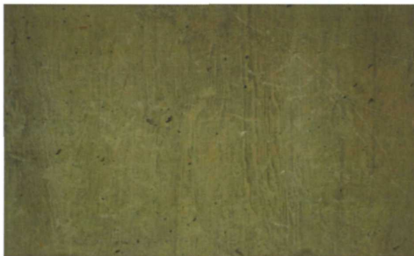
Figure 102. Foundation wall painted to mimic wood, May 2017.
