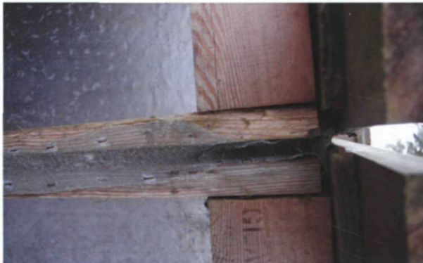
Figure 164. Opening in battens, March 2017.
