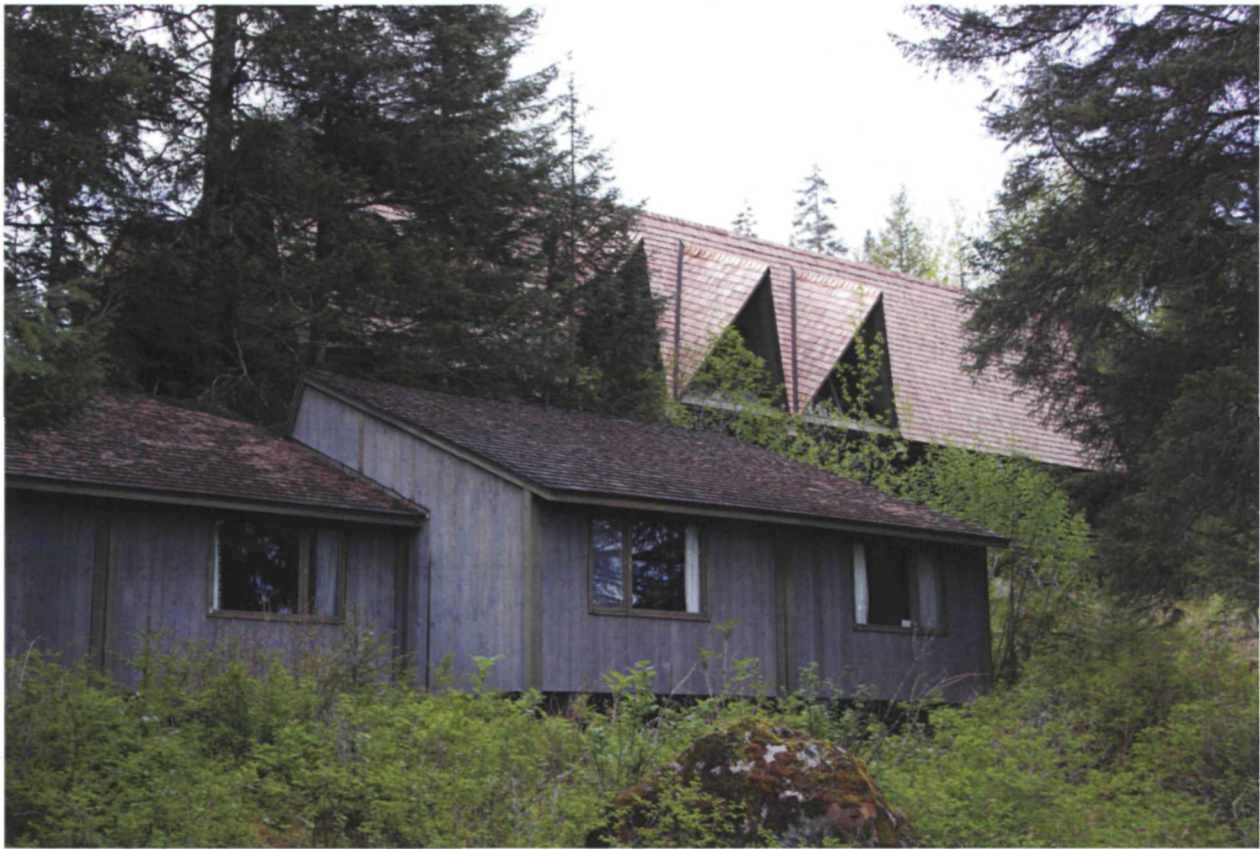
Figure 1. Glacier Bay Lodge Complex, looking southwest, May 2017.
