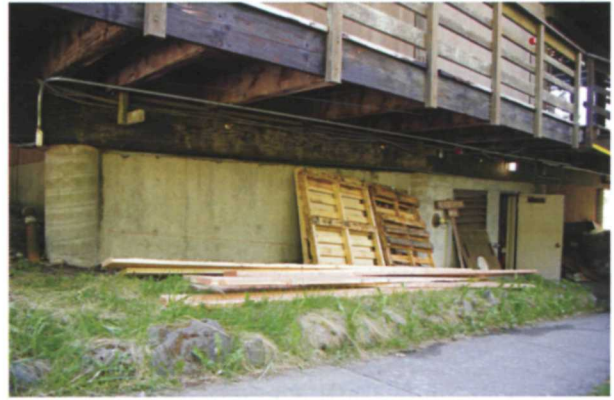
Figure 101. Lodge foundation, May 2017.
