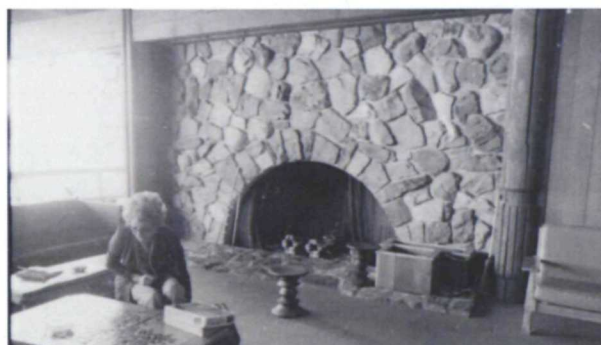
Figure 138. Cracks present in 1974, unknown photographer, circa 1974 (GLBA Archives, GLBA 6009 a-f).
