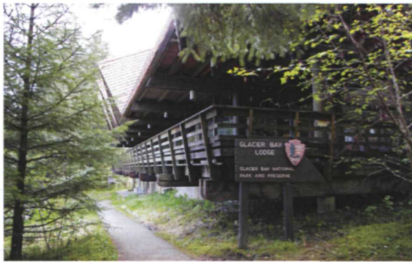
Figure 130. Lodge, south elevation, May 2017.
