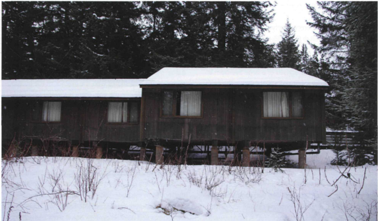
Figure 136. Cabin, rear elevation, March 2017.
