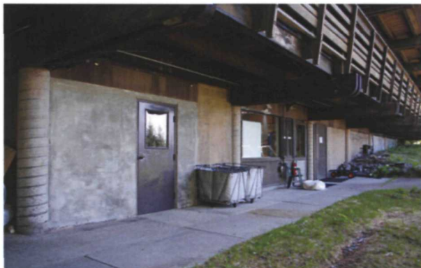
Figure 103. Plywood tops foundation on north elevation, May 2017.
