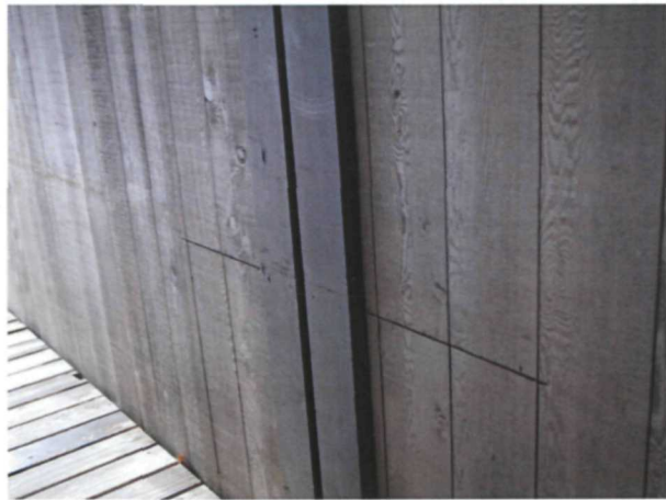
Figure 156. Cut in siding, March 2017.
