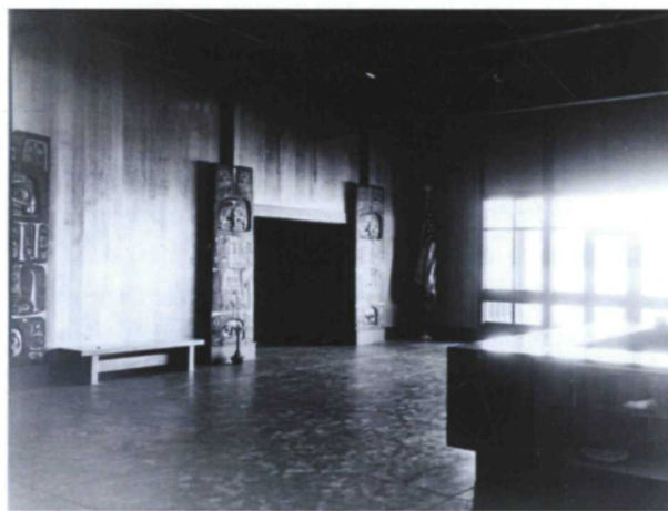
Figure 13. "Lobby interior of new visitor center, Sitka National Monument," photographed by Paul F. J. Schumacher, July 2, 1965 (SITK Museum Collection, SNM, Series 5, File Unit 119f).
