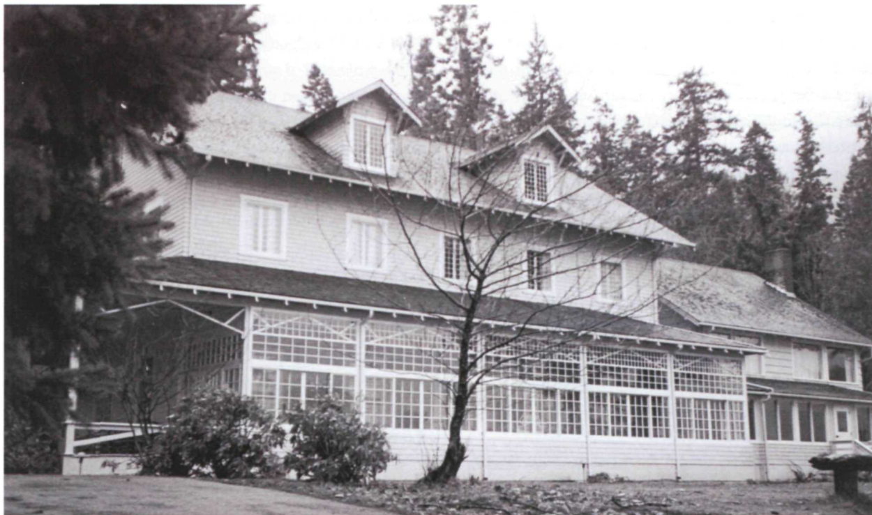
Figure 14. Lake Crescent Lodge, Olympic National Park, unknown photographer, 1999 (OLYM Archives, Maintenance Collection).
