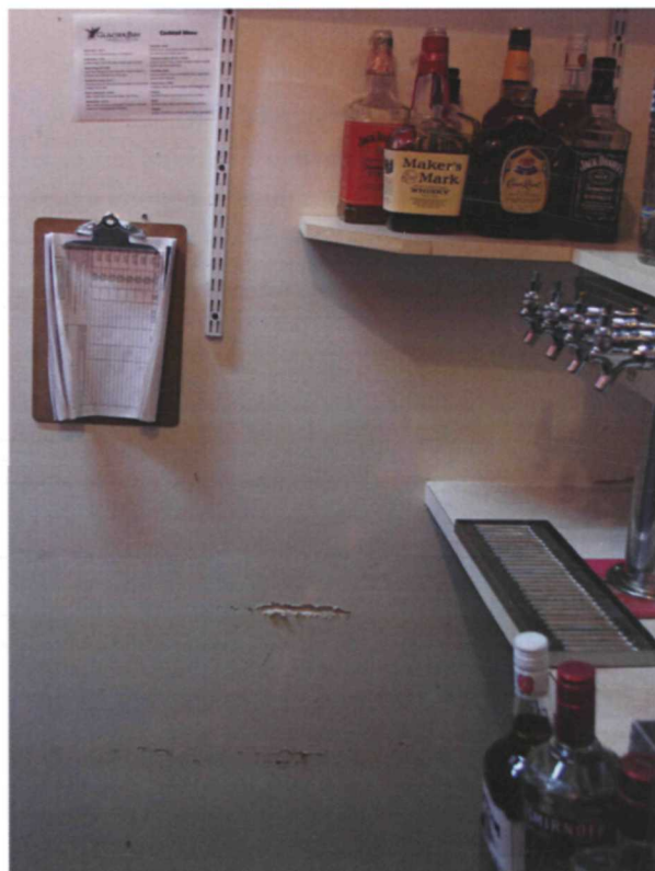
Figure 151. Cut in gypsum board in office wall, May 2017.
