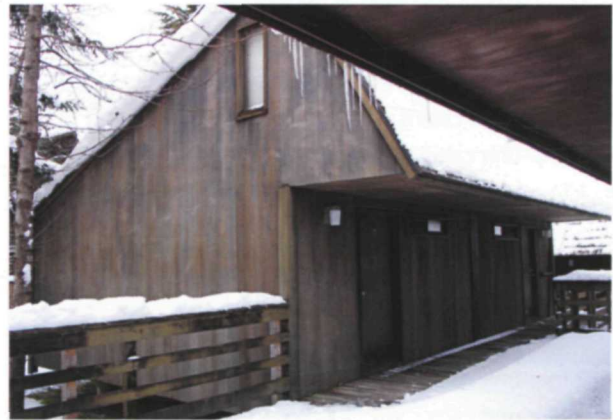
Figure 135. Cabin, front elevation, March 2017.
