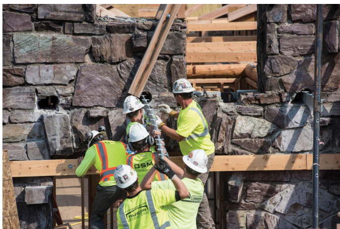
Figure 8. Construction crew fishes second-floor balcony's joist flitch through wall pocket. Courtesy of A Boring Photo.
