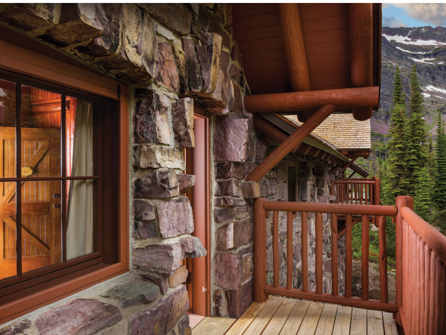
Figure 6. Completed roof and balcony framing as well as rehabilitated masonry. Note unremovable soot stain over door. Courtesy of Mark Bryant Photographics.
