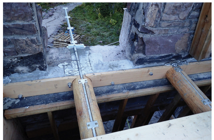
Figure 9. Second-floor balcony joist flitch grouted in wall pocket. Joists are supported on inside face of wall by a steel angle ledger.
