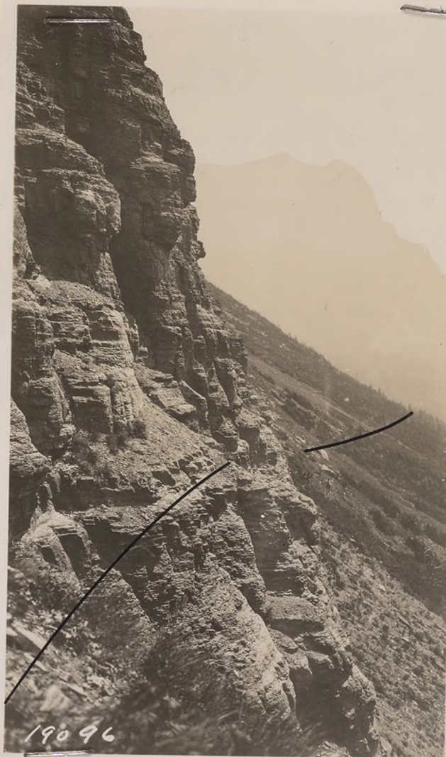
No. 19096. Sta. 66+50 east. Bench cutting just below tunnel. Three-hundred and fifty feet of one-inch hemp rope necessary when taking cross sections here. Going to the Sun Mountain in the Background.
