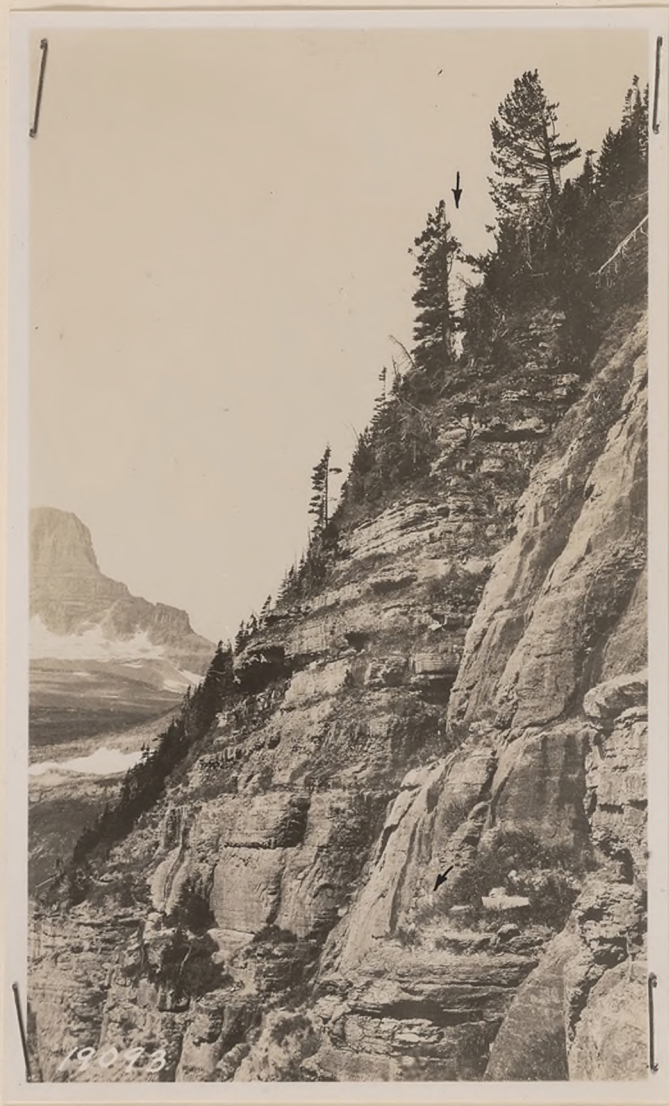
No. 19093. Proposed east portal of tunnel, Sta. 66+50 west. Stake in foreground and brush cutting at top indicates center line.
