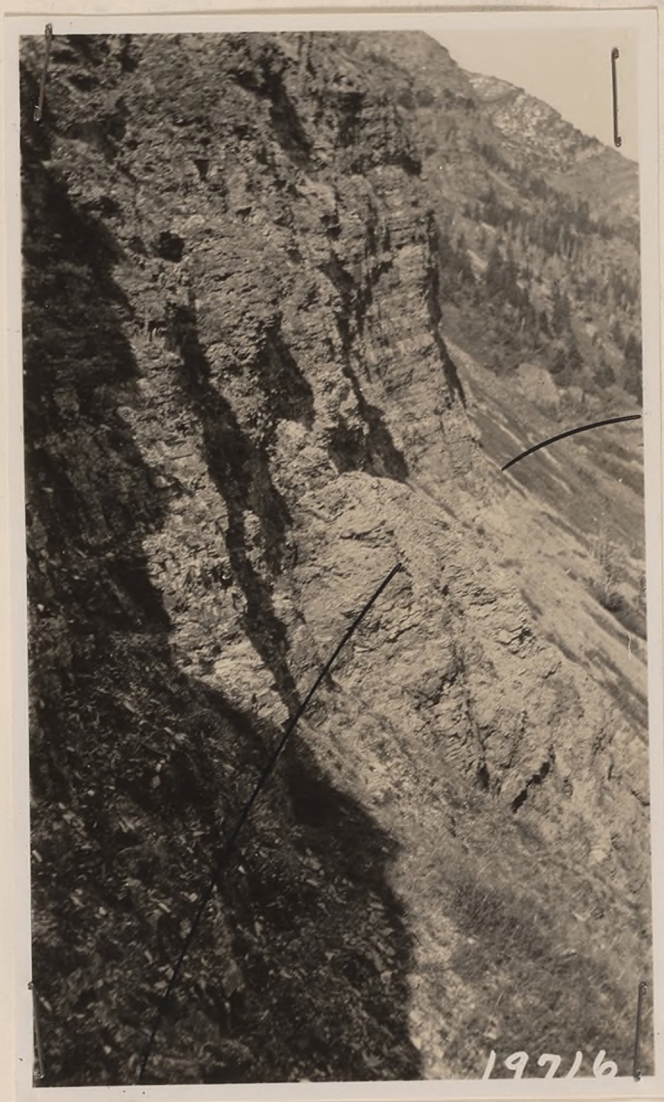
No. 19716. Looking east along cliffs, Sta. 518 to Sta. 523. End of survey and existing road is at Sta. 533.
