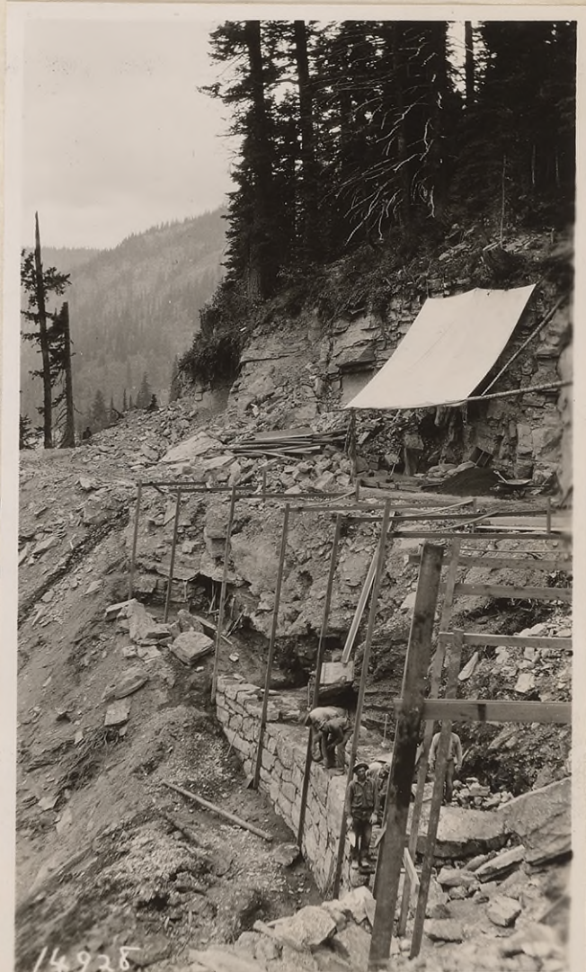
#14960. September, 1927. Showing end wall construction on cement rubble masonry culvert, 6' x 6', sta. 153. Also showing gasoline "dinky" engine and cars for hauling and making fill.
