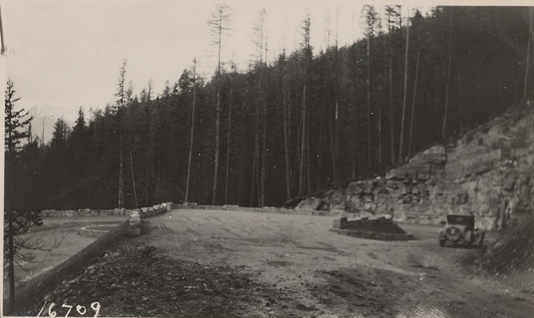
#16709 - View ahead from sta. 408 showing upper parking area, 8170 sq. ft. at "The Loop". Automobile on right side of main highway. Beginning of cement rubble masonry toe wall joining guard rail at left of car. Oct. 18, 1928.
