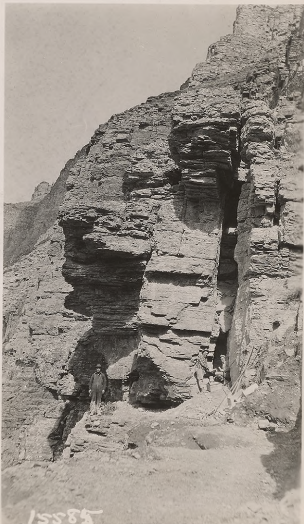
#15585 Sept. 1926 Sta. 38 ahead, showing "seam shooting" by stationmen. Advantage taken of natural seams in rock to place dynamite and powder charges. Limestone rock.
