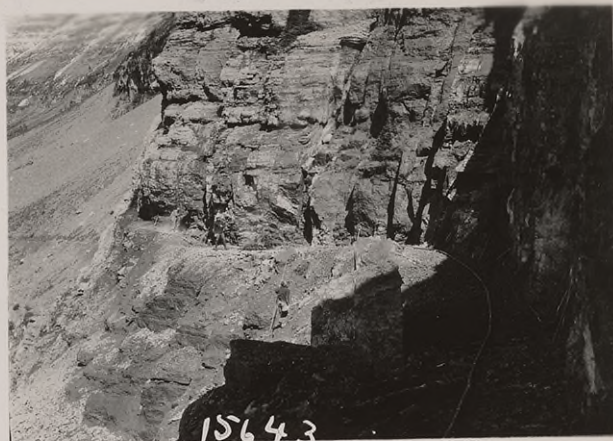
#15643. View showing close-up of saddle horse trail along face of cliff, 100 feet above road, stas. 35 to 45. Six feet wide. To be made safe by cement rubble masonry guard rail. October 1927.
