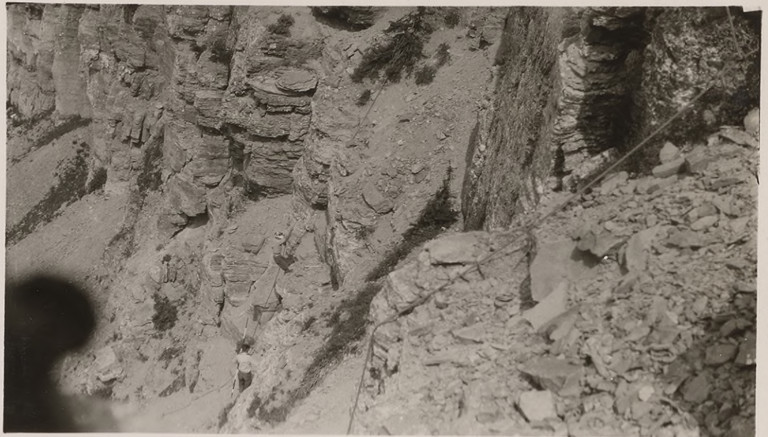
# ( Dept. of Motion Pictures, Dept. of Agri., film ) July, 1926. View showing cross-section party of engineers at work on difficult cliff sections, stas. 35 to 45. Note safety ropes. Steepness of cliffs and loose rocks made work extremely dangerous.
