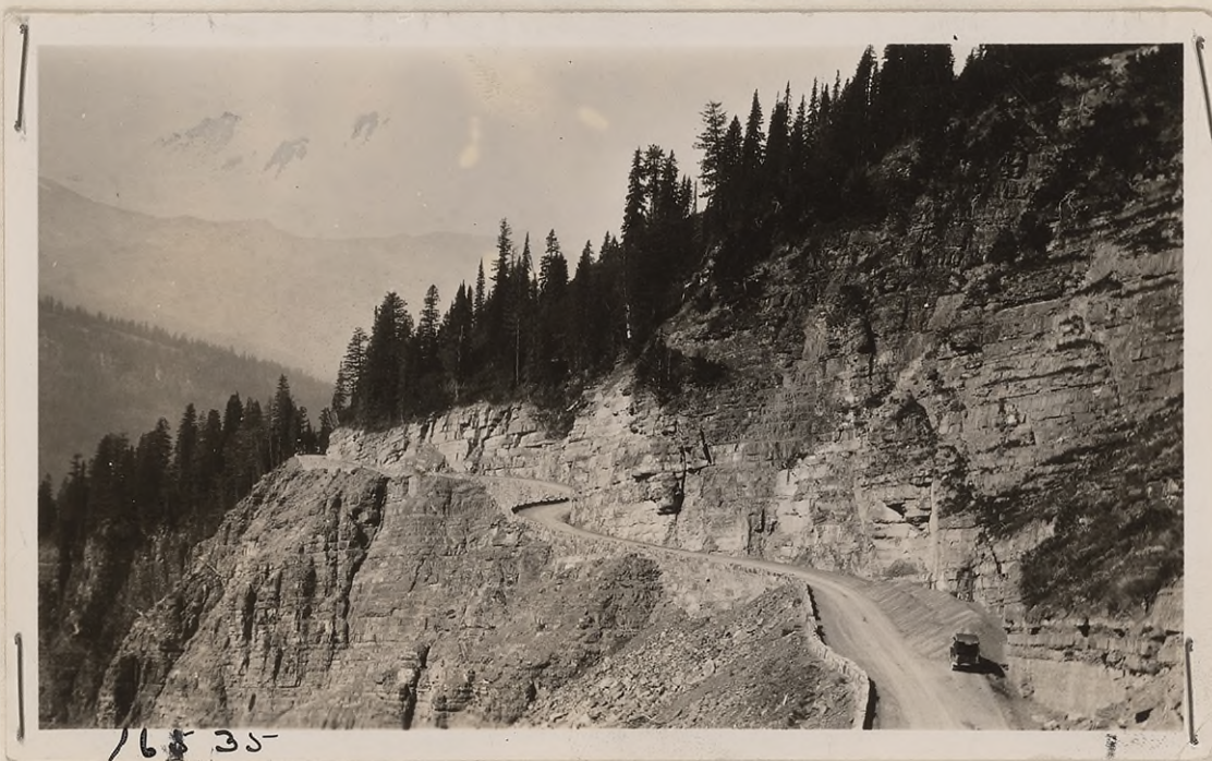
#16542 - Sta 89. Completed cement rubble masonry retaining walls and guard rails. Wall 47' maximum height. outer batter 1 to 10, inner batter 1/4 to 1, top thickness 1.65 ft. on 54° 30' curve. September, 1928.
