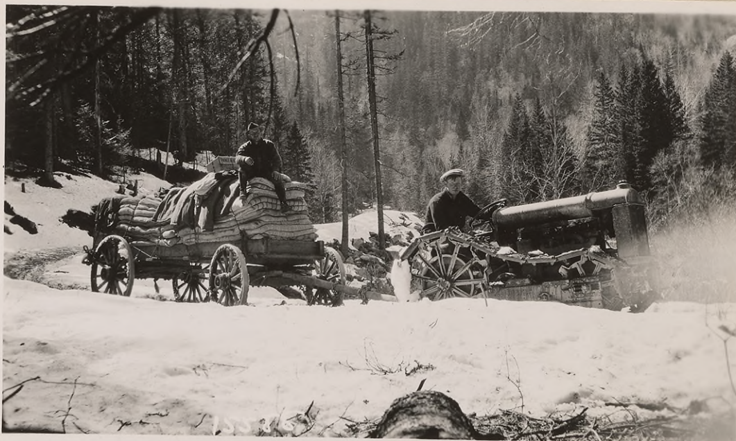
#15588. April 17, 1926. Fordson caterpillar tractor hauling supplies from cribbing on Mt. Cannon Section to camp #1. Prior to use of wagon, sled was necessary. This system of hauling was required for a period of about one month.
