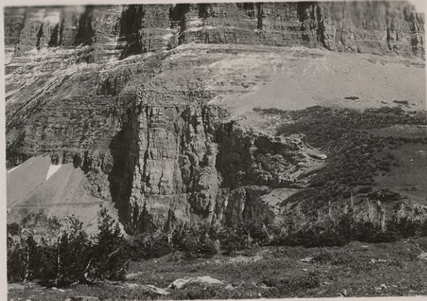
#15901. View of site of saddle horse trail above road, stas. 35 to 45. One hundred feet in elevation above roadway. Six feet wide. To be safe guarded with cement rubble masonry railing. October 1927.
