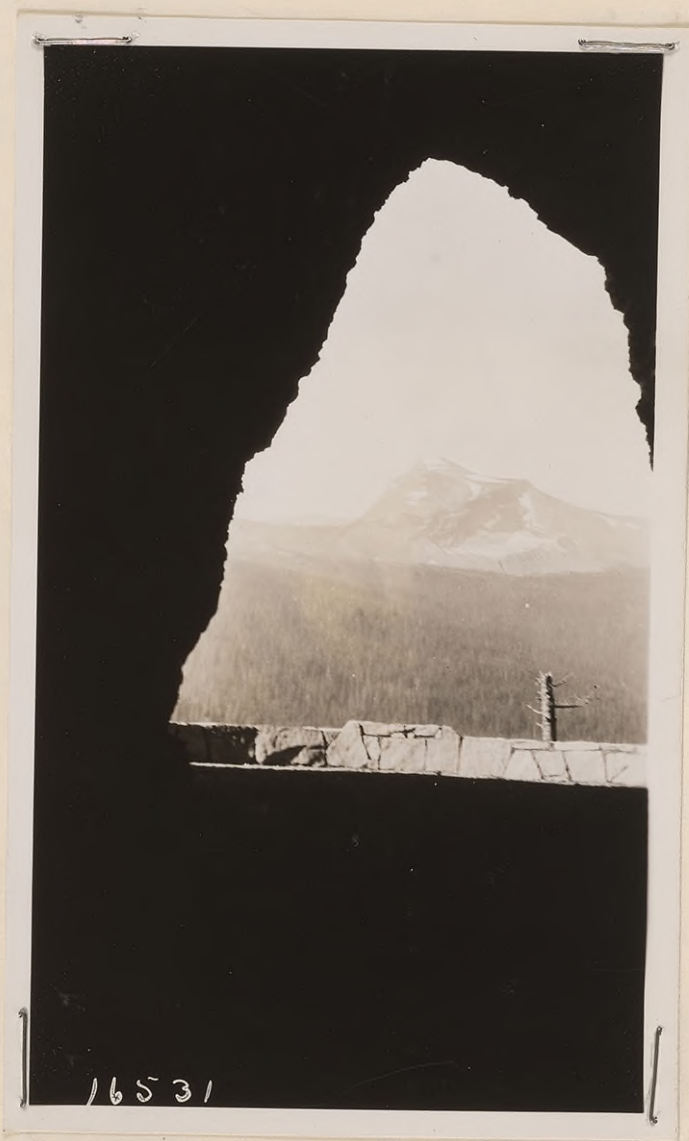
#16531 - View from window of tunnel, Sta. 643/20. Two similar windows, width about 16 ft. wide and 20 ft. high. Heaven's Peak, elevation 8994, in background. Cement rubble guard rail at cliff edge. Oct. 1928.
