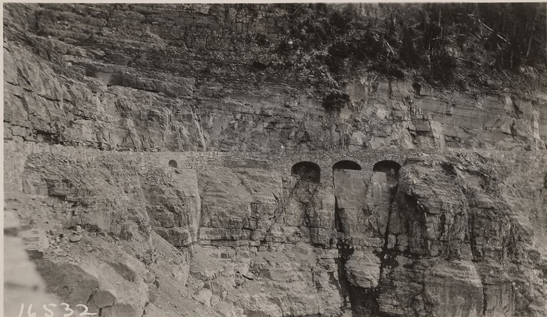
#16532 - View shows three 16' span cement rubble masonry arches at Sta. 102 constructed in order to avoid excessive structure excavation and resulting high retaining walls. Arch barrels support about half of roadway. Also shows 6' x 4' arch culvert as well as character of rock encountered and depth of cuts required. (Ladder may be used for comparison).
