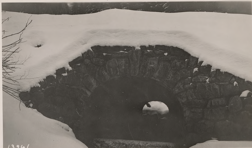
#13961 Cement rubble masonry end wall and wings on 6' x 4' concrete box culvert, sta. 499. Oct. 1926
