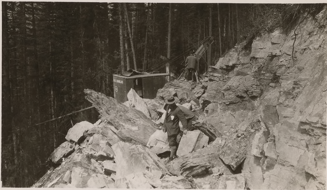
No number - Pictures from Dept. of Agriculture, Dept. of motion pictures. Showing power shovel handling rock excavation. Sta. 430 Black. July, 1926.
