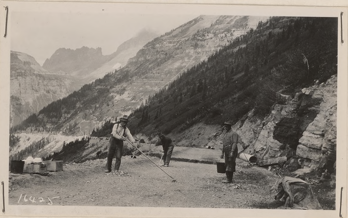
#16425 - Sta. 70. Sept., 1928. Raking subgrade to remove over-size rocks preparatory to laying of crushed rock surfacing. Note trench section to hold surfacing material.
