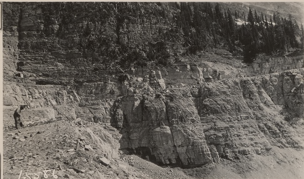
#15586 - Rough graded highway along cliffs, Stas. 100 to 110. Retaining walls, arches, and guard rails later constructed. Center of view site of three 16' span arches built to hold half roadway. Camp #5 upper right. August, 1927.
