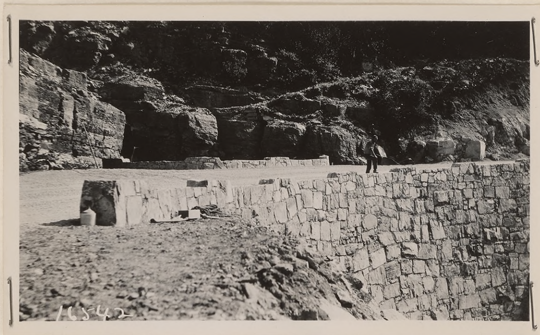
#16542 - Sta 89. Completed cement rubble masonry retaining walls and guard rails. Wall 47' maximum height. outer batter 1 to 10, inner batter 1/4 to 1, top thickness 1.65 ft. on 54° 30' curve. September, 1928.
