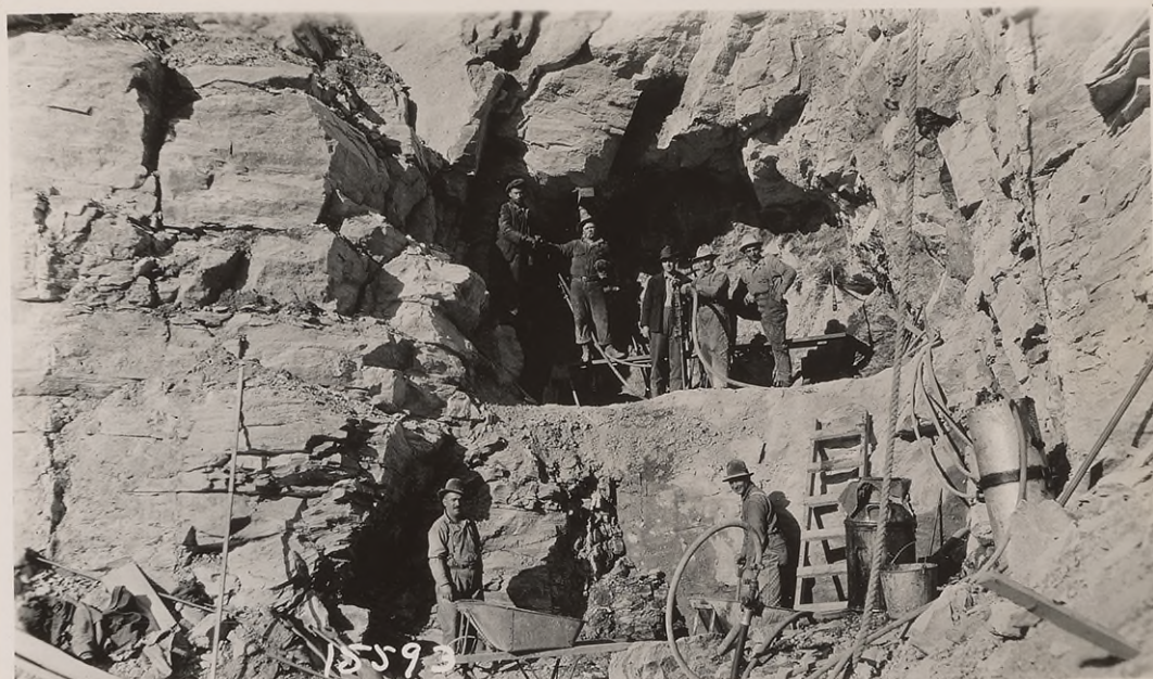
#15593. Oct. 1926. Beginning of tunnel at east portal, sta. 444, showing system of construction, character of rock, seams, etc.
