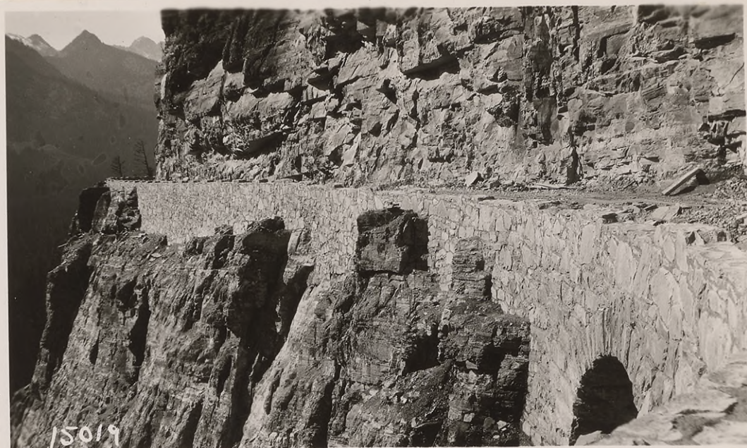
#15019 October 1927. Sta. 379 ahead showing 18' span cement rubble masonry culvert opening in wall, general type of retaining wall along cliff section, and type of guard rail to be used on entire project.
