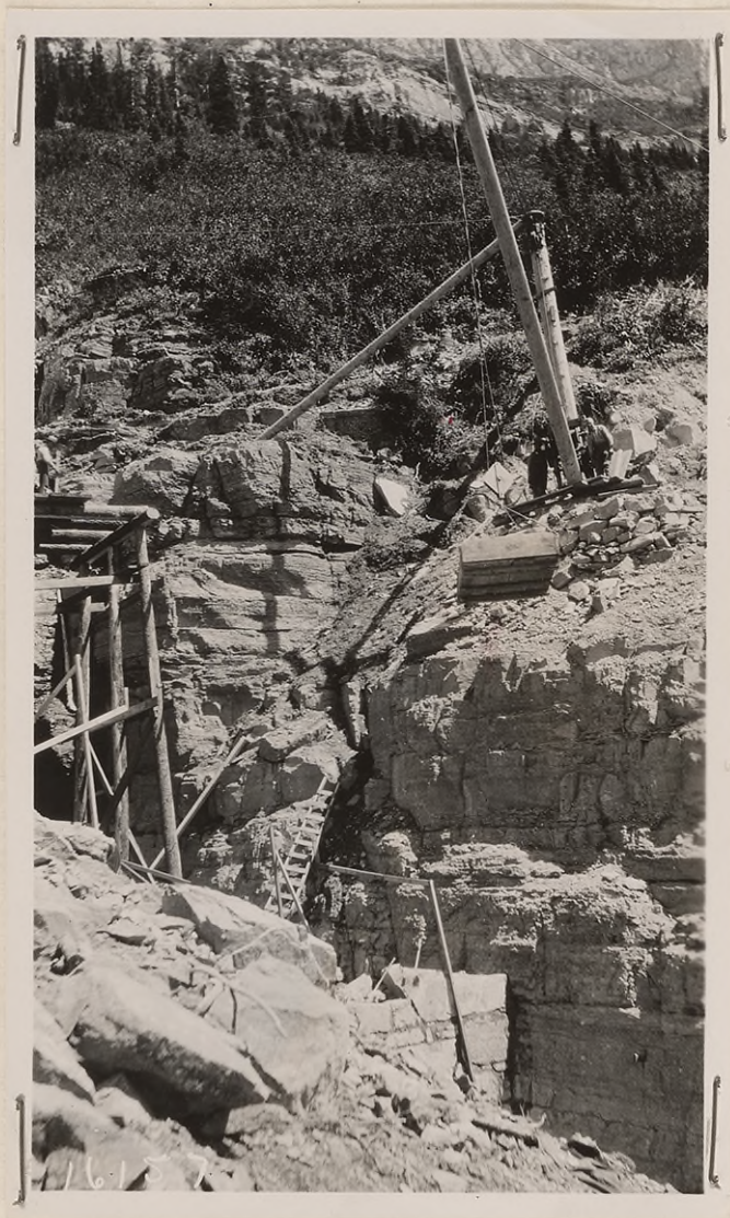
X #16157 - Showing start of cement rubble masonry retaining wall at Sta. 89, derrick or gin pole with skip for handling rocks for wall. Temporary frame trestle at side for construction purposes. Maximum height of wall 47' outer batter 1 to 10, inner batter 1 to 4, wall on 54 degree curve making arch action in wall. Note large rocks used. July 10, 1928.
