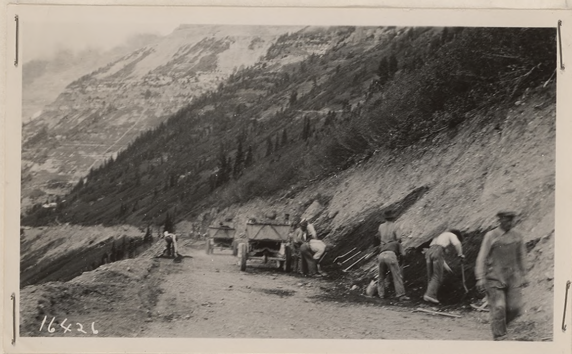
#16426 - 1-1/2 yd. Ford dump trucks hauling cushion material for rock sections along cliffs. Sta. 70 ahead. September, 1928.
