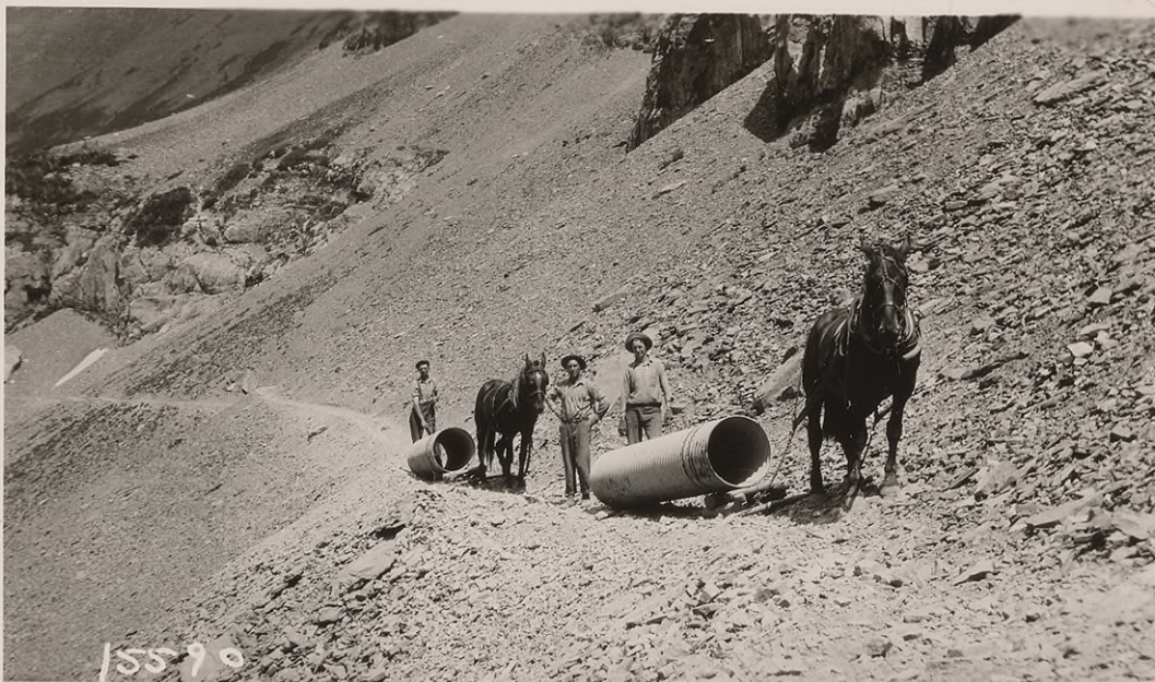
#15590. August 1926. Sta. 40 ahead on old Granite Park trail. Elevation 6450. Showing use of "go-devil" or travois for hauling culvert pipes, steel rails, air pipes, etc. over the narrow trail from camp #1, elevation 3500 to camps #5 and #6 at elevation 6600. One day for one trip.
