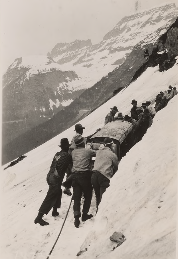
X #14724. June 22, 1927 Sta. 45 ahead. Men hauling compressor from camp #6, sta. 15 to sta. 50. Along old Garden Wall Trail.
