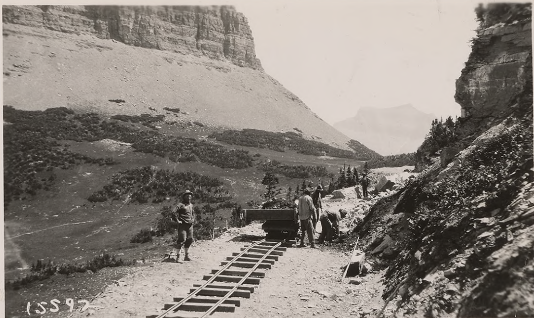
* #15592 Aug. 1926. Sta. 12 back showing car and track method of handling excavation by stationmen. "Garden Wall" and trail on left. Logan Pass in middle background.
