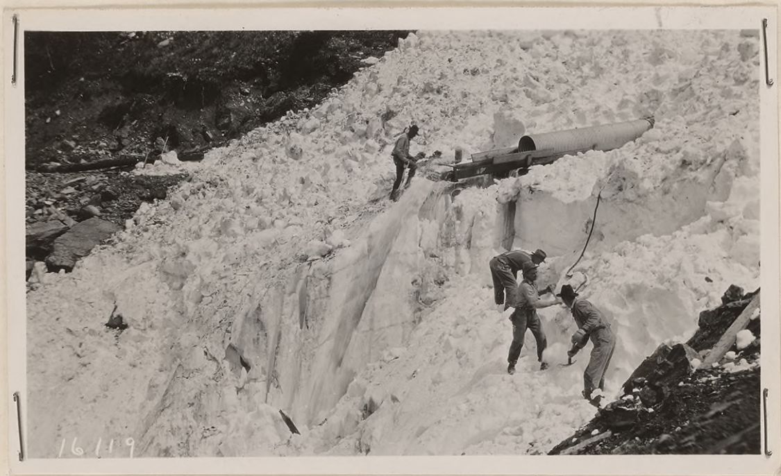
#16119 - Removing snow from deep gulch, 50 ft. deep 40 ft. wide, June 23, 1928, to begin construction of two retaining walls, sta. 89. Sluicing was attempted but found impractical. Bridge not desired on account of danger of snow slide carrying bridge away. Two walls with back filled road between thought best for conditions. June 23, 1928.
