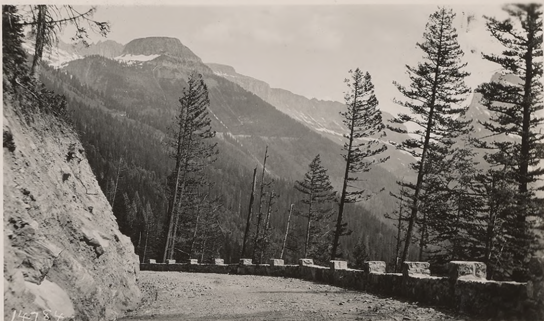
#14784 July 1927. Sta. 456 ahead. Cement rubble masonry guard rail, 1'6" high, 1'6" thick; pilasters 18" square, 10" high, spaced 13' c-c. This type discontinued in favor of type shown below. Background shows road on slope of Haystack Butte, big slide approximately at sta. 219.
