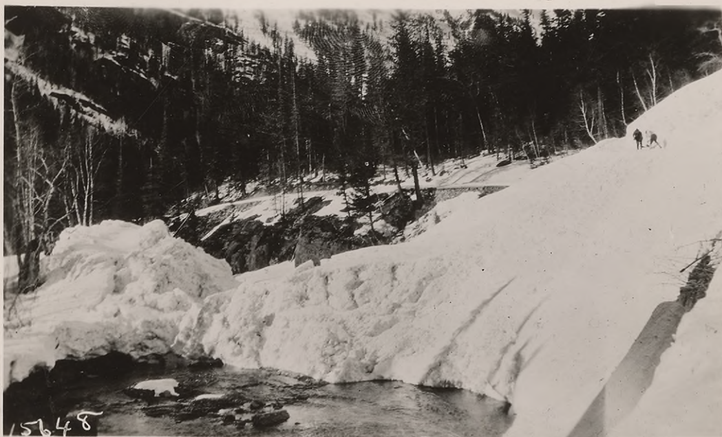
#15648. View of huge snow slide at cribbing on Mt. Cannon Section, 18.5 miles from Belton, 2\frac{1}{2} miles from beginning of #287 project, 3\frac{3}{4} miles from camp. #1 of contractors. Slide about 600' long and 20 to 50 ft. deep. April 1927.
