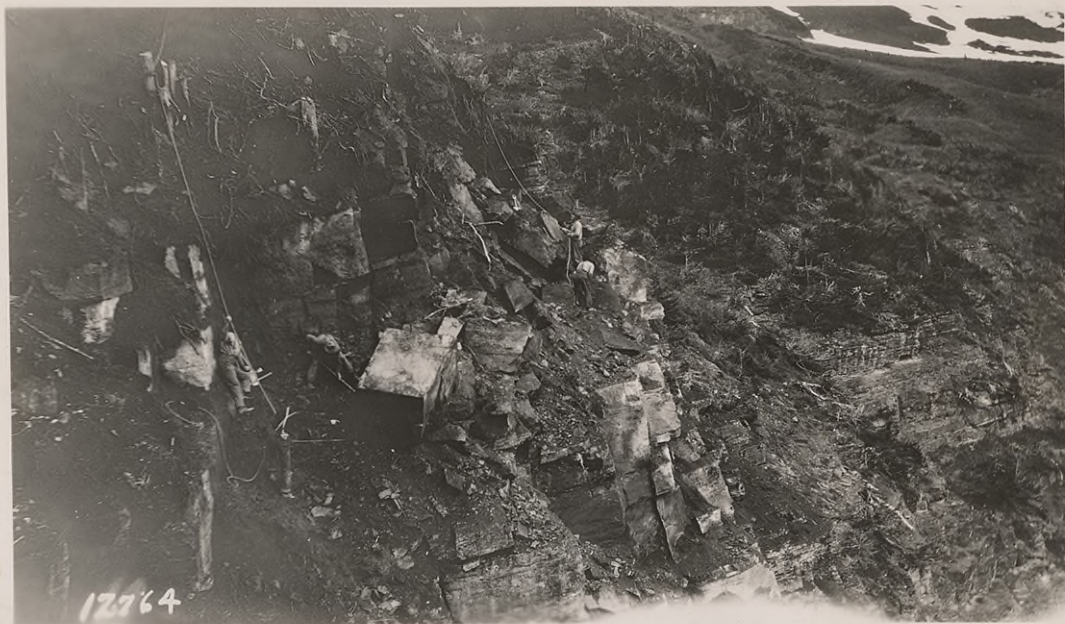
#12764. June 1926. Sta. 255 back showing stationman beginning excavation on steep rock cliff. Rock barred off in first operations. Note safety ropes used by laborers. Natural dump grounds below cliff. North gulch of Haystack Butte.
