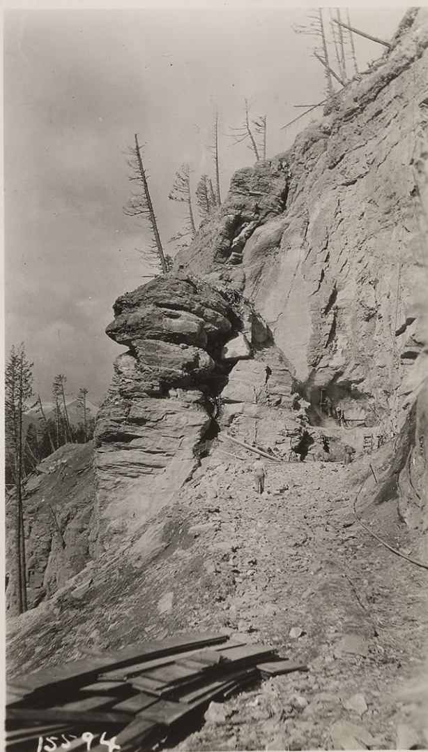
#15593. Oct. 1926. Beginning of tunnel at east portal, sta. 444, showing system of construction, character of rock, seams, etc.
