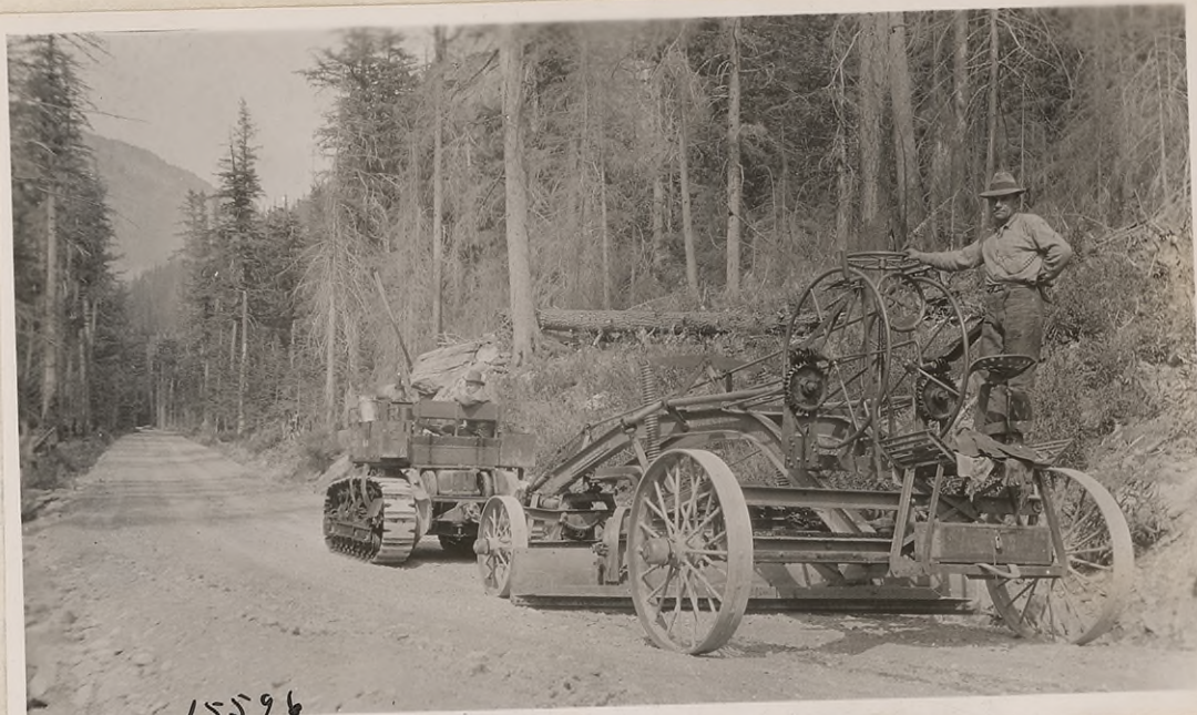
#15596 Aug. 1926 Use of tractor and blade machine in preparation of subgrade before laying of base course rock on Mt. Cannon Section, \frac{1}{2} mile above Avalanche Creek.
