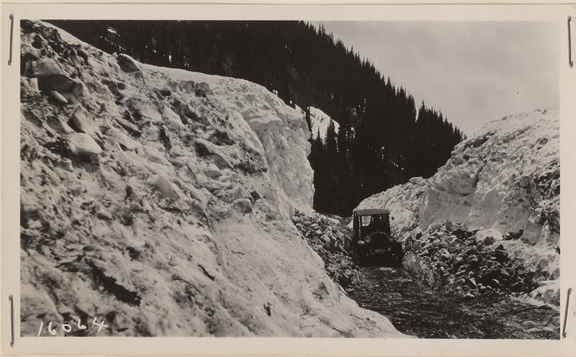
#16064 - Cut through big snow slide at Sta. 150, July, 1928. Usual slide each year 1000' wide by 10' to 35' deep. Removed by steam shovel.
