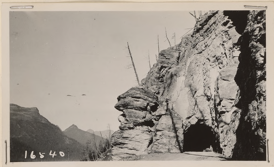
#16540 - East portal of tunnel, Sta. 444/42. Length 192 ft., width 20 ft., height 18 ft., ceiling semi-circle of 10 ft. radius. Unlined. On curved alignment, one 15^{\circ} 30' curve complete and portions of 44^{\circ} and 23^{\circ} . October, 1928.
