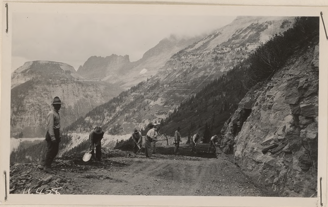
#16428 - September, 1928. Sta. 60 ahead. Fine grading preparatory to laying crushed rock surfacing. Camp #5, sta. 98 in center background. Also construction trail. Haystack Butte left. "Garden Wall", continental divide, background.
