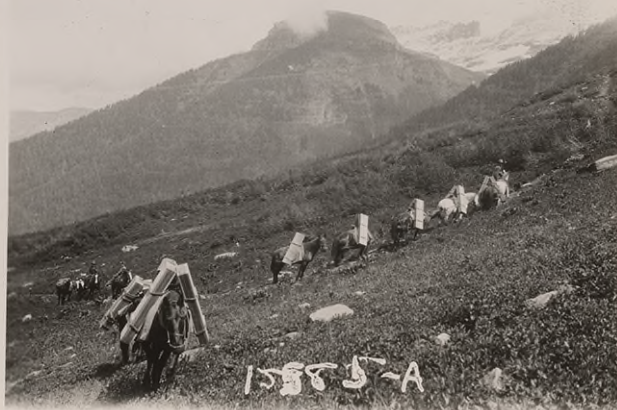
#15585-A. Aug. 1926 Showing pack horse string leaving "Jones" Flat, below Logan Pass, enroute to camp #5, sta. 96. Loads of 3/8" x 5'0" lumber for construction camp. All camp lumber for #5 and #6 hauled thus.
