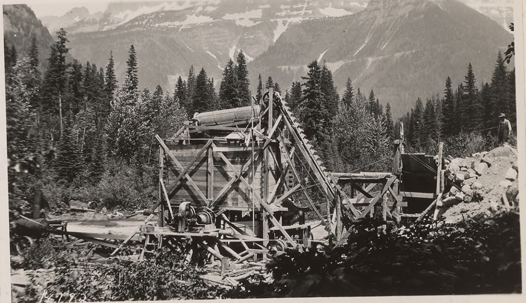
#14792 July 1927. Rock crushing plant 300 ft. left of sta. 639. #2 Aurora Jaw Crusher, 1-4½" Traylor Gyratory finishing crusher, 1-double drum belted hoist for drag line, 30" x 12' revolving screen, 1-90 HP. Russell steam tractor. Background shows road along side of Haystack Butte. Camp #4 at left center.
