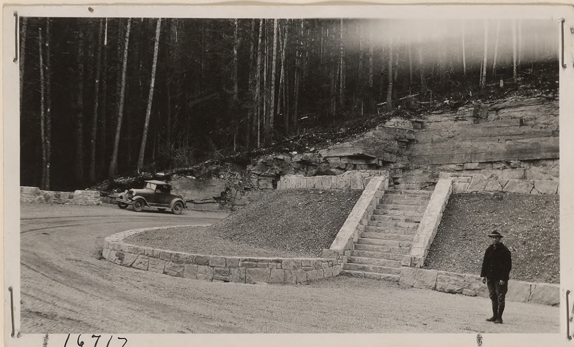
#16717 - Close up of cement rubble masonry toe wall, guard rail and steps. Inlet of 6" porous tile drain may be seen in center of toe wall left of steps. Steps, tread 12", rise 8", width 6' - 0". Oct. 18, 1928.
