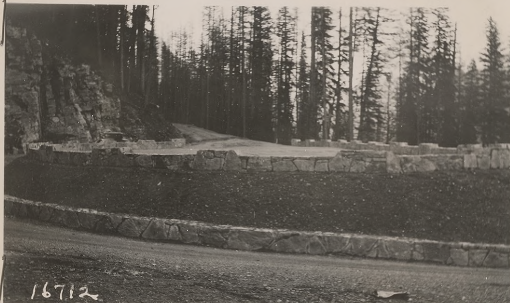
#16712 - View back from sta. 411/50 across upper parking area of "The Loop" showing cement rubble toe wall and guard rail. "The Loop" - radius 75 ft., central angle 215 degrees, widened 4 ft. and superelevated 3 ft. 3% grade. Oct. 18, 1928.
