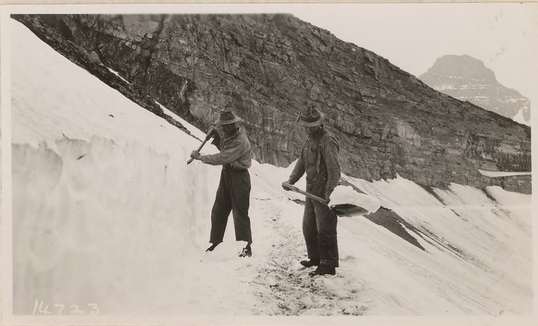
#14723. Sta. 45 back toward summit, showing hand methods of handling snow. Preparing trail to move compressor from camp #6, sta. 15 to sta. 50. Trail also used for packing to camp #6 from camp #1, sta. 575. June 22, 1927.
