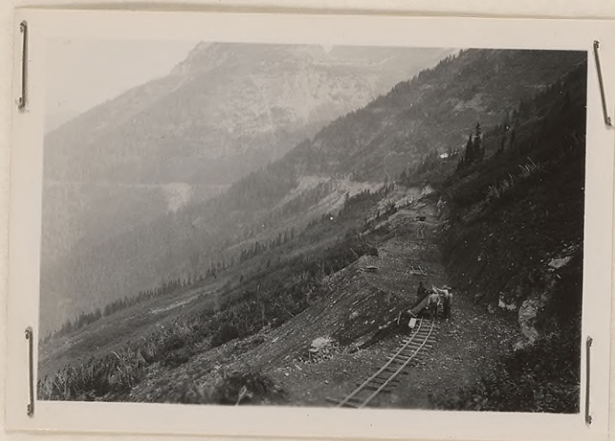
Private photos - no number. Sta. 55 ahead showing use of cars and tracks for hauling by station crew. August, 1927.
