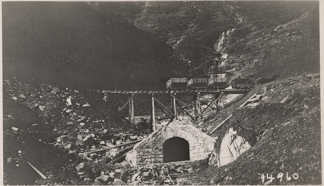
#14960. September, 1927. Showing end wall construction on cement rubble masonry culvert, 6' x 6', sta. 153. Also showing gasoline "dinky" engine and cars for hauling and making fill.
