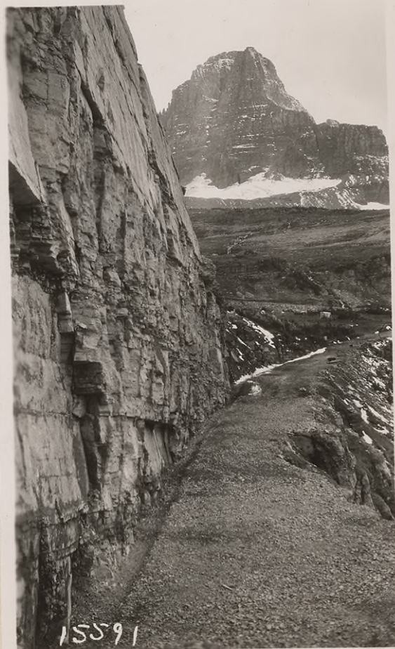
#15591. September 1926. Sta. 36 back showing fine example of rock slope in heavy work along cliff section. Slope about 1 to 20, cut being about 90°. Slope made in lifts of 8' to 10' by stationmen sub-contractors. Retaining wall needed at intervals with continuous guard rail. Mt. Clements, elev. 8764, in background, having perpetual snow and glacier.
