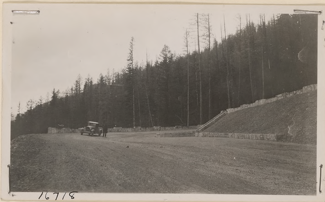
#16718 - View back from Sta. 414 showing lower parking area, 5750 sq.ft. at "The Loop". Also cement rubble toe wall, guard rail and steps leading to upper parking area. October 18, 1928.
