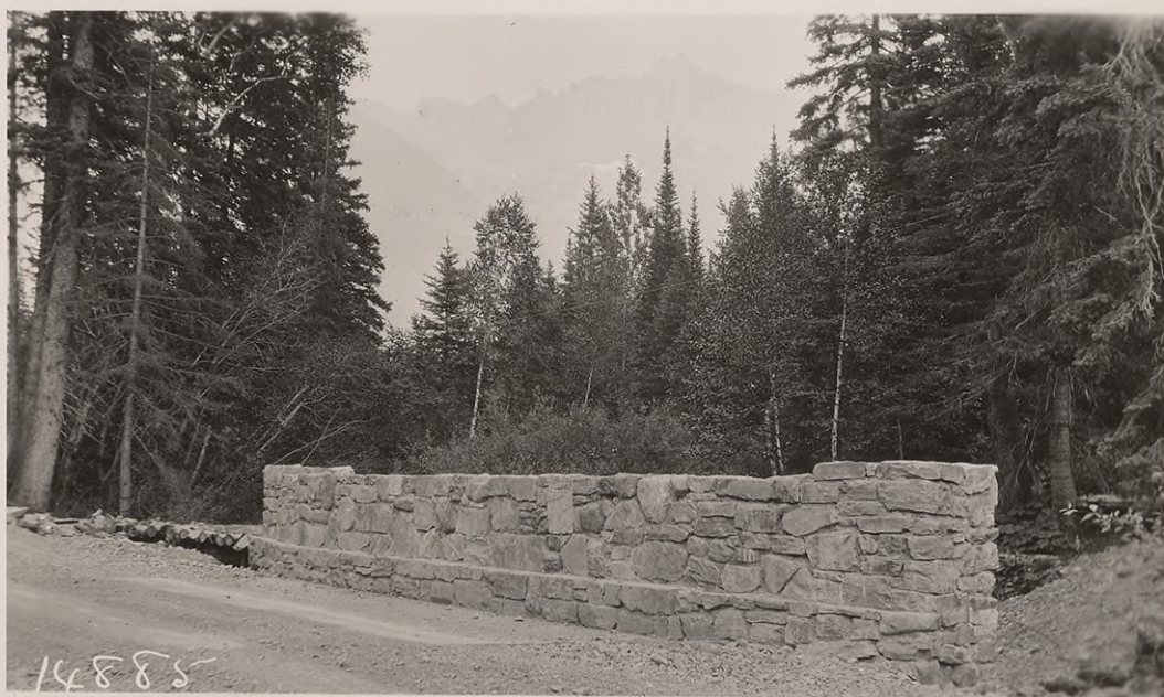
#14885 Cement rubble masonry railing on 16' span, concrete slab bridge, sta. 644. 1'6" thick, 3'3" high, 32' long. September 1927.
