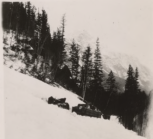
#15648. View of huge snow slide at cribbing on Mt. Cannon Section, 18.5 miles from Belton, 2\frac{1}{2} miles from beginning of #287 project, 3\frac{3}{4} miles from camp. #1 of contractors. Slide about 600' long and 20 to 50 ft. deep. April 1927.
