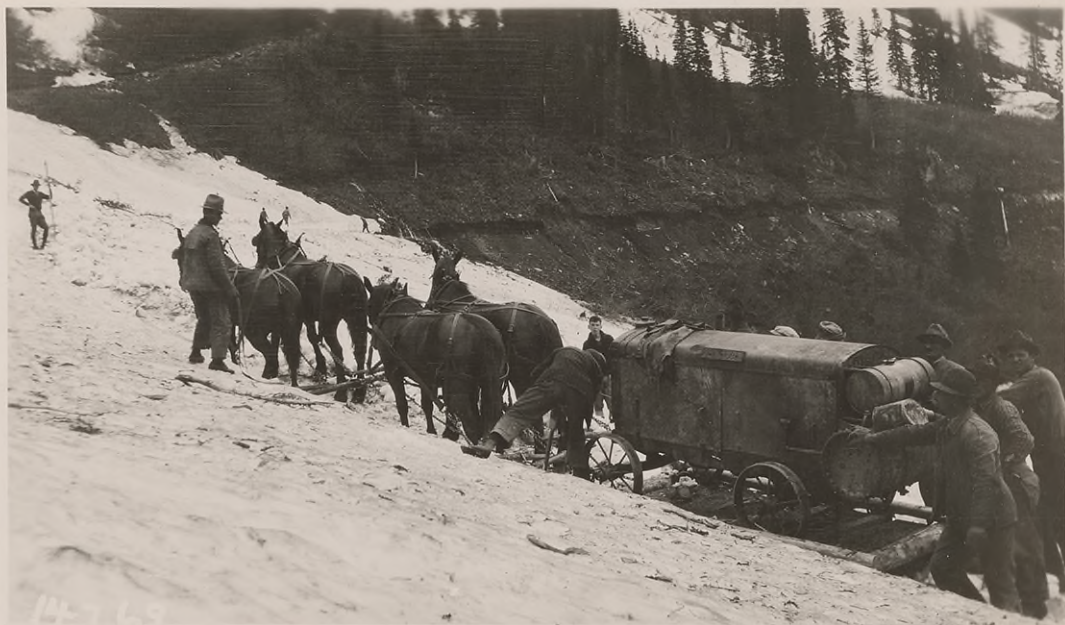
#14769 Moving compressor across snow slide, 50' deep by 1000' wide, sta. 145, south gulch Haystack Butte. July 7, 1927 View toward summit.
