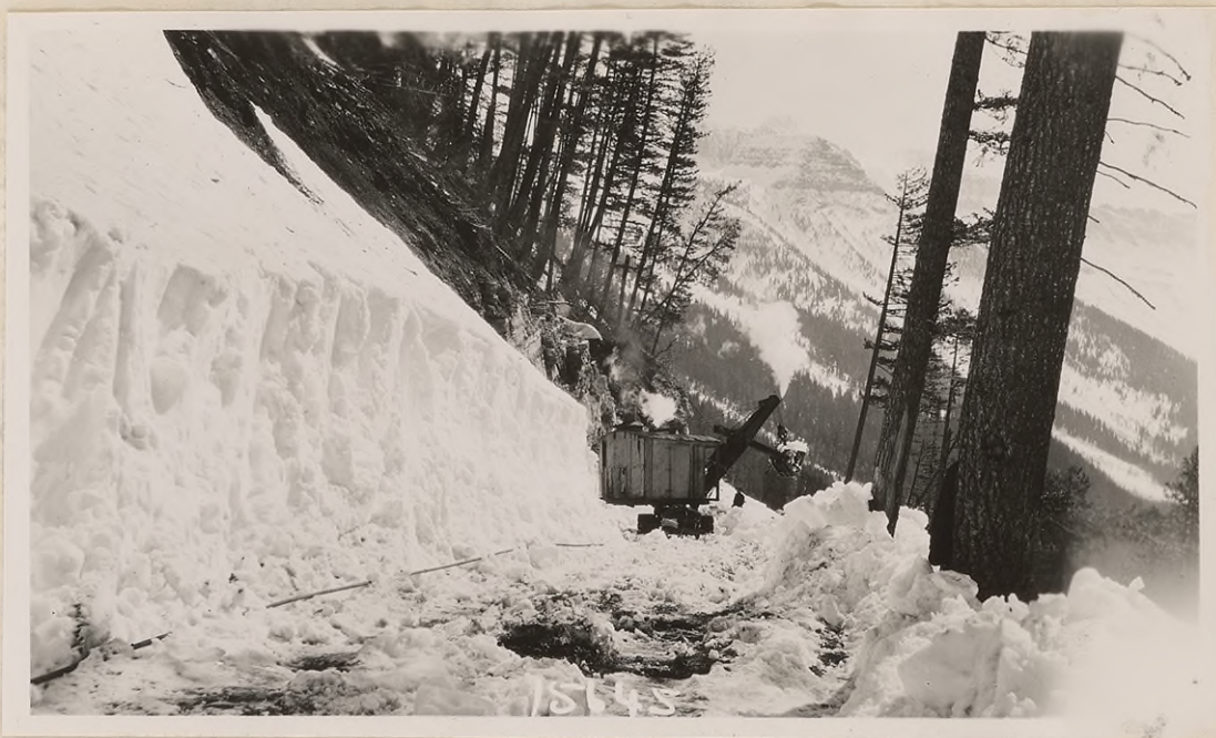
#15645. Sta. 435 ahead. Steam shovel working its way through snow toward tunnel. April 10, 1927. Much shovelling of snow necessary across slides.
