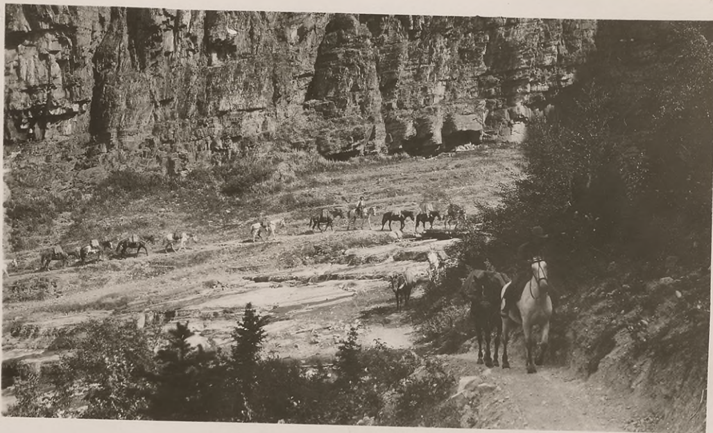
# July 1926. ( Dept. of Agri. Moving Picture Div. film.) Showing pack string at site of high falls on Logan Pass trail. Enroute to camps # 5 and #6 from camp #1 with dynamite, black powder, supplies, etc. Load of each horse from 150# to 200#. One day required for trip a distance of about five miles, one way, and climb of 3,000. ft. in elevation. Sixty horses used at peak of work. One man needed for each every eight to ten horses.
