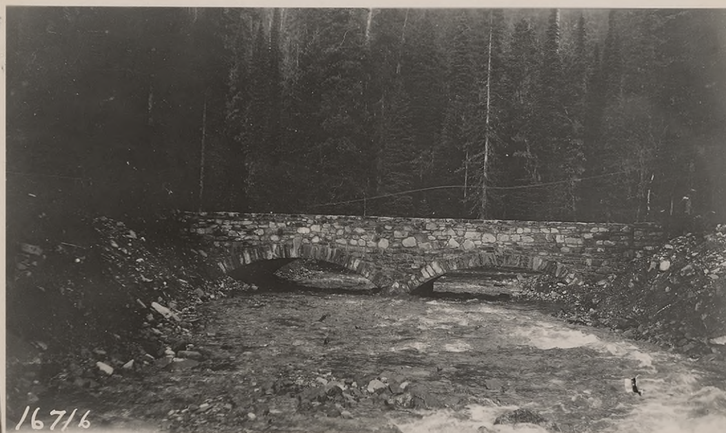
#16716 - Trapper Creek bridge, Sta. 588. Two 16' span cement rubble masonry false arches and rails combined with reinforced concrete slabs. Channel straightened and widened. Oct. 1928.
