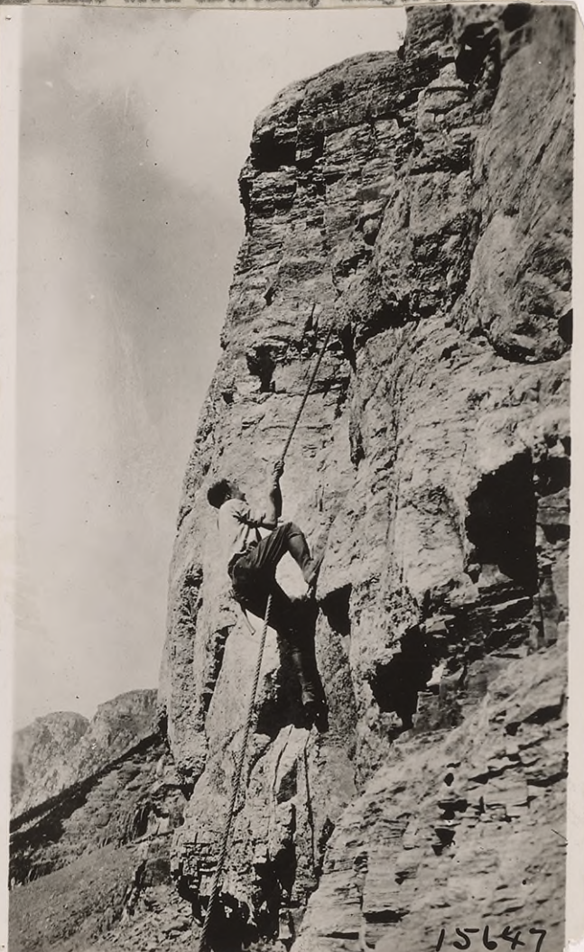
# ( Dept. of Motion Pictures, Dept. of Agri., film ) July, 1926. View showing cross-section party of engineers at work on difficult cliff sections, stas. 35 to 45. Note safety ropes. Steepness of cliffs and loose rocks made work extremely dangerous.
