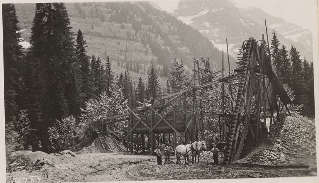
#14789 July 1927. Sand washing plant at sta. 628, 200' right of road. Rock crushing plant later transferred to this site. First oversize removed; next small gravel; last sand settling bins. Capacity about 20 - 25 C.Y. per day. Sand made and delivered to masons on project at $3.00 per C.Y.
