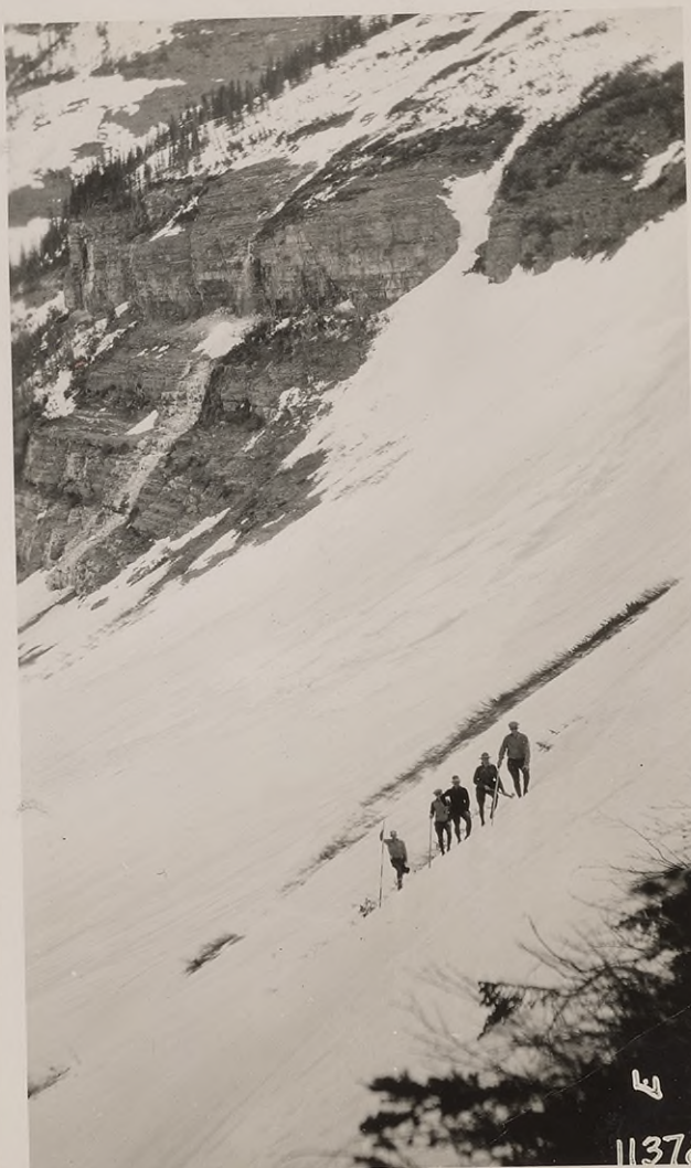
#11378 - Making ascent to Jones Flat on inspect- ion trip of May 8, 1925. Use of axe and shovel necessary to cut steps in frozen crust of snow in order to climb steep slopes Route of road above cliffs in upper part of view.
