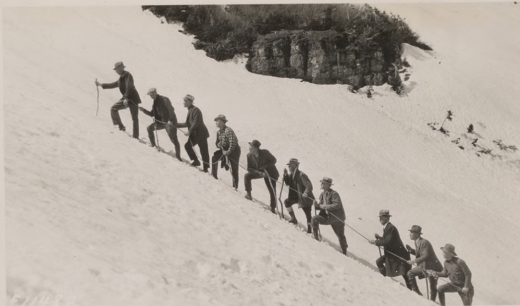
#11482 - Contractors above Jones Flat, half mile from summit. June 3, 1925.
