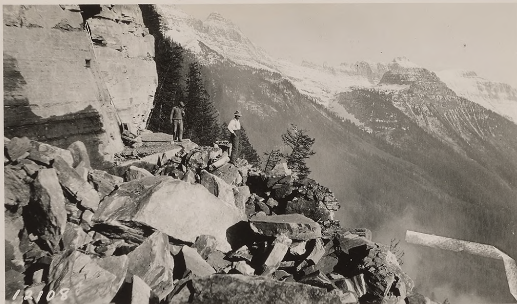
#P-5 (above) Sta. 383 back showing way rock breaks after shooting. Garden Wall in background and Haystack Butte at right. Route of road passes around to right of latter. Man on left near center line and 17 ft. above grade. October, 1925. 12108.
