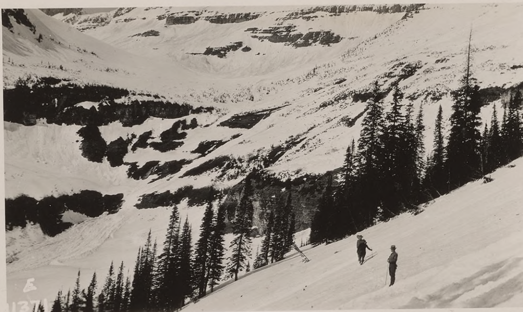
#11371 - View ahead from Sta. 135, West Side Project, into east fork of Haystack Butte Creek. Taken on inspection trip of May 8, 1925.
