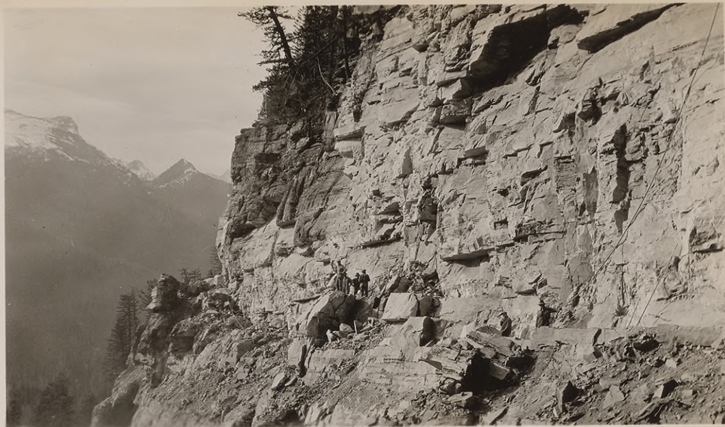
#P-20 General view of cliff work Stas. 379 to 382 (379 ahead) Note air line running up cliff, then ahead to compressors. Half tunnel effect to be attempted here. Point shows same spot as in view #11989 before shooting. October 17, 1925. 12117.
