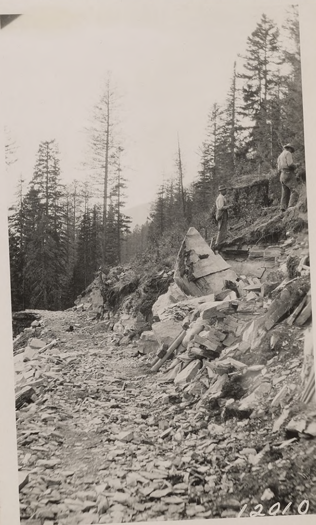
#12010 (right) Trail road built by contractor along grade line of highway to haul compressors to site of heavy cliff work. Sta. 392 ahead. July, 1925.
