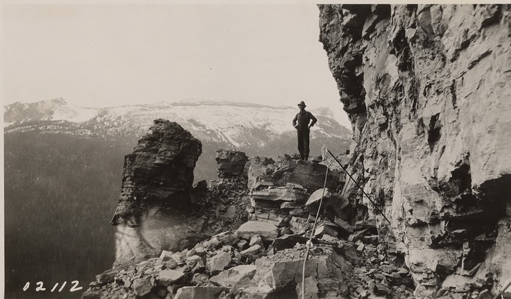
#P-15 shows undercut or half tunnel effect being accomplished. Drill with handkerchief attached shows direction of drill hole for plug-shot in undercutting. Closeup of #P-20. 12112.
