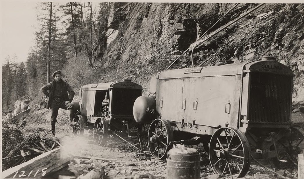
#P-21 (above) Sullivan Compressors used to furnish air for Denver Jackhammers, one drill to each compressor Sta. 388 ahead. October, 1925. 12118.
