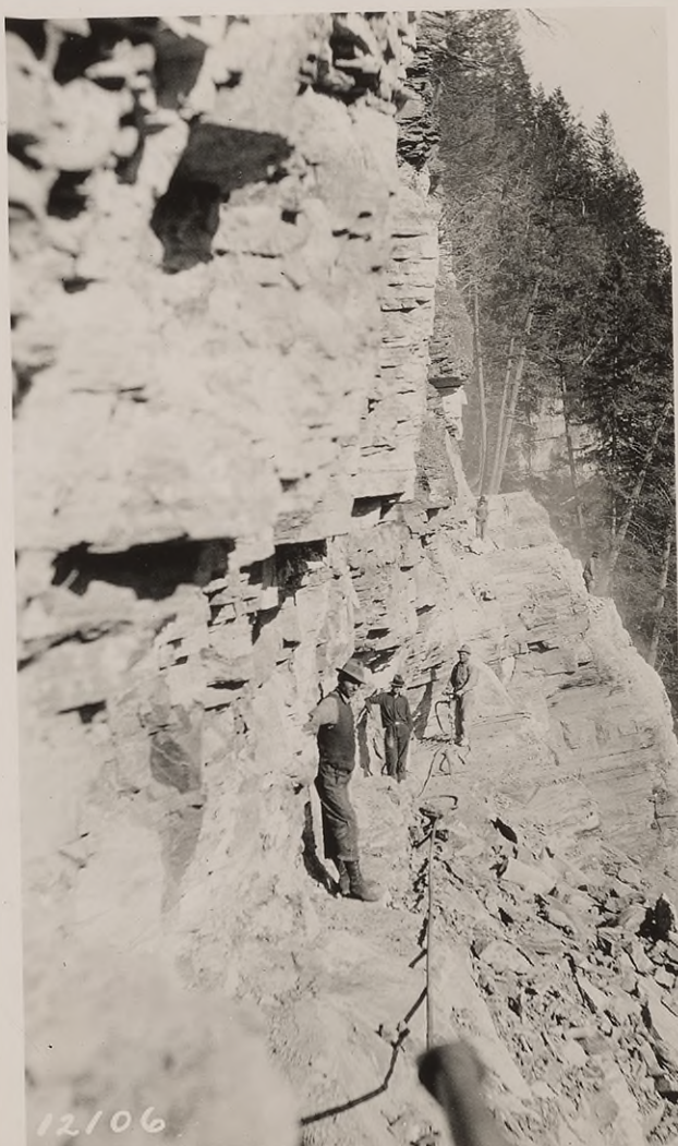
#P-5 (above) Sta. 383 back showing way rock breaks after shooting. Garden Wall in background and Haystack Butte at right. Route of road passes around to right of latter. Man on left near center line and 17 ft. above grade. October, 1925. 12108.
