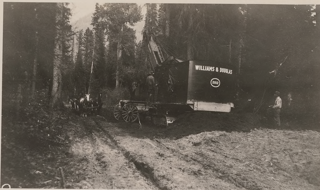
#P-9 (above) 3/4 yd. Osgood Gasoline Power Shovel excavating. Sta. 618 back, dump wagons hauling. August, 1925. Light work. 12330.
