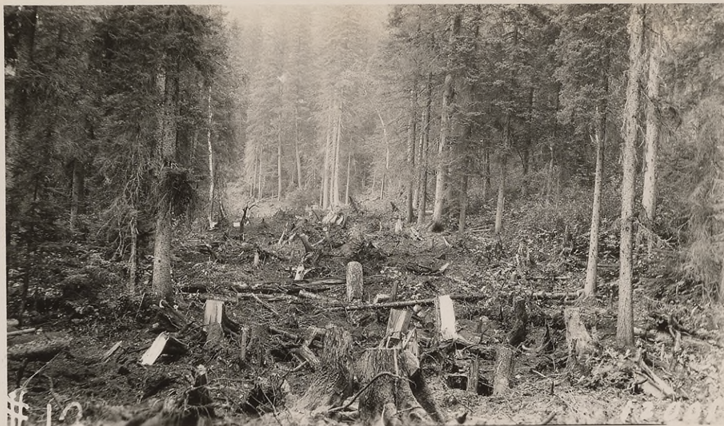
#12001 - Sta. 556 ahead, showing type of clearing, and stumps blown ready for grubbing and burning. July, 1925.
