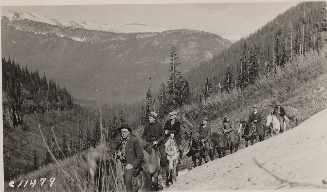
#11479 - Contractors enroute to Logan Pass to look over upper portion of West Side Project. Nearing snow fields and the end of horse back travel. Note brushed out line of previous survey by National Park Service on left side hill. McDonald Creek Valley in center. June 3, 1925.
