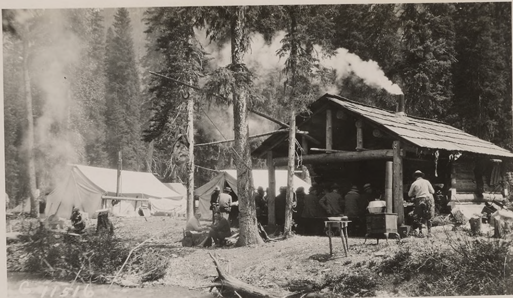
#11516 - Prospective bidders being provided for at Trapper Creek Camp, June 2, 1925.
